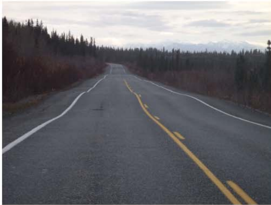
Thawing permafrost causing embankment damage. Tok Highway, MP 42.
