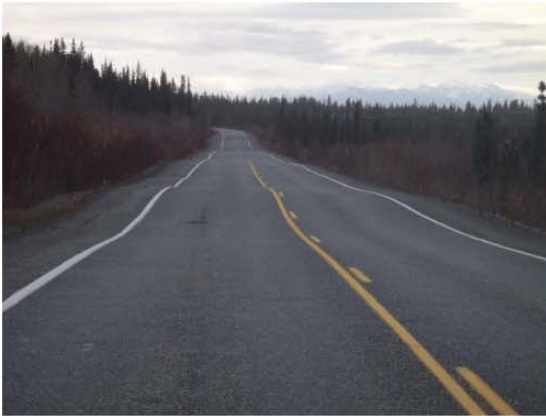
Thawing permafrost causing embankment damage. Tok Highway, MP 42.
