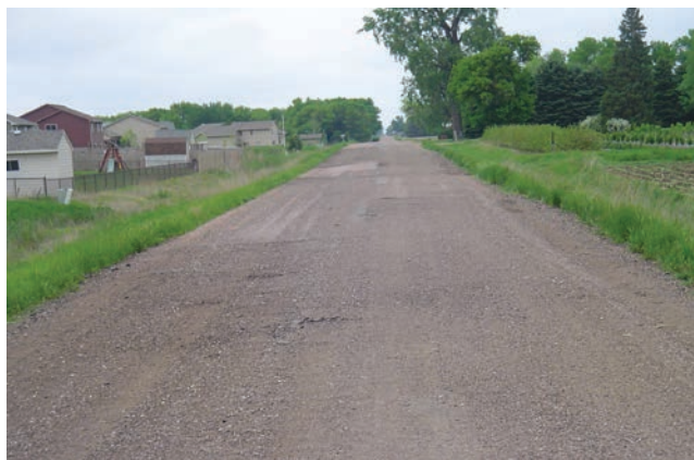
FIGURE 7 A township road failing because it carries heavy loads for which it was not designed. (Photo courtesy of K. Skorseth.)
