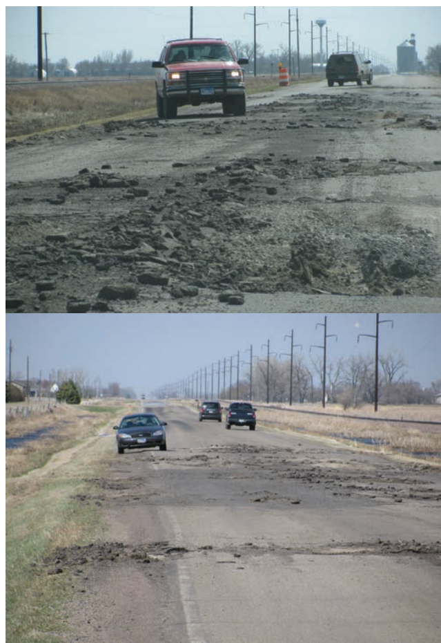
FIGURE 8 Examples of road safety effects caused by failing asphalt roads. The failures force traffic to travel outside of the lane and disrupt traffic movement. (Photos courtesy of K. Skorseth.)
