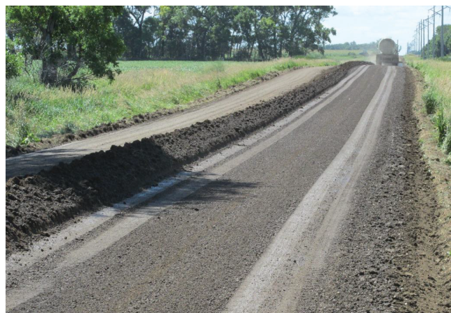
FIGURE 5 Active conversion of a failing pavement by adding new gravel and recycling. (Photo courtesy of K. Skorseth.)
