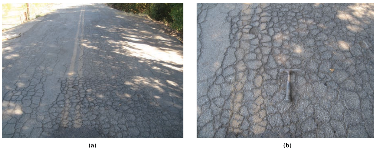
FIGURE 1 A failing asphalt road (a), and a close-up showing breakup of the pavement surface (b). (Photos courtesy of D. Jones.)
