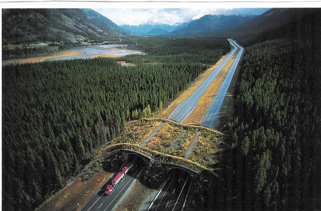
Photo 2. One of two overpasses along the Trans-Canada Highway in Banff National Park constructed to maintain wildlife connectivity.
