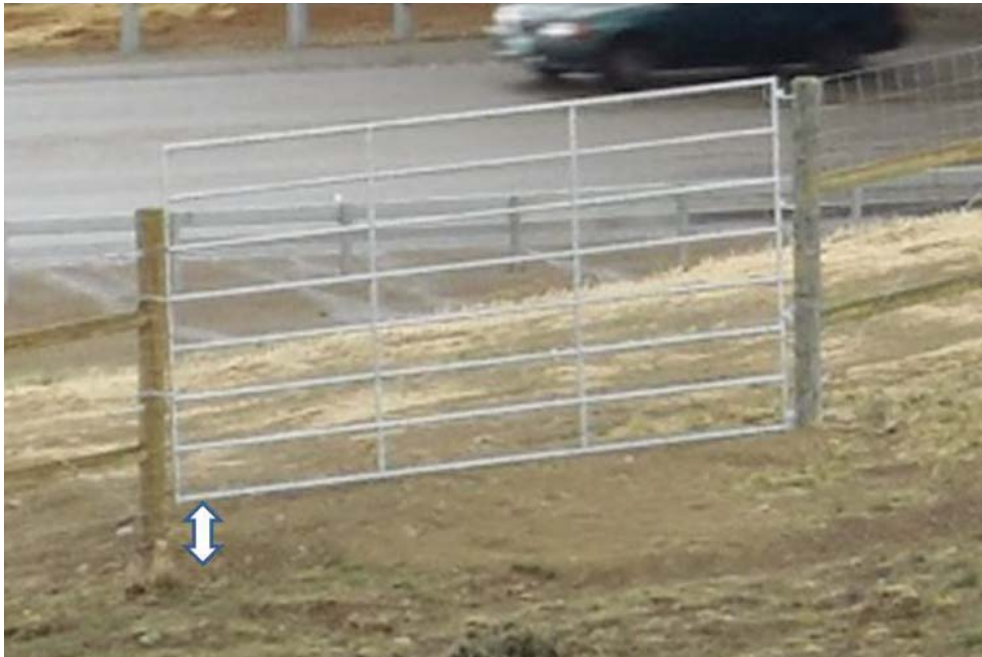
Figure 59: Example of how not specifying gate installation details could lead to large gaps in fence gate. (source: Pat McGowen).
