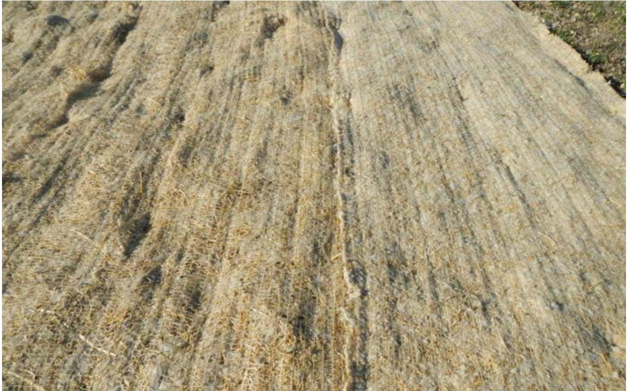
Figure 8: Photo of demonstration site where two different wool:straw ratio erosion control blankets produced by Ramy Turf Products are staked next to each other on a slope being reclaimed after recent construction along Interstate Highway 90 near Belgrade, Montana.
