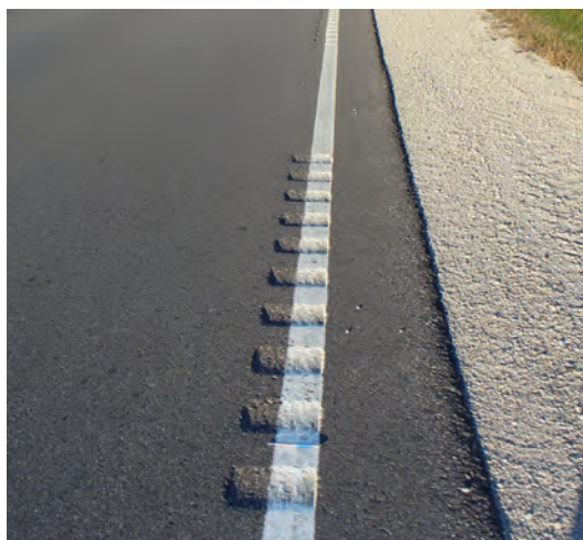
Figure 2: Edge-line rumble stripe with bike gaps (Photo courtesy of the FHWA)
