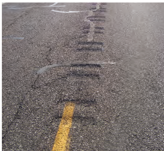
Figure 3: Centerline rumble stripe (Photo courtesy of the FHWA)
