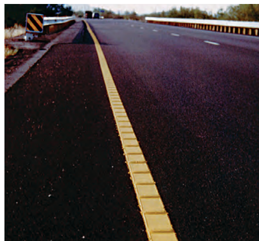
Figure 5: Profiled marking (Photo courtesy of Seth Chalmers, Pima County, Arizona)
