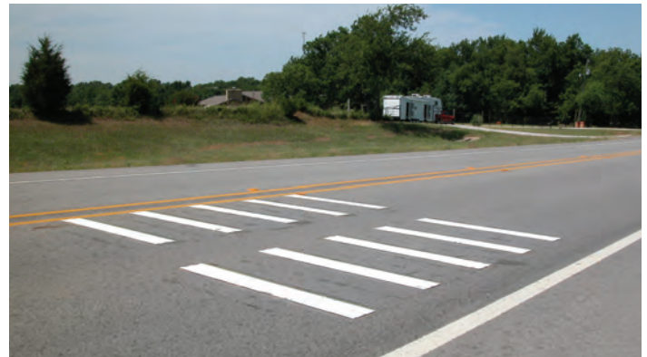
Figure 6: Transverse rumble strip marking (Photo courtesy of Texas A&M Transportation Institute)
