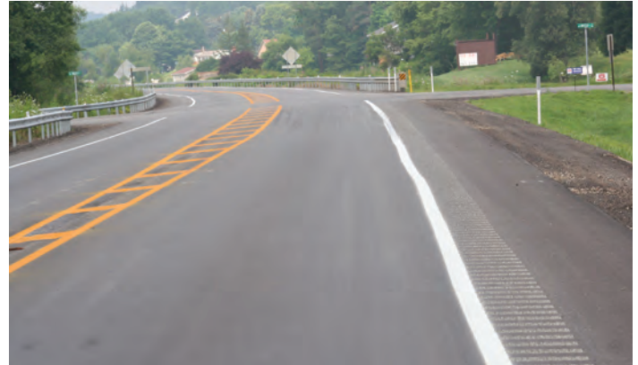
Figure 19: Lane narrowing via painted median (Photo courtesy of the FHWA – Turner-Fairbank Highway Research Center)
