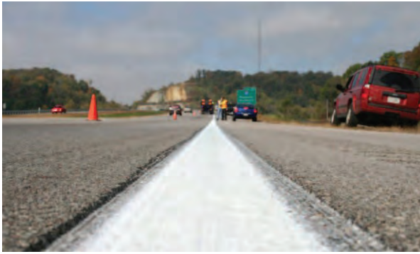
Figure 1. Pavement marking line in a grooved strip (Photo courtesy of Neal Hawkins, Center for Transportation Research and Education, Iowa State University)
