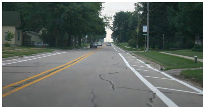
Figure 18: Lane narrowing via shoulder widening (Photo courtesy of the Center for Transportation Research and Education at Iowa State University)
