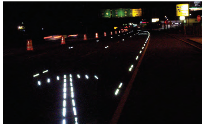
Figure 22: Lighted RPMs for a merge area (Photo courtesy of Nick Hutchins, HIL-Tech Ltd.)
