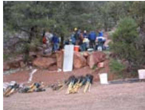
Figure 2: Volunteer Trail Maintenance Work Parties (Photo courtesy of Davis Farrar, Red Hill Council)
