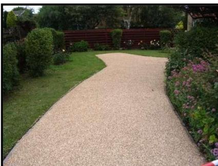
Resin bonded aggregates on a stable base in garden setting.
