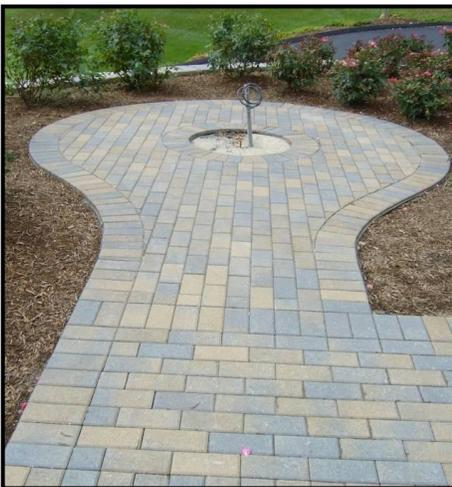
Interlocking unit pavers can be installed with mechanical laying machines to reduce cost, but this material remains at the high end of pavement costs
