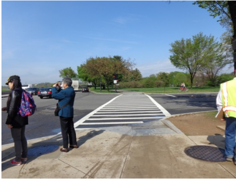
Figure 14: Curb ramp, narrower than crosswalk
