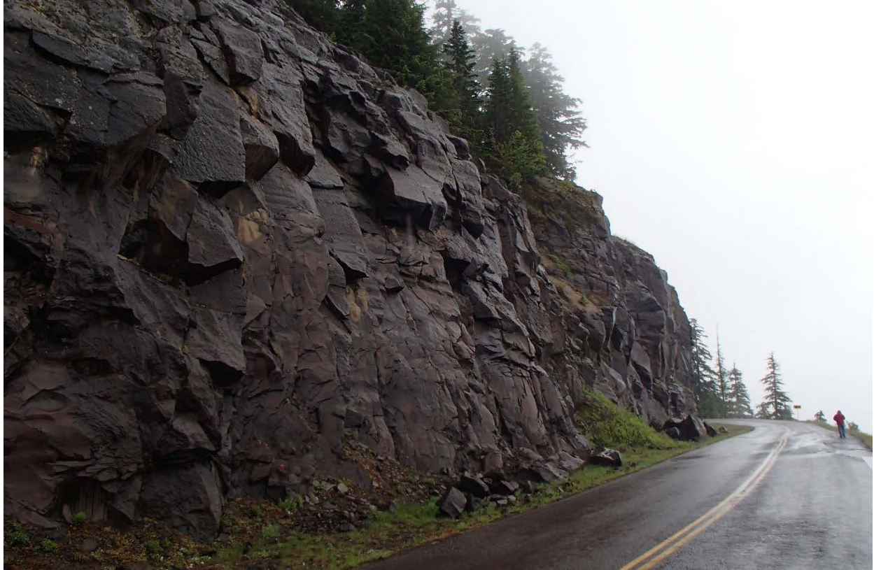
Figure 10. Rockfall debris in the roadside ditch can be used to help assess both block size/event volume and failure type. Forest Service Rd 25, Milepost 25.
