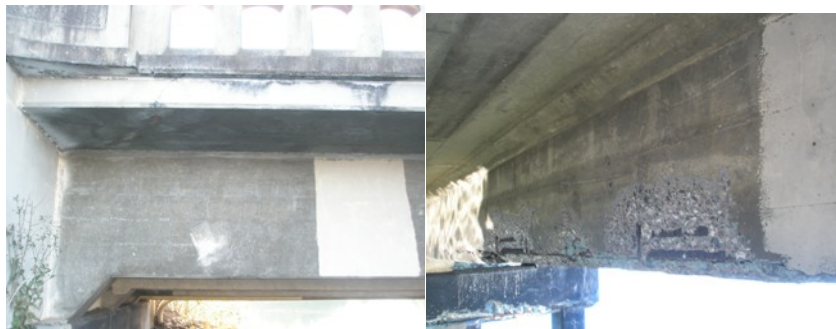
Figure 1. Two photos of the same reinforced concrete girder showing no concrete damage on the ocean-facing side (left) and corrosion damage on the face of the beam opposite the ocean (right).
