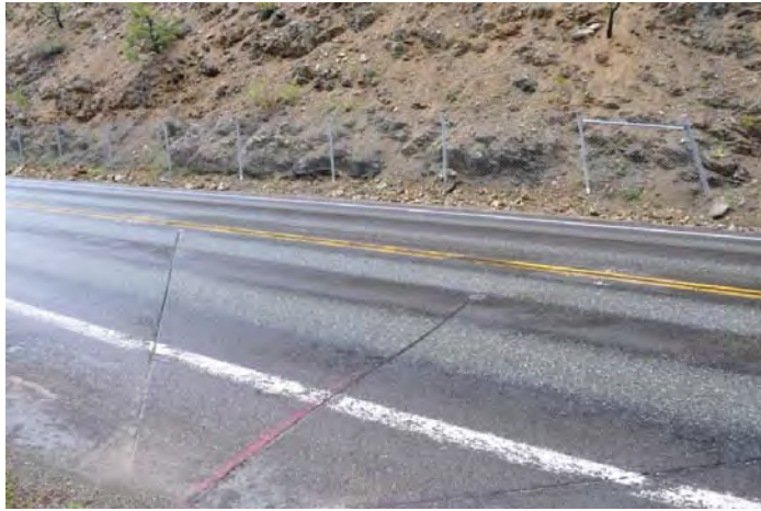
Figure 8: Pavement Surface Sensors
