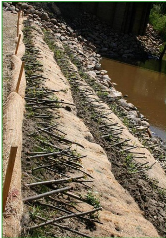
FIGURE 24 BRUSH LAYERING WITH LIVE STAKES. PHOTO PROVIDED BY G. KELLER.
