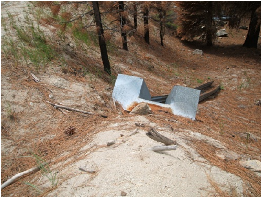
FIGURE 7 DOWN DRAIN. PHOTO PROVIDED BY G. KELLER.
