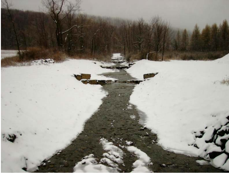
FIGURE 20 STONE CHECK DAMS. PHOTO PROVIDED BY D. ORR.
