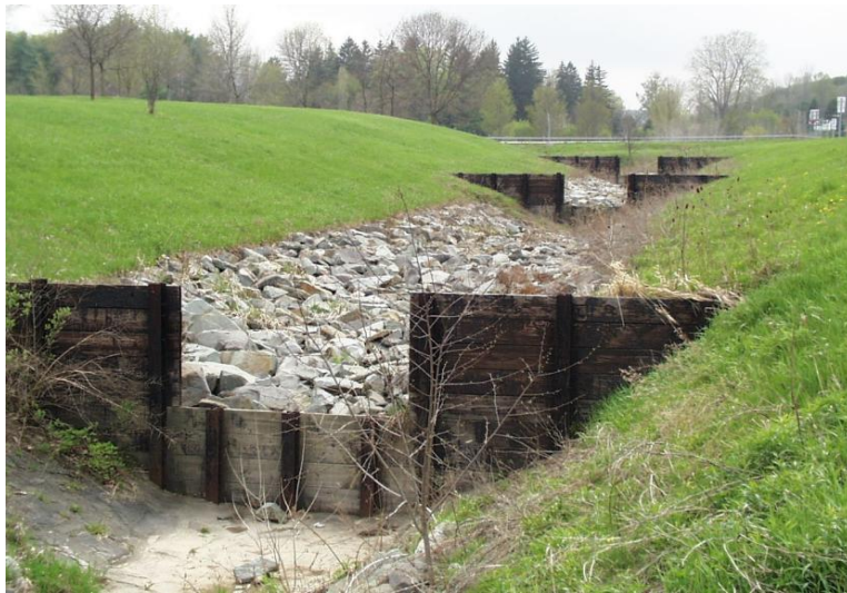
FIGURE 19 WOODEN CHECK DAMS WITH ROCK REINFORCEMENT. PHOTO PROVIDED BY D. ORR.
