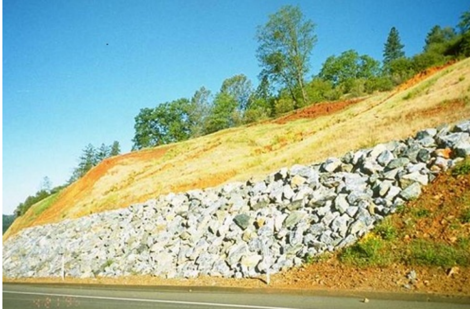
FIGURE 18 RIPRAP, OR ROCK BLANKET. PHOTO PROVIDED BY G. KELLER.
