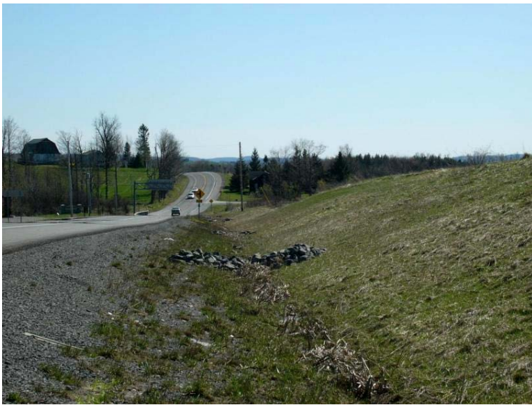
FIGURE 21 ROCK PILE CHECK DAM. PHOTO PROVIDED BY D. ORR.
