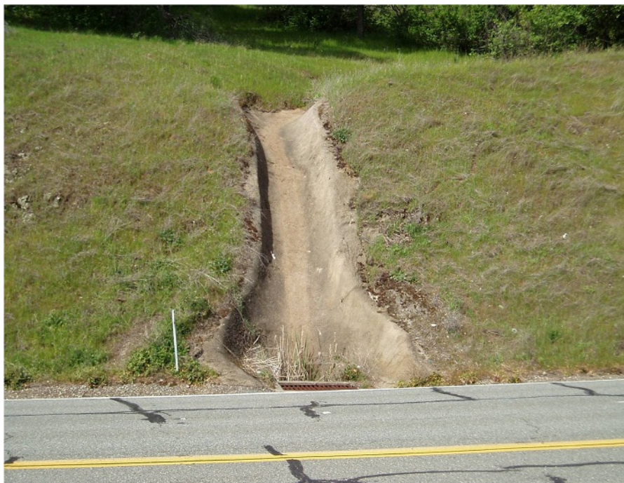
FIGURE 8 CONCRETE SURFACE DRAINAGE. PHOTO PROVIDED BY G. KELLER.
