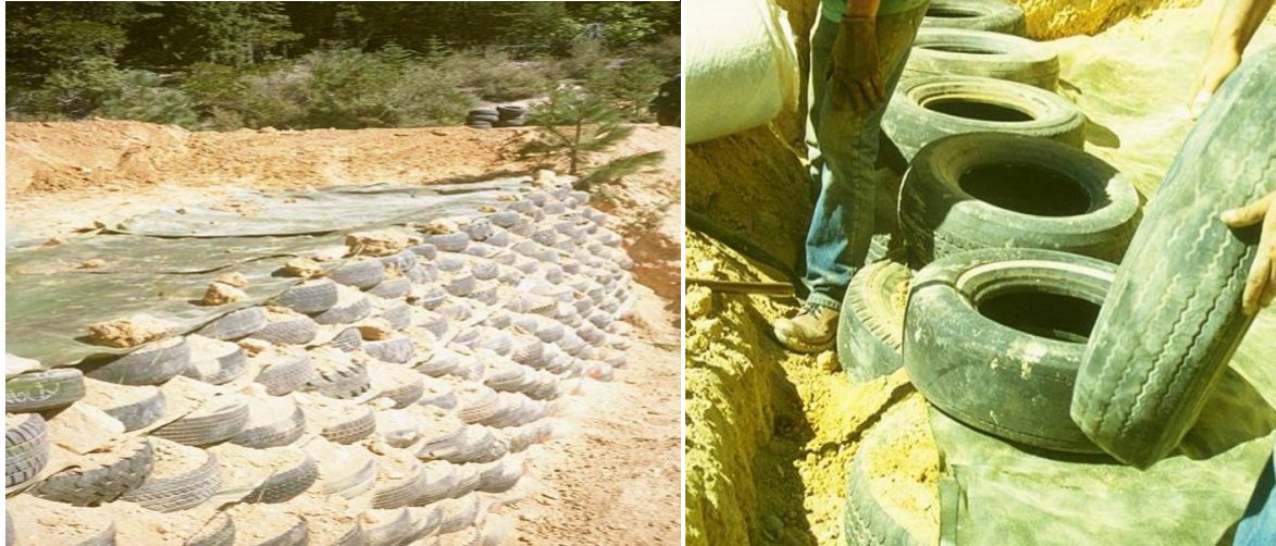
FIGURE 38 TIRE WALL AND CONSTRUCTION. PHOTOS PROVIDED BY G. KELLER.
