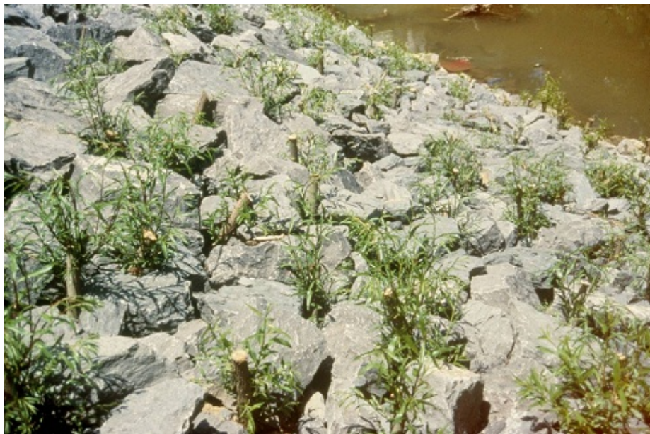
FIGURE 26 ROCK JOINT PLANTING. PHOTO PROVIDED BY G. KELLER.
