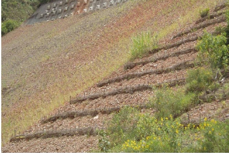
FIGURE 23 LIVE FASCINES. PHOTO PROVIDED BY G. KELLER.
