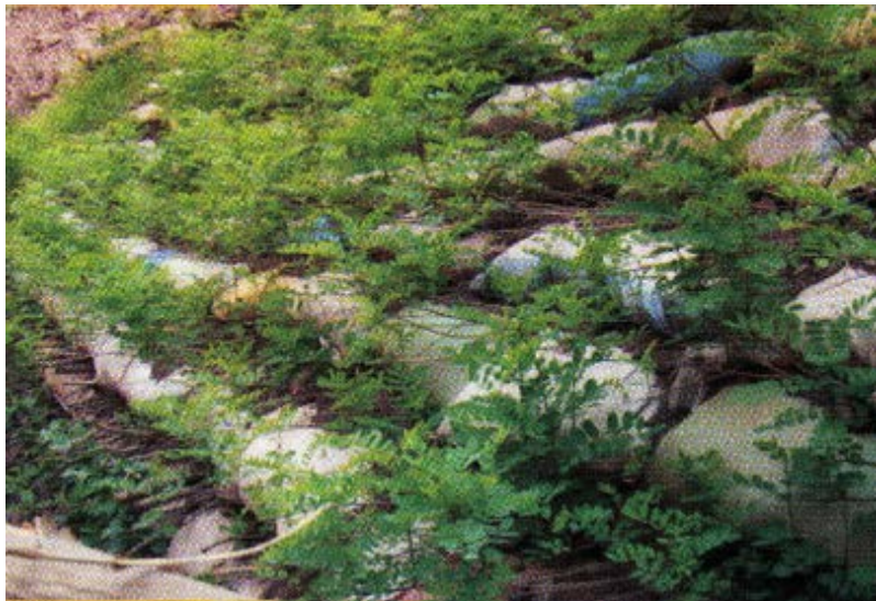
FIGURE 30 PHOTOGRAPH OF A VEGETATED SOFT GABION WALL. TAKEN FROM (SHAH, 2008).
