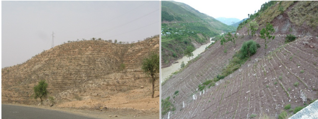
FIGURE 41 CONSTRUCTED TERRACES ON EXPOSED SLOPES IN ERITREA AND PAKISTAN. PHOTOS PROVIDED BY A. FAIZ.
