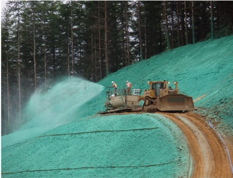
FIGURE 15 HYDRO SEEDING OF A SLOPE. PHOTO PROVIDED BY M. LONG.
