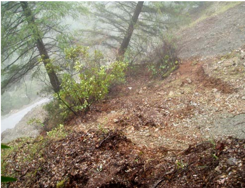
FIGURE 5 SLUMPED SLOPE WITH LEANING TREES. PHOTO PROVIDED BY G. KELLER.
