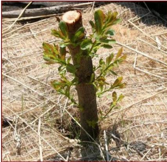
FIGURE 22 LIVE STAKE USED TO PIN DOWN MATTING. PHOTO PROVIDED BY G. KELLER.
