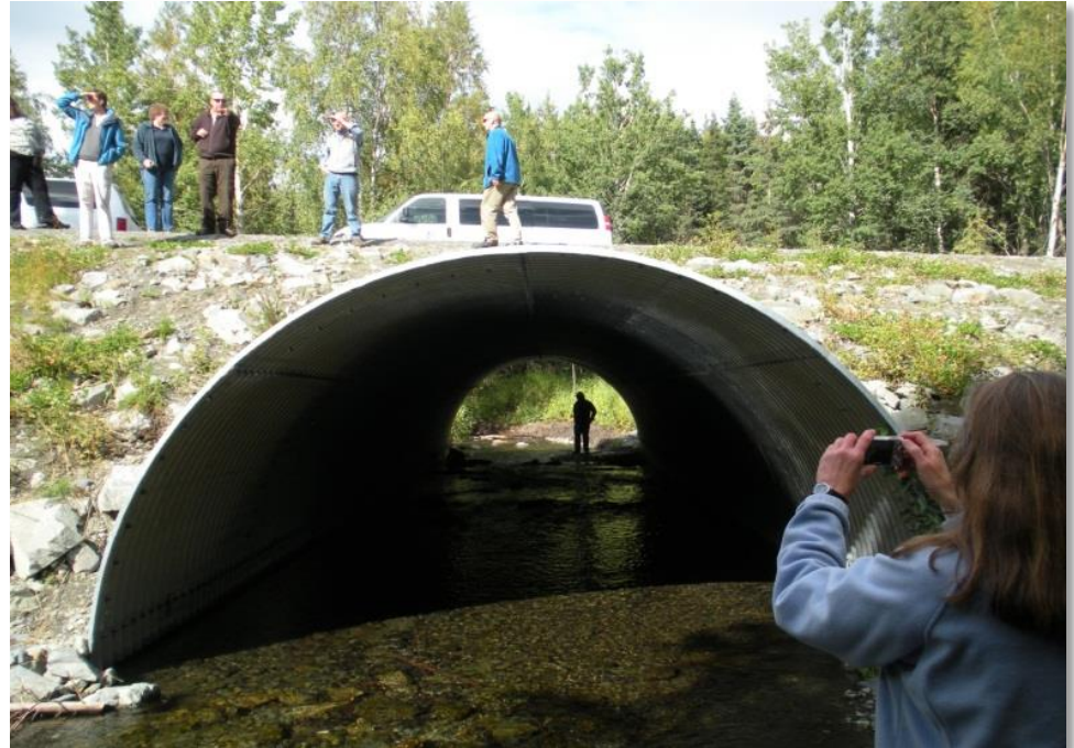
Kenai NWR, Skilak Loop Road Culvert replacement for aquatic passage; many partners (State/locality-delivered)
