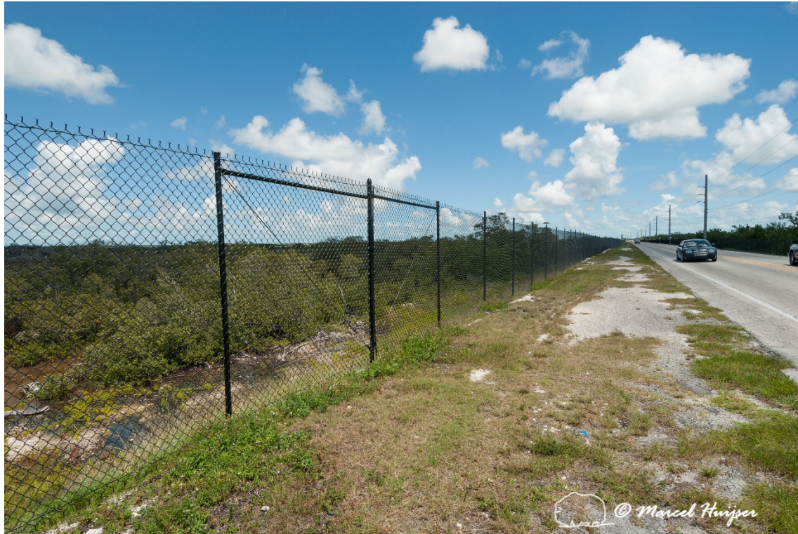
Figure 4: The wildlife fence to Keep Key deer off US Hwy 1, Big Pine Key, Florida.
