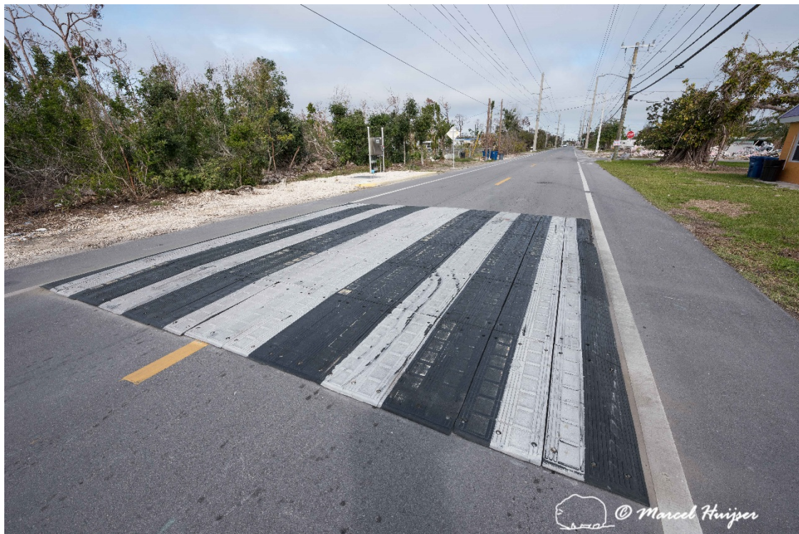
Figure 13: Speed bump (with cross walk pattern) aimed at reducing Key deer-vehicle collisions on one of the secondary roads, Big Pine Key, Florida.
