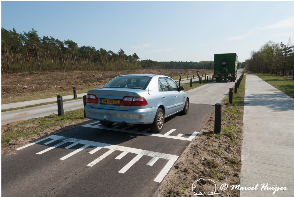
Figure 35: At-grade crossing opportunity for large mammals at a gap in the fence with speed bumps, The Netherlands.
