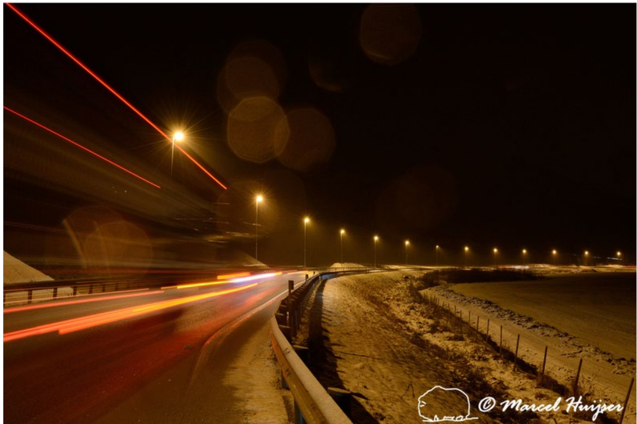
Figure 34: Street lighting to increase the visibility of moose to drivers, Norway.
