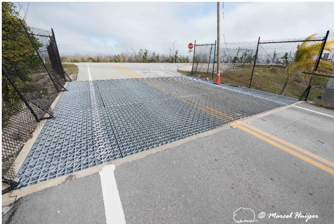
Figure 7: A wildlife guard at one of the side roads of US Hwy 1, Big Pine Key, Florida.
