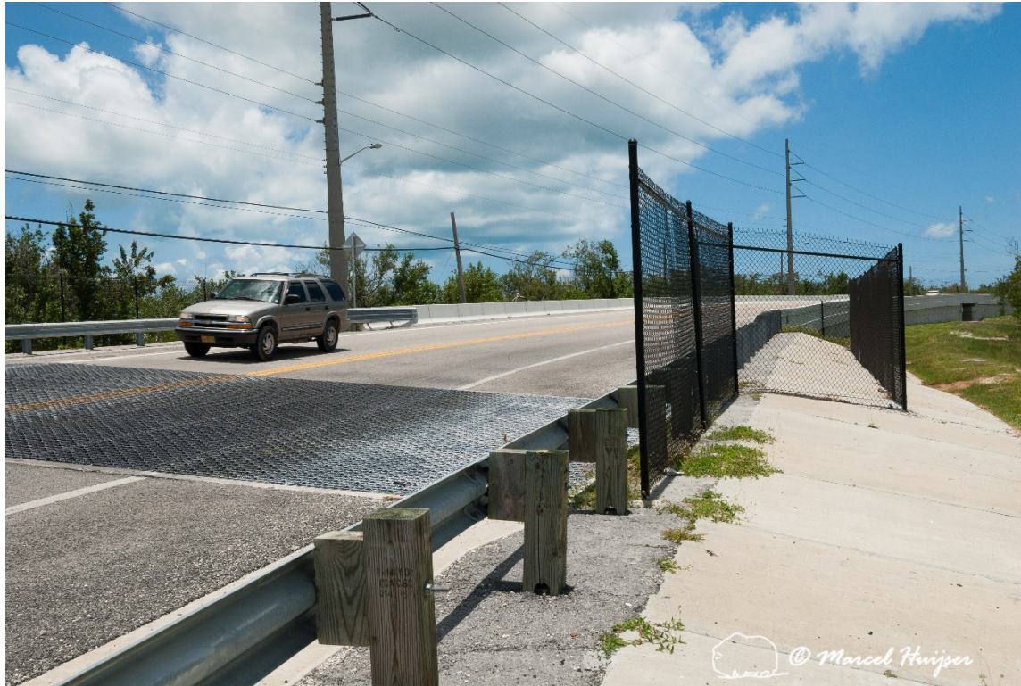
Figure 6: The wildlife guard at the fence end, US Hwy 1, Big Pine Key, Florida.
