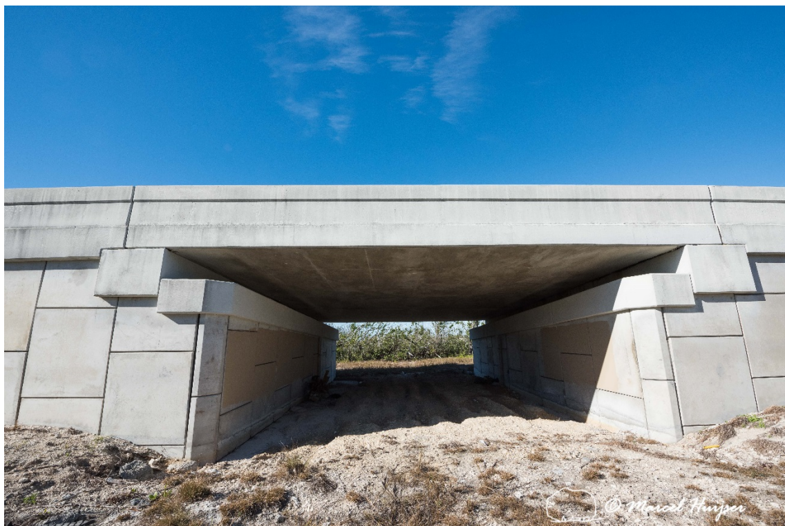
Figure 5: The northern wildlife underpass aimed at providing safe crossing to Key deer and other wildlife, US Hwy 1, Big Pine Key, Florida.
