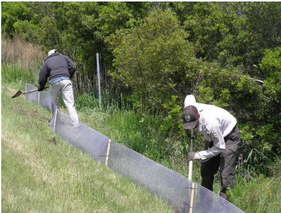
Figure 7: The plastic netting fence, Fisherman Island NWR, Virginia, present for the 2008 and 2009 nesting seasons only (Photo credit USFWS).
