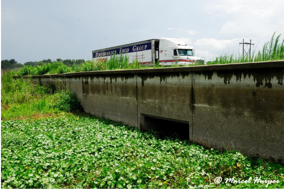
Figure 27: Example of a “wet” underpass and barrier wall for reptiles, amphibians and small mammals, U.S. Hwy 441, Paynes Prairie Ecopassage, south of Gainesville, Florida, USA.
