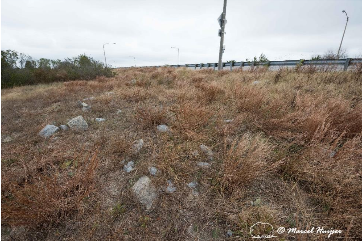
Figure 18: Roadbed with rocks on the north side of Fisherman Island (west side of US Hwy 13), resulting in uneven surface making installation of the 20 ft long concrete barriers a challenge.
