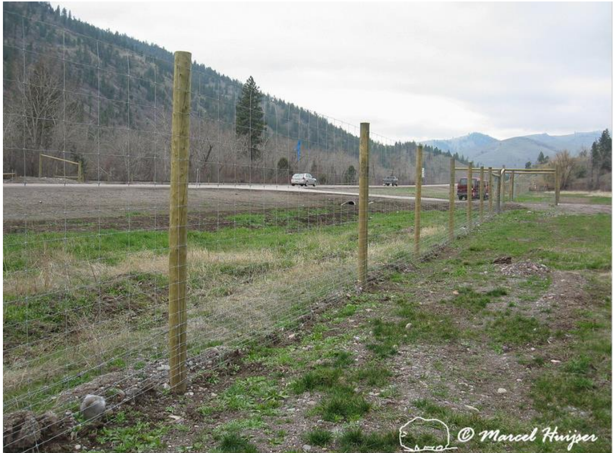
Figure 36: Wildlife fence (8 ft tall smaller mesh size towards bottom), U.S. Hwy 93, near Ravalli, Flathead Indian Reservation, Montana, USA.
