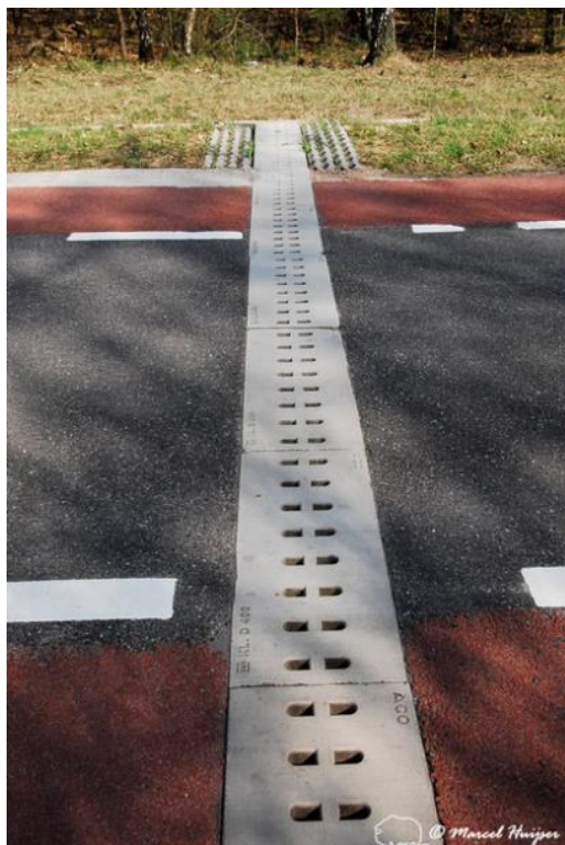
Figure 30: Example of an amphibian tunnel (ACO) with an open slotted roof embedded in the pavement under a 2-lane road, Deelenseweg, between Hoenderloo and Arnhem, Gelderland, The Netherlands.
