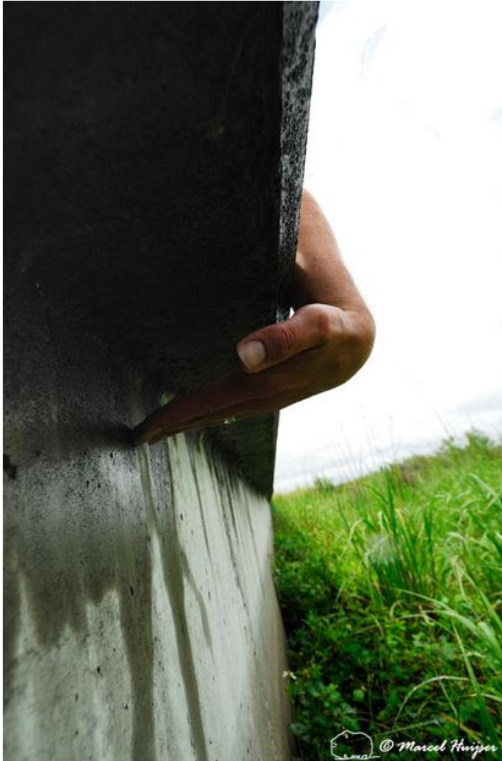
Figure 21: Concrete barrier wall (1.1 m tall) with overhang or ‘lip’ (15.2 cm) for reptiles, amphibians and small mammals, U.S. 441, Paynes Prairie Ecopassage, south of Gainesville, Florida, USA.
