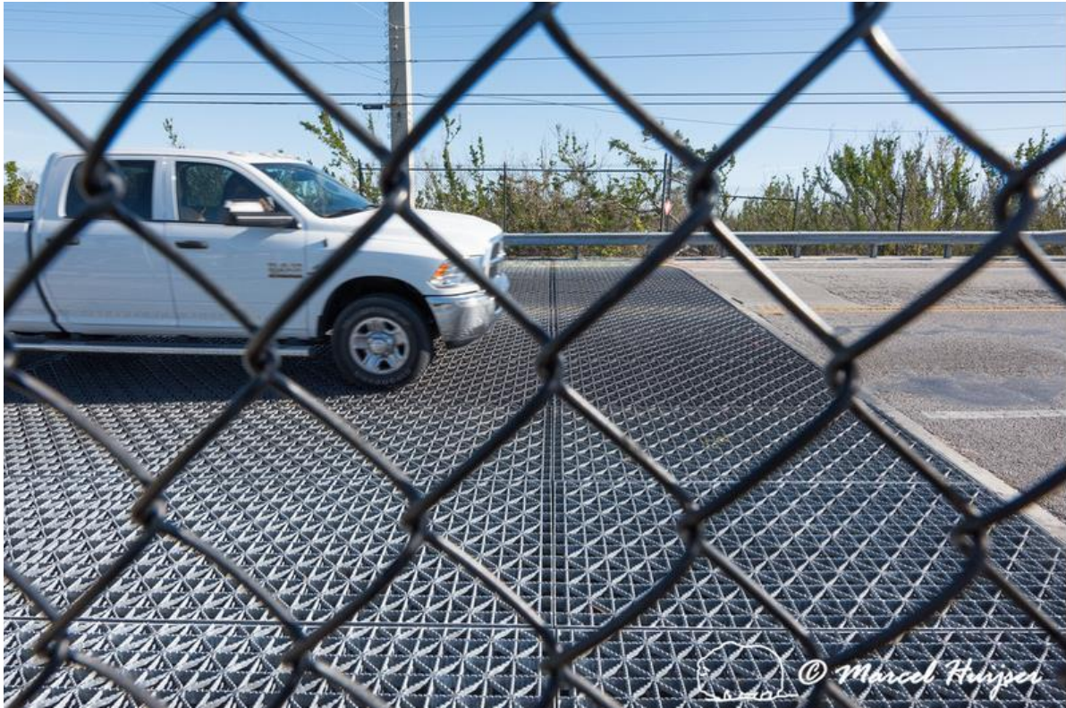
Figure 37: Wildlife guard at fence end on U.S. Hwy 1, Big Pine Key, Florida, USA.
