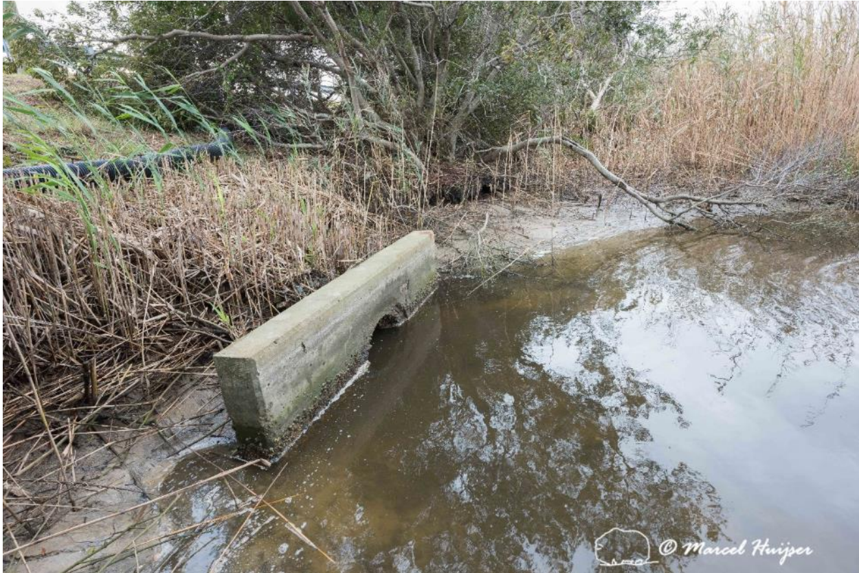
Figure 26: The existing culvert under highway (west side) that may or may not be used by northern diamondback terrapins ( Malaclemys terrapin terrapin ), Fisherman Island National Wildlife Refuge, Virginia. It is a 24” Reinforced Concrete Pipe (RCP) (Pers. com. Timothy R. Holloway, Chesapeake Bay Bridge-Tunnel). It is subject to tidal influence.
