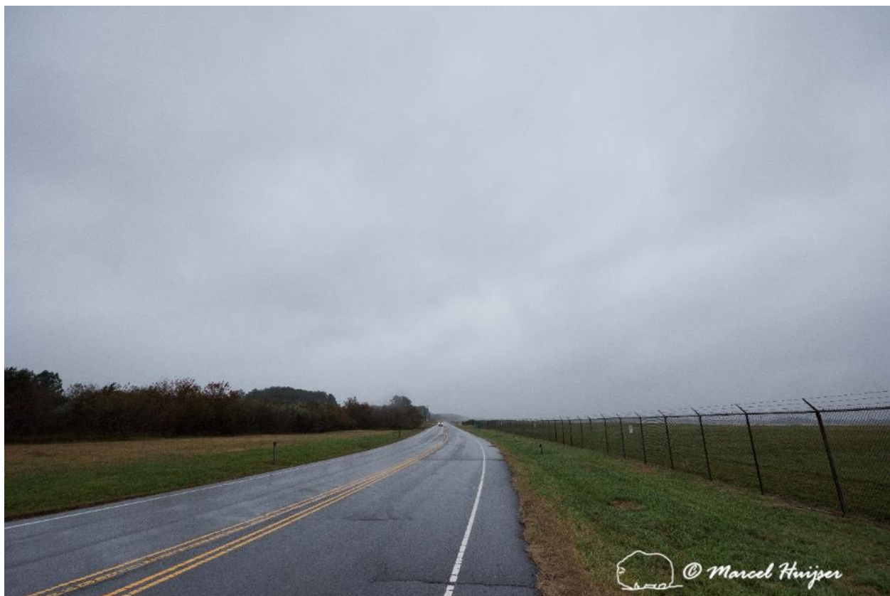
Figure 35: Hwy 175 adjacent to Wallops Island National Wildlife Refuge and NASA Wallops Flight Facility (other side of fence), Wallops Island, Virginia, USA.
