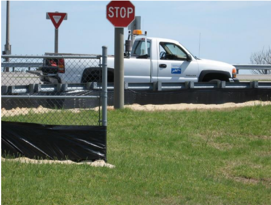
Figure 6: The silt fence, Fisherman Island NWR, Virginia, considered an ineffective barrier and (partially) present for 2007 nesting season only (Photo credit USFWS).
