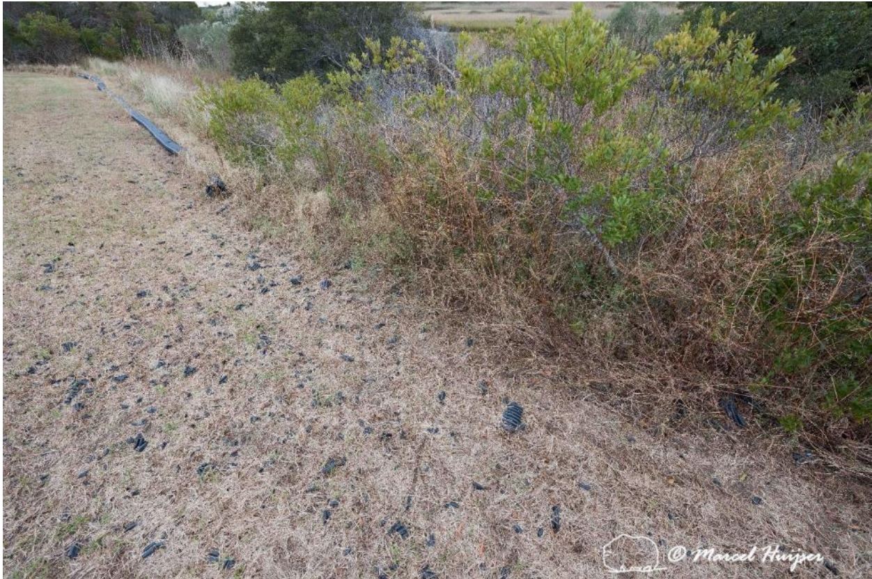
Figure 11: The plastic corrugated pipe can be destroyed by mowing equipment, Fisherman Island NWR, Virginia, present 2010 through 2018 nesting seasons.
