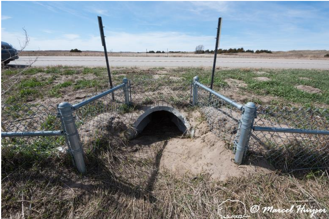
Figure 28: Example of a dry culvert (no openings in roof) used by turtles under a 2-lane road, Valentine National Wildlife Refuge, Ballard's South, Valentine, Nebraska, USA.
