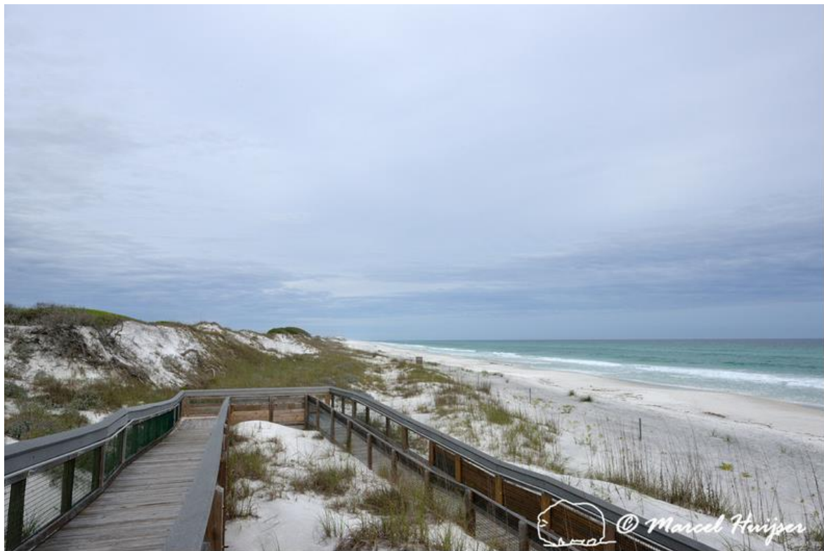
Figure 52: Boardwalk across coastal dunes to reduce erosion, east of Seagrave Beach. Florida, USA.
