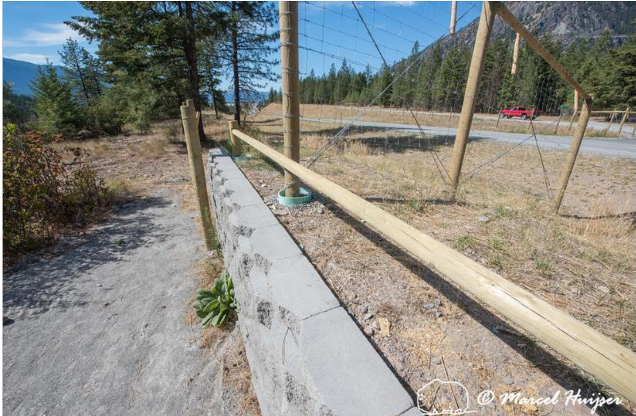
Figure 39: Wildlife jump-out, near Thompson Falls, Montana, USA. Note the horizontal bar that increase the effective height for animals that want to jump into the fenced road corridor.
