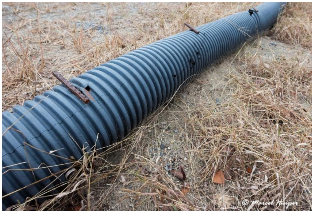
Figure 9: The plastic corrugated pipe is staked down with rebar, pinning the pipe close to the ground to reduce the likelihood of diamondback terrapins crawling under the pipe, Fisherman Island NWR, Virginia, present 2010 through 2018 nesting seasons.
