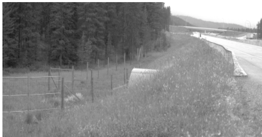
Fence at wildlife crossing is intended to restrict animal movement across the road and to funnel wildlife toward crossing structures.
