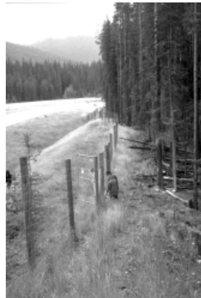
Wildlife fencing set back from road to provide safe area for animals caught on wrong side of fence.
