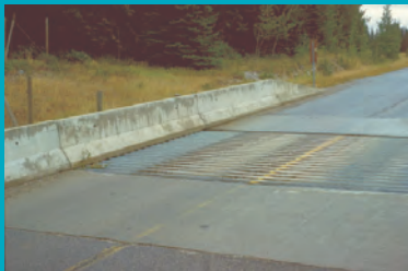
Typical cattle guard (size varies). Crossbars approximately 8" on center. Use guards on all roads and driveways connecting to U.S. 93 in areas with continuous fencing.
