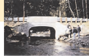
Box Culvert (after construction)
