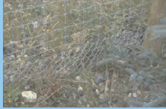
Typical continuous chain link apron dig barrier located below grade at a 45 degree angle. Dig barrier joins typical fence mesh pattern at 12"-18" above grade.
