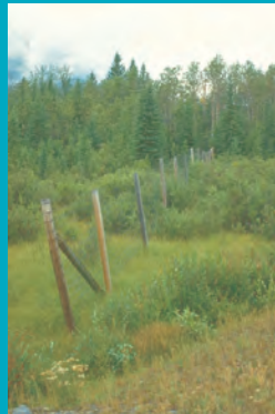
Typical 8' high page wire fencing. Posts are approximately 10' on center.
