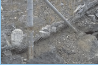
Typical continuous chain link apron dig barrier located below grade at a 45 degree angle. Dig barrier joins typical fence mesh pattern at 12"-18" above grade.
