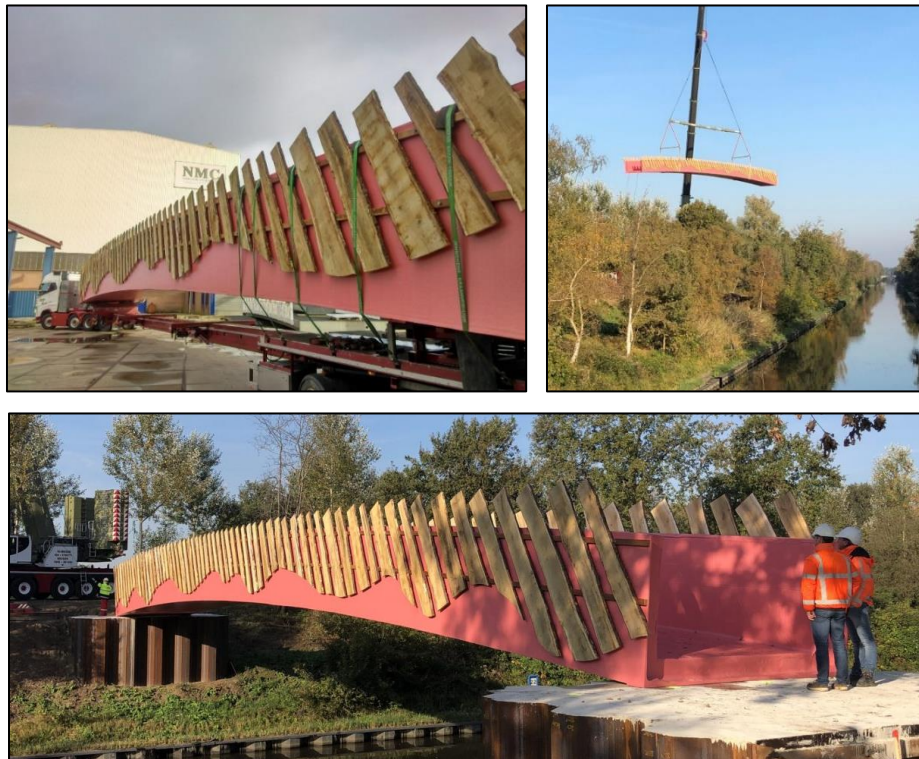
Figure 10: Installation of a uni-mold FRP ecoduct near Eindhoven, The Netherlands. Bridge is 36m x 3.5m [63]. Top left; bridge is delivered in one piece from the factory to the construction site. Top right; bridge is lifted into place using one crane. Bottom; FRP ecoduct is placed onto abutments over a canal.
