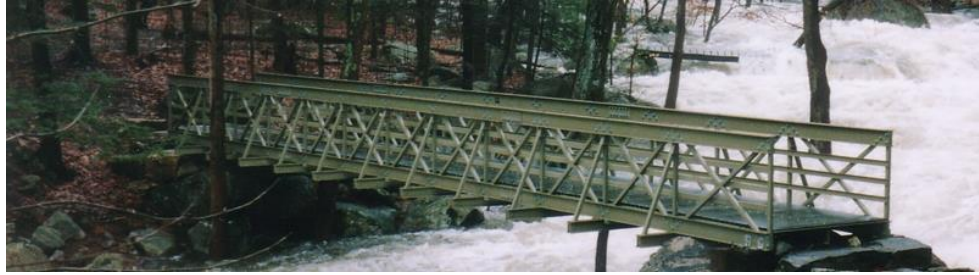
Figure 11: Example of a pedestrian bridge built by Creative Pultrusions. This bridge is in Bear Mountain, New York, and is 62ft x 6ft with a strait design using FRP railings for trusses and FRP decking for the walkway.
