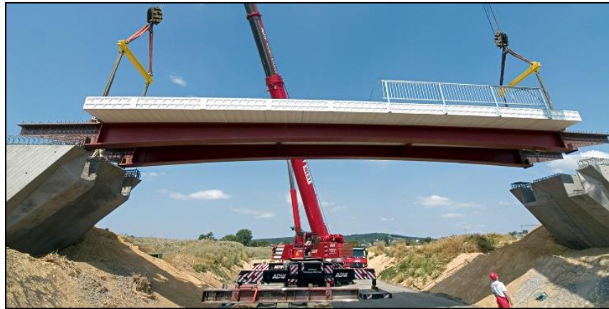
Figure 6: A 21.5 m FRP deck placed on top of steel girders to create a traffic bridge over B3 highway in Germany [50].
