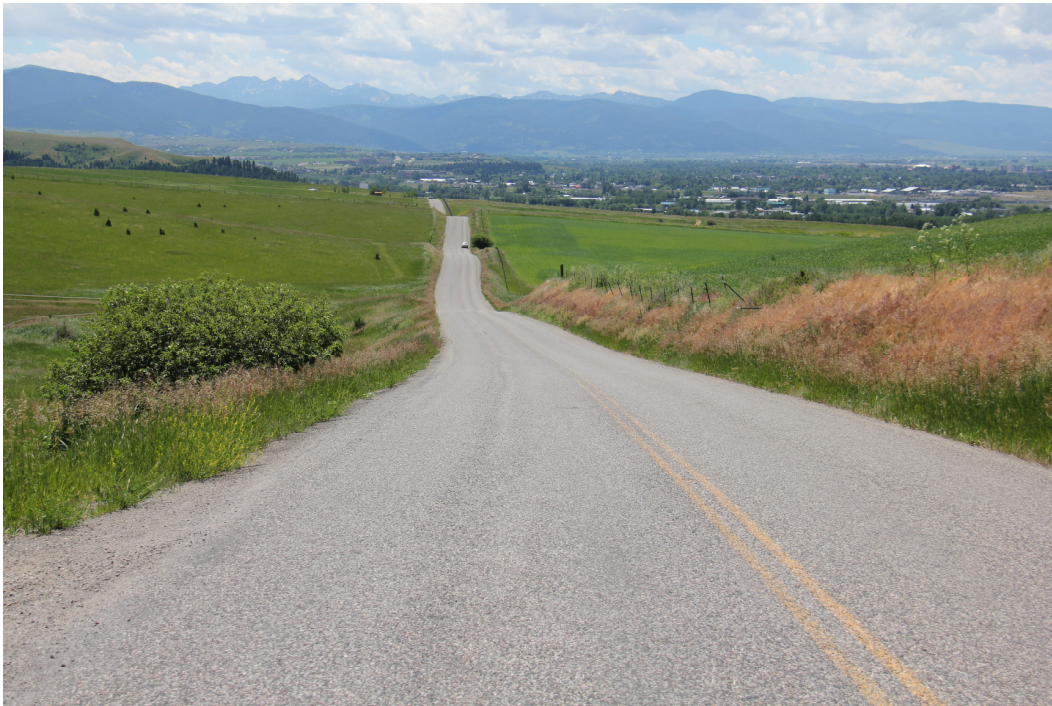
Figure 12. Story Mill Road looking south (section N2-b). Ditches are very small and there are several areas of thru-cuts and steep slopes.
