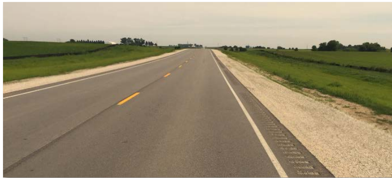
Figure 12. Poorly placed rumble strip (courtesy of Iowa DOT)
