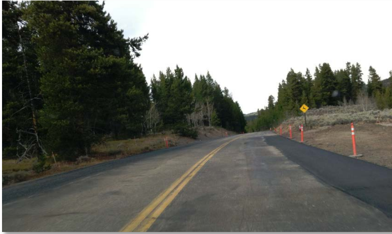
Figure 11. Shoulder widening on Highway 287 in Grand Teton National Park (2012)
