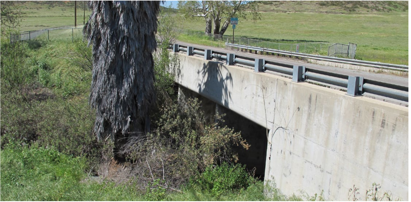
Figure 26: Image shows a 30 ft/9.1 m Type 3 concrete temporary stream bridge along Campo Road/Highway 94, San Diego County, south of San Diego. The bridge has three 10 ft × 10 ft concrete chambers and was built without specific wildlife goals. Image: Tom Langton
