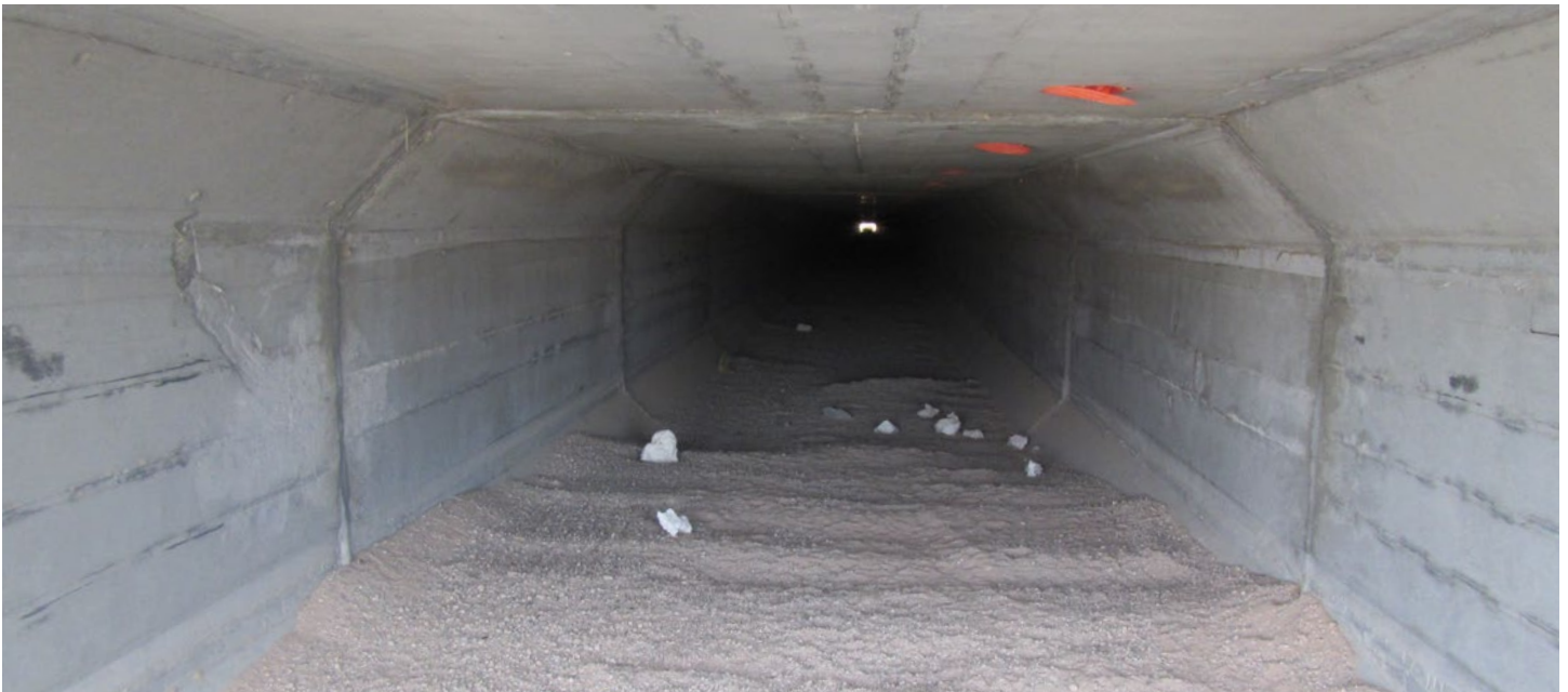
Figure 29: With a large median and easements under a four-lane highway, desert culverts can be extremely long (over 300 ft /90 m) and dark during the day. The view foreground here is lit by a camera flash. Image: Cheryl Brehme
