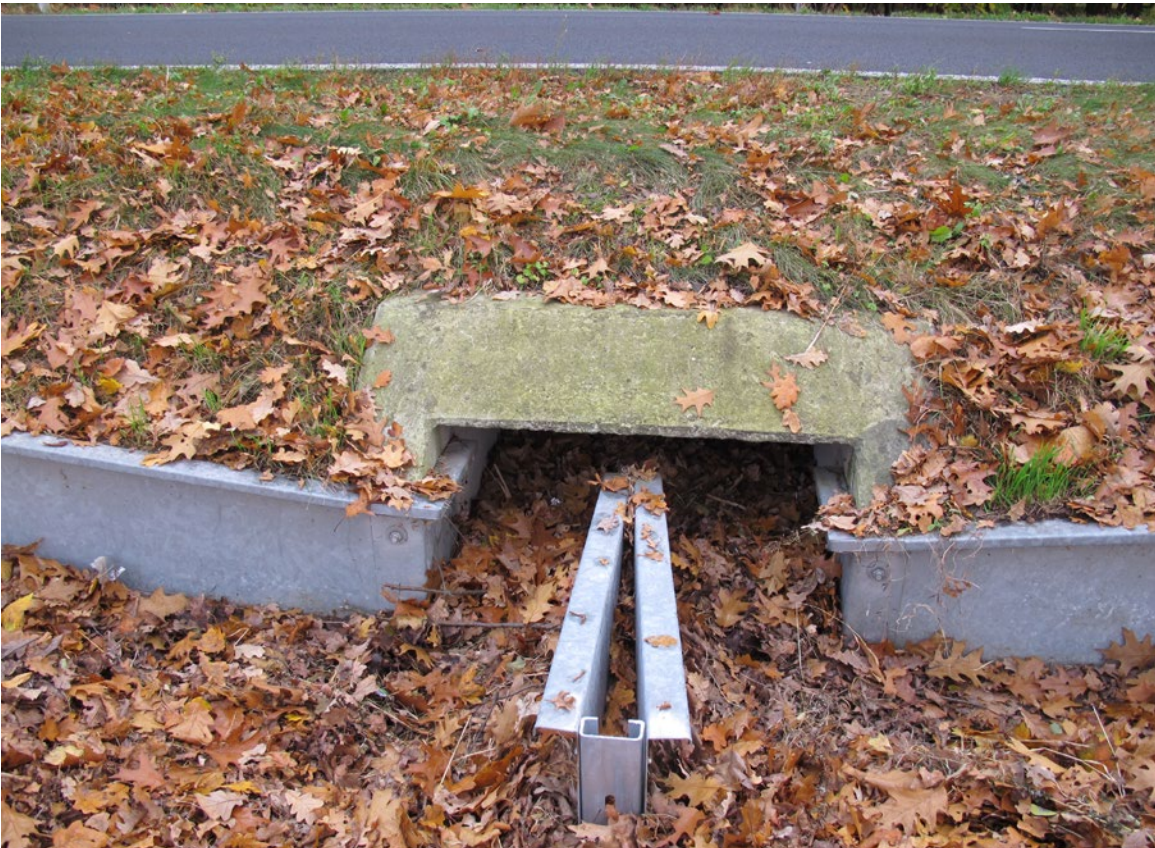
Figure 45: A small ‘bottomless’ or ‘stilt’ passage (cast concrete roof and sides on foundations, with a natural soil base) under a 2-lane road. There is an extensive late-season leaf litter component that amphibians shelter under. The barrier and deflection panel are made from galvanized sheet metal fence material with an overhang. Image: Tom Langton
