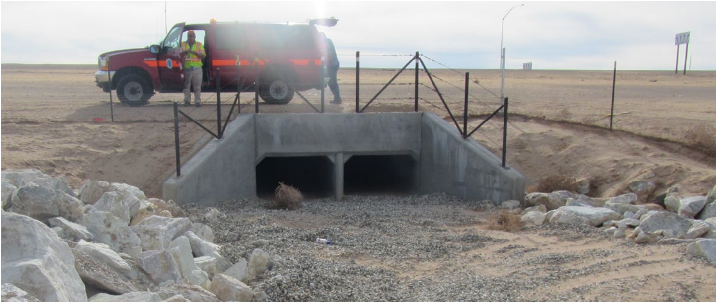
Figure 28: A new culvert built under State Route 58 in southern California (Hinkley Highway Re-alignment Project, Caltrans District 8). Adjustments will be needed to join wire fencing to the entrance of the passages and to make the rip-rap safe, so desert tortoises do not get trapped in it. Image: Cheryl Brehme
