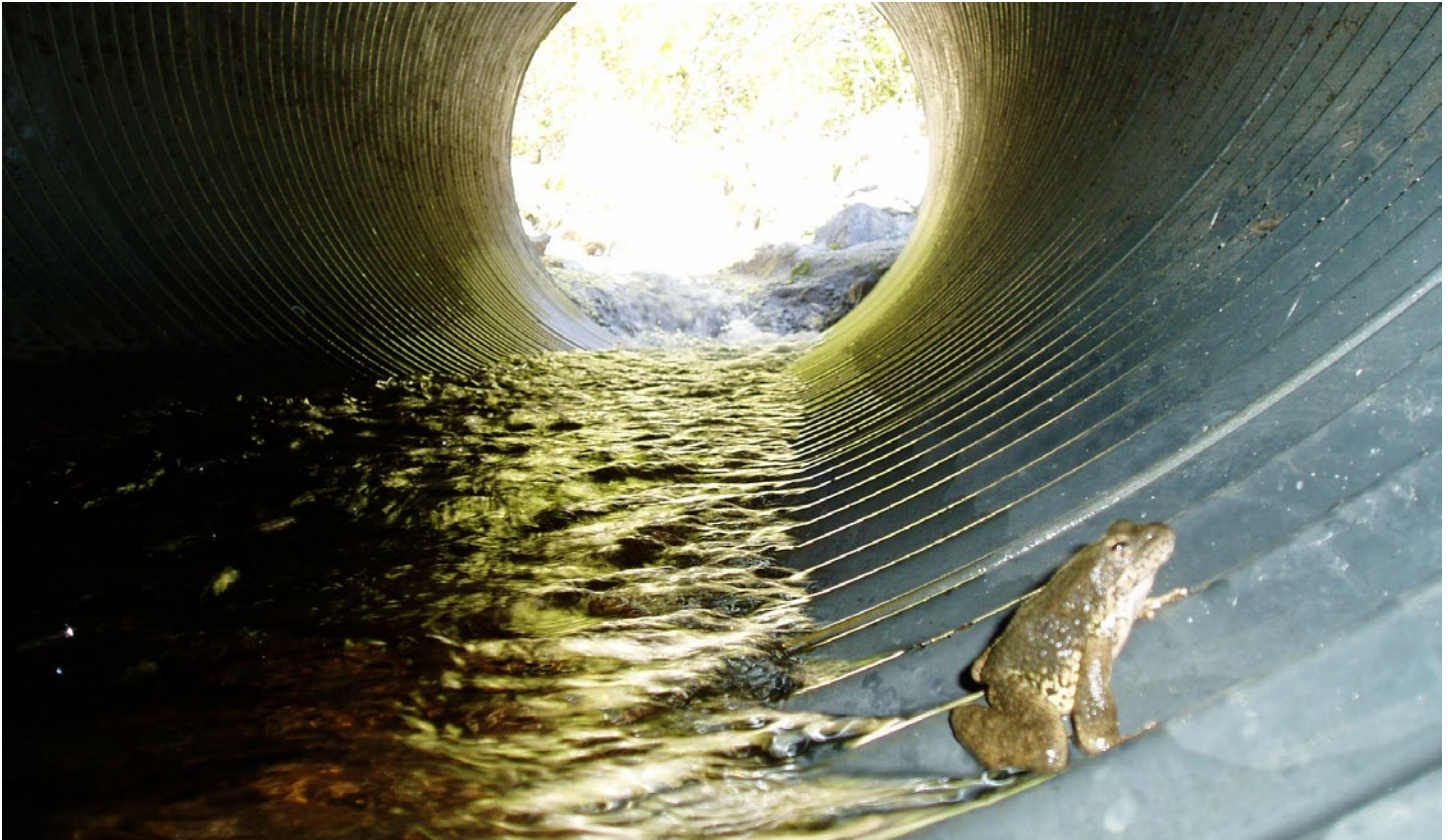
Figure 76: Corrugated culverts without a flat base may be difficult to navigate for some species. Here a foothill yellow-legged frog ( Rana boylii ) can be seen at the side of a corrugated metal passage under Highway 70 at the Shady Rest Area, Butte County, California. Image: Garcia and Associates. See: Garcia and Associates. 2008.
