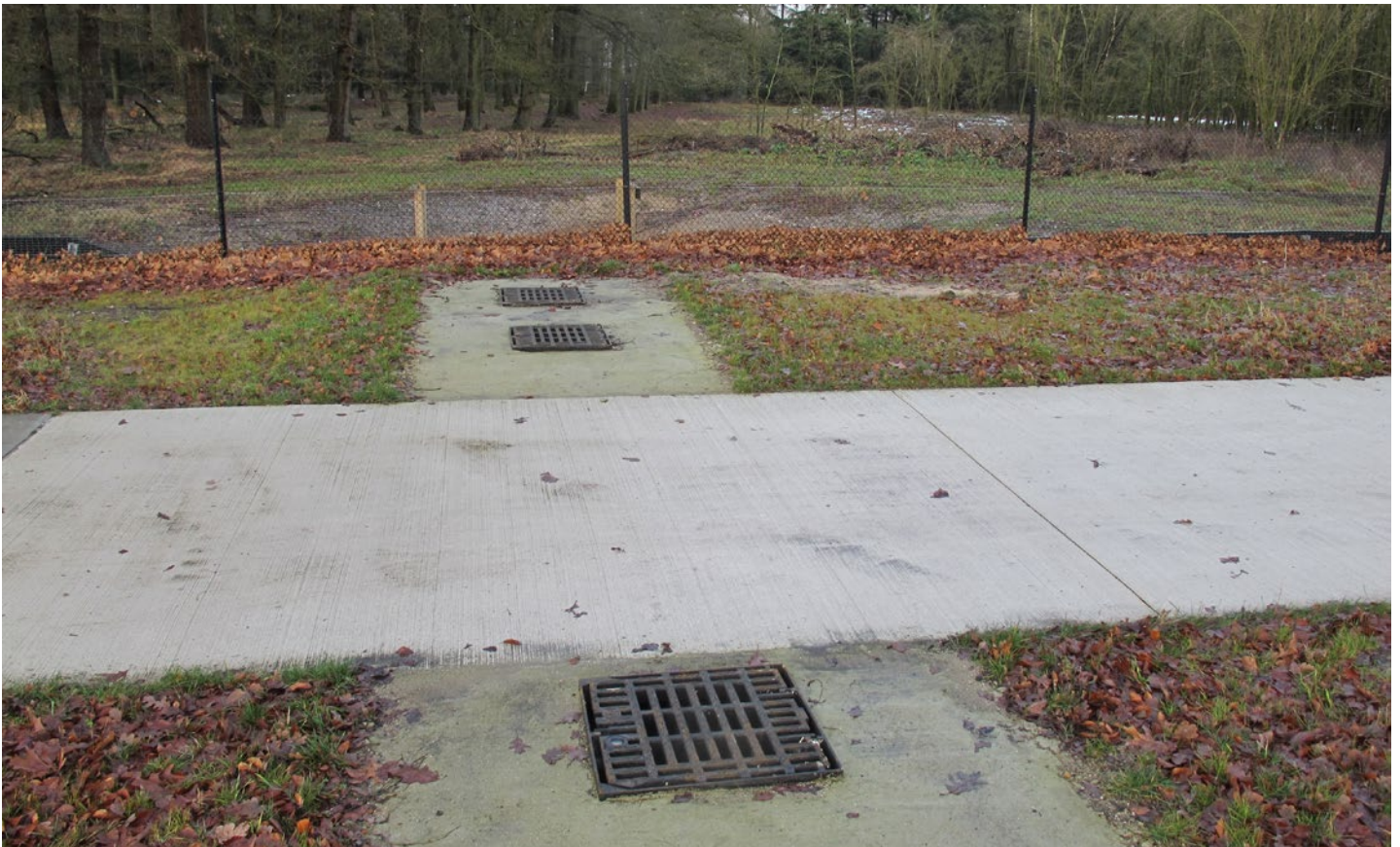
Figure 31: Located on the far side of the road shown in Figure 30 and either side of the cycle lane is a series of cast steel gratings placed within the roof of the wildlife passage to allow entry of light and moisture. Image: Tom Langton
