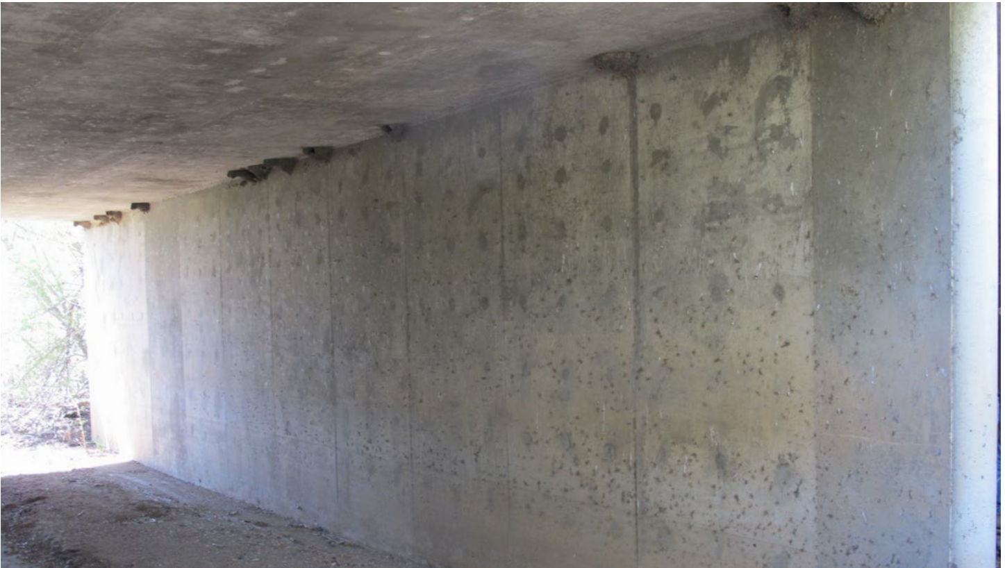
Figure 27: From the same structure shown in Figure 26, one of the chamber dividing walls. These chambers can be scoured out by seasonal heavy stream flow and flash flooding, but may also be used by nesting birds as well as mammals, such as the kangaroo rat ( Dipodomys californicus ) which has excavated soil in the base of this structure. Image: Tom Langton
