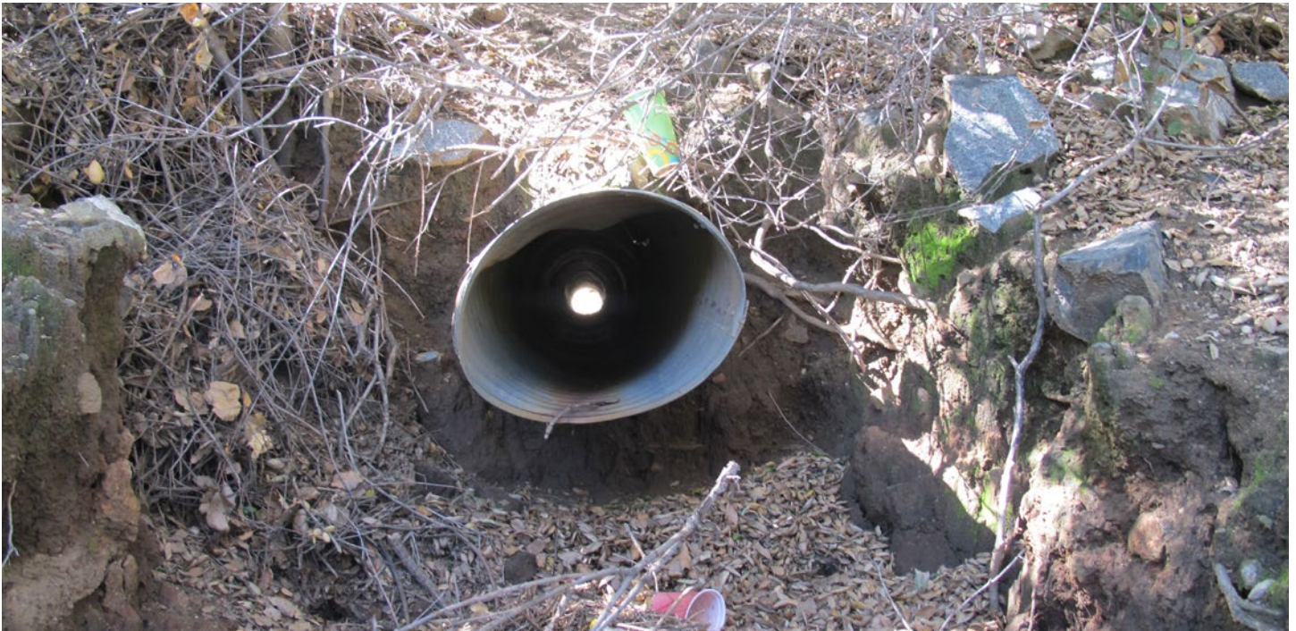
Figure 38: There are many small cross-road steel drainage culverts on California roads, such as this elliptical shaped steel culvert near San Diego. This culvert was built during the last century and is nearing time for refurbishment. This type of scenario offers an opportunity for culverts to be adapted for safe wildlife passage as well as for road drainage purposes. See also Chapter 9. Image: Tom Langton
