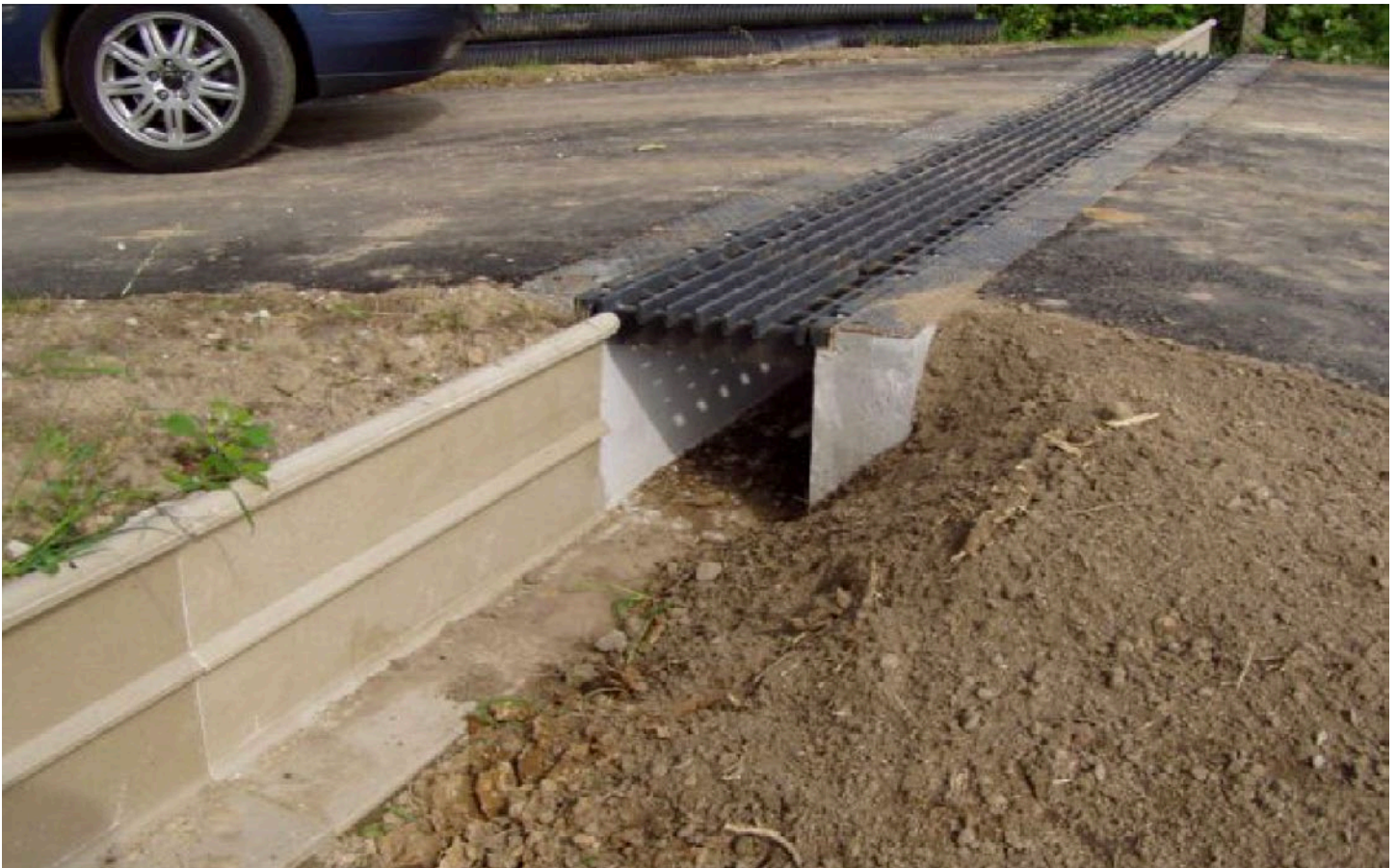
Figure 60: A purpose-made 'stop grid', built where a side road approaches a main road in a herp migration location. Gratings may be made with wider gaps but must conform to road regulations. Image: ACO
