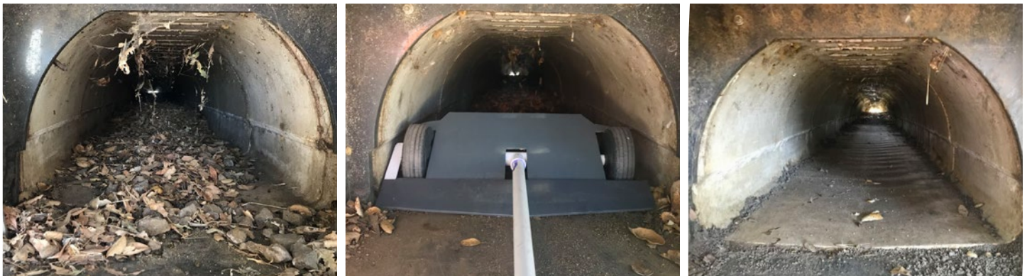
Figure 71: Blown leaves may in some locations fill and become compacted in a small passage thus reducing wildlife use. An extending pole device can clear them as shown in this slotted surface passage. Image: Michael Hobbs.
