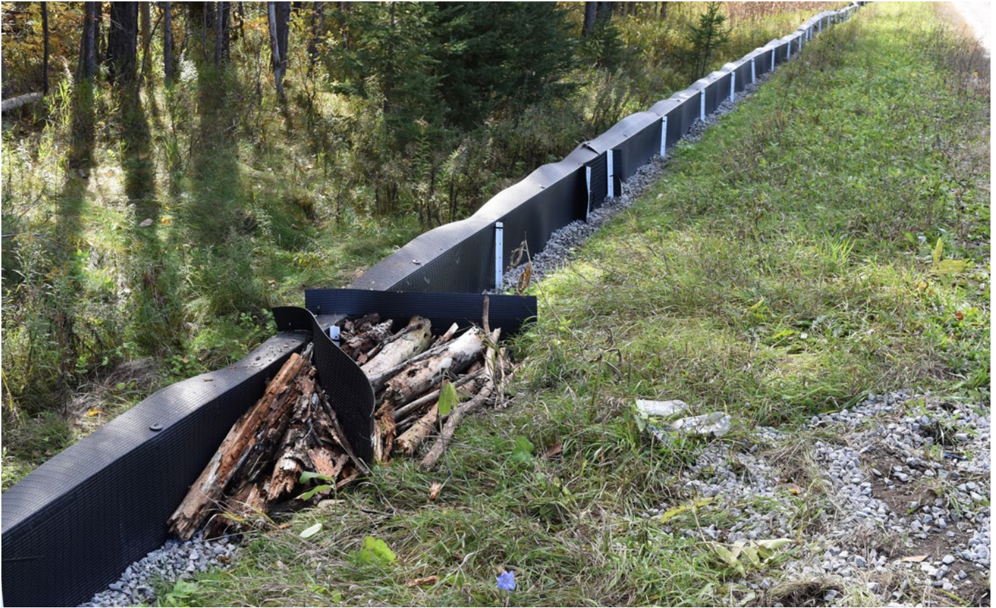
Figure 62: A jump-out constructed within a section of solid HDPE sheet fence, constructed along a road edge. The jump-out is outfitted with decaying logs to form a ramp for small turtle species and it directs them to the safe side of the barrier. Image: Animex fencing
