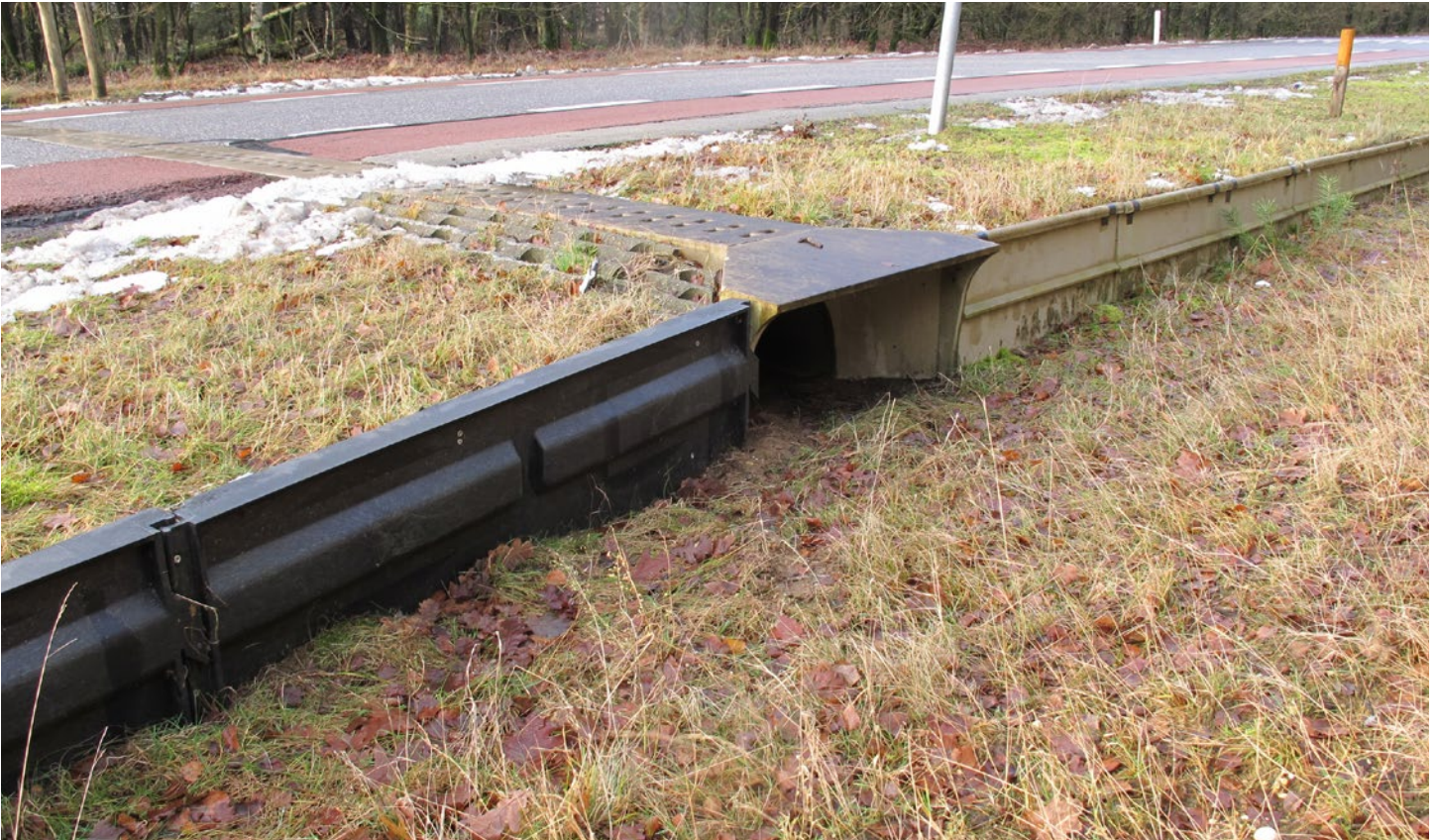
Figure 48: Guide walls for small snakes and lizard species on a single lane road with cycle path. Attached to a Type 5 (20 in/0.5 m wide) micro-passage, is a molded plastic barrier on the left hand side and a polymer concrete barrier on the right hand side. Both barrier types are circa 20 in/0.5 m above ground. Image: Tom Langton
