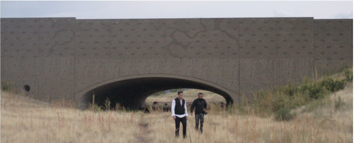
Figure 24: A Type 2 underpass in the Sonoran Desert in Arizona, constructed for passage by deer and bighorn sheep. The passage crosses under a 6-lane road with a median. It is a purpose-built, 50 ft wide, 12 ft high, and 190 ft long (15.2 m wide, 3.6 m high and 58 m long) structure is located at Oracle Road, near Tucson, Arizona. Image: Tony Clevenger.
