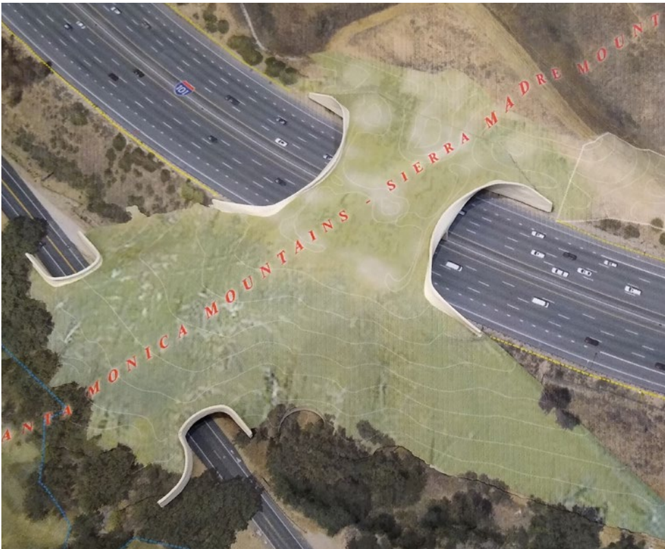
Figure 18: Design model for a large Type 1C multi-road wildlife overpass crossing at Liberty Canyon (Agoura Hills, CA). Image: Simulations: #SAVELACOUGARS & NATIONAL WILDLIFE FEDERATION Image: Tom Langton.
