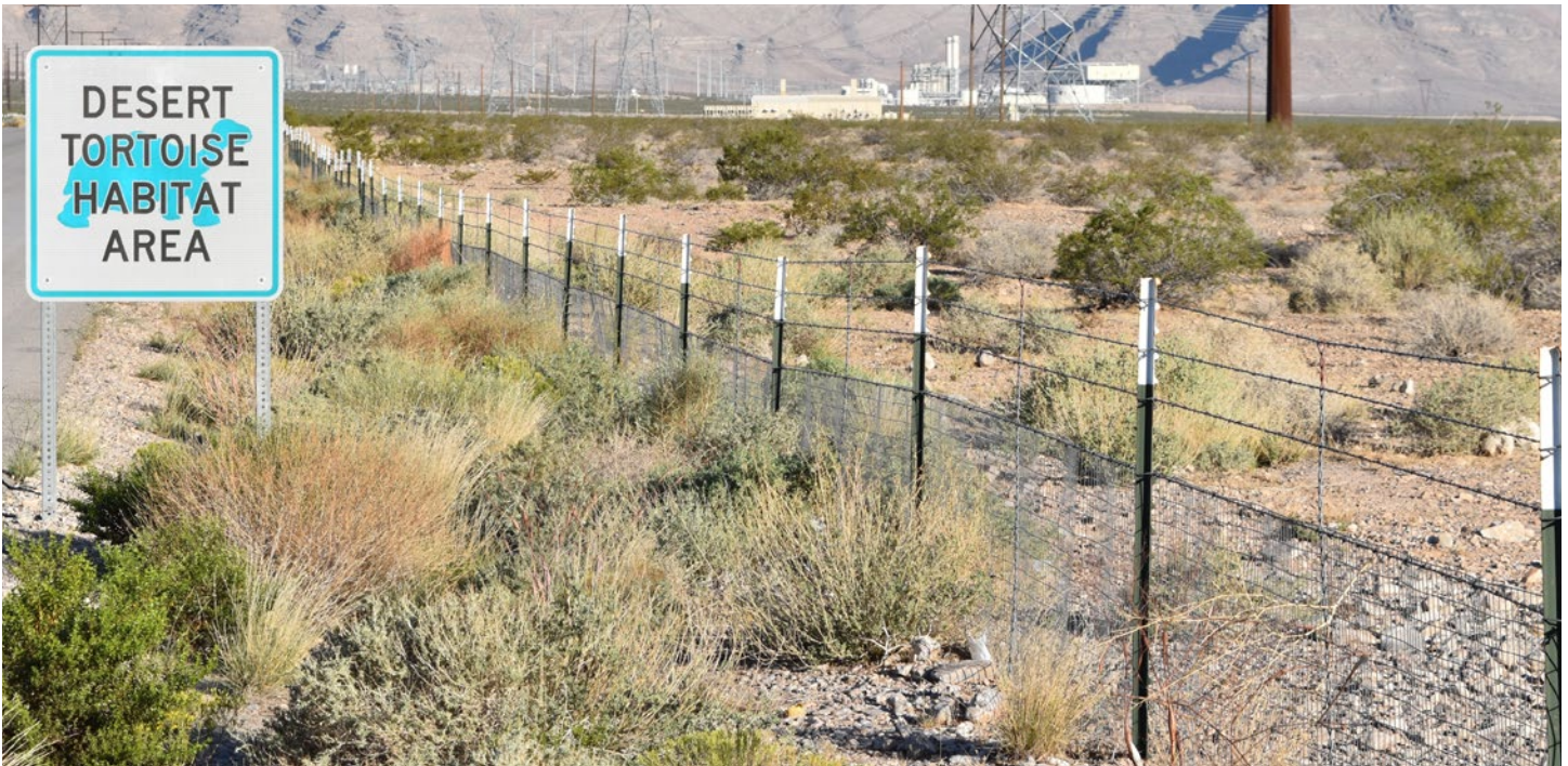
Figure 54: Typical wire mesh and stock fencing on metal posts in desert tortoise habitat. Image: Dean Swensson
