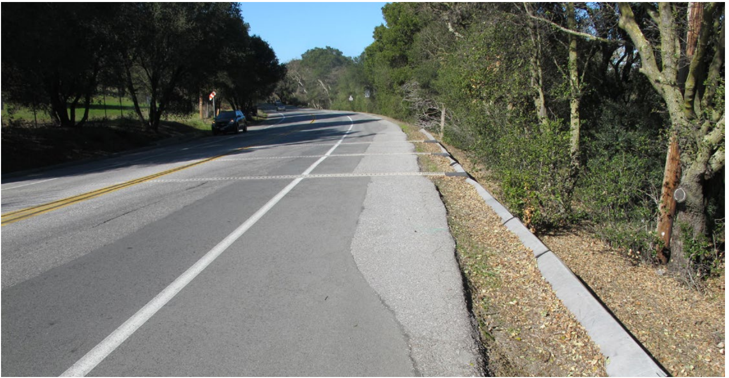
Figure 41: General alignment of three purpose-built polymer concrete slotted surface-passages with one-way plastic panel fencing, (shown) and mesh (not shown). Passages show as narrow grey lines across the road. These were built 2001 and 2003 next to Lake Lagunitas in Stanford, California, for California tiger salamander. Image: Tom Langton
