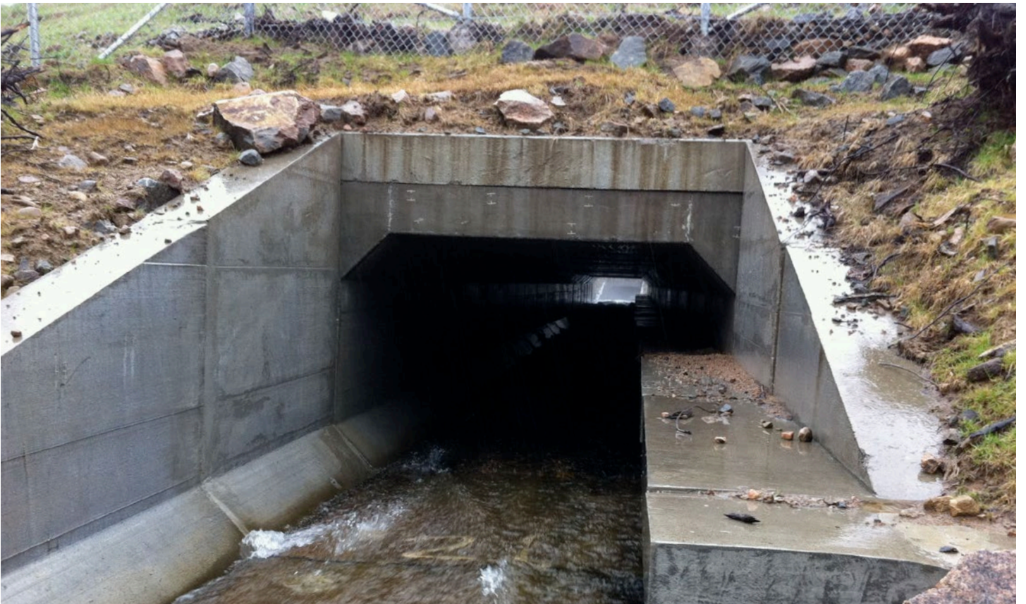
Figure 79: A cast-in-place concrete stream passage with a mammal shelf, that could be enhanced for use by herpetofauna with addition of directional fencing. Image: Tony Clevenger
