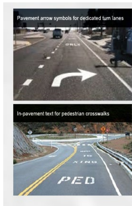
Figure 195: Examples of Pavement Symbols for Dedicated Turn Lanes & Pedestrian Crosswalks (Street views from Google Maps)
