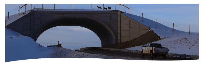
Figure 4: Wildlife crossing structure on US Highway 191 in Wyoming (photo courtesy of AFWA presentation).
