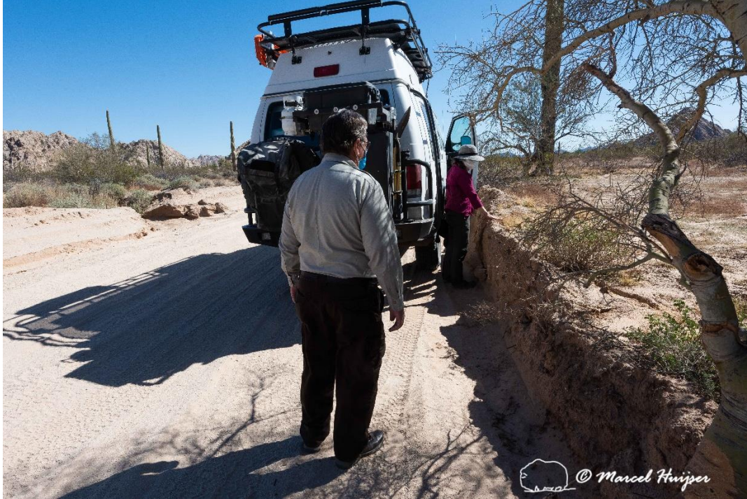
Berm (about 2.5 ft tall), primarily caused by erosion, along a widened section of El Camino del Diablo, about 7.3 miles from western boundary, Cabeza Prieta National Wildlife Refuge, Arizona ( 32^{\circ}14'48.906'' N 113^{\circ}50'47.453'' W).
