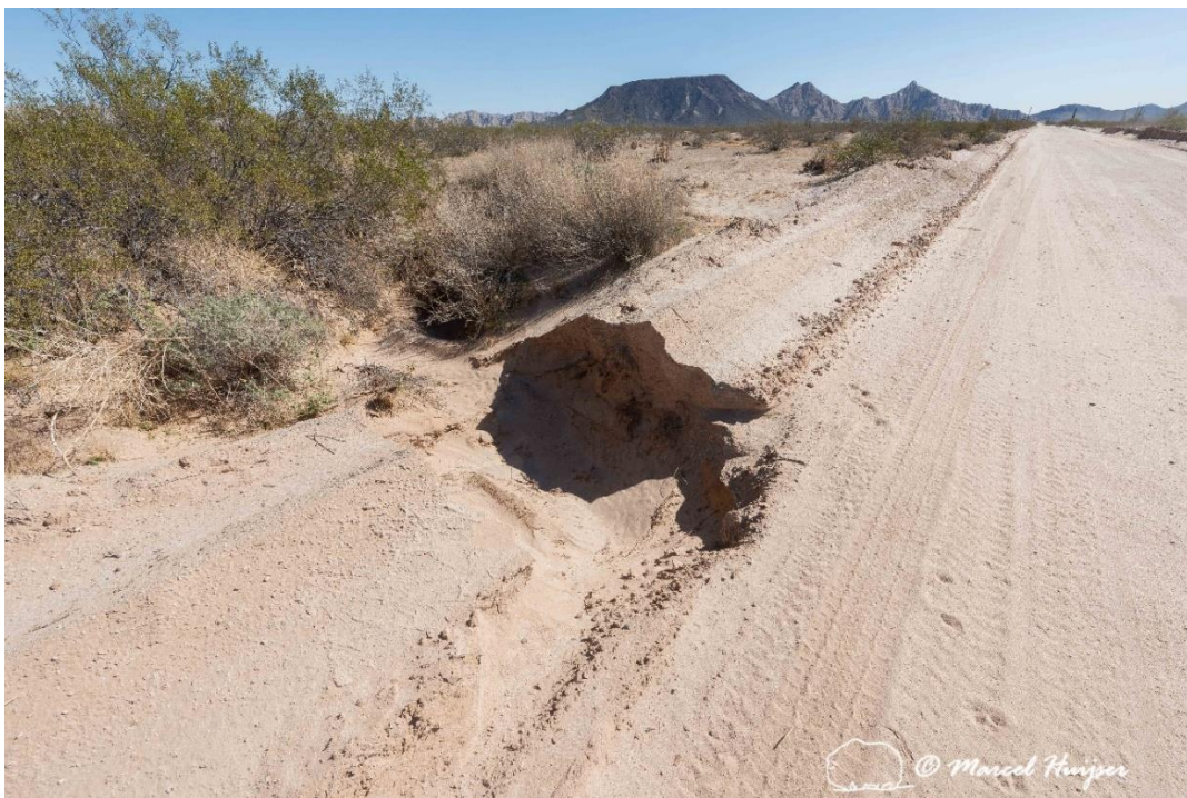
Berm (1-2 ft tall), primarily caused by grading, with runoff eroding across the berm, along a widened section of El Camino del Diablo about 3.1 miles from western boundary, Cabeza Prieta National Wildlife Refuge, Arizona ( 32^{\circ}15'53.004'' N 113^{\circ}54'42.503'' W).
