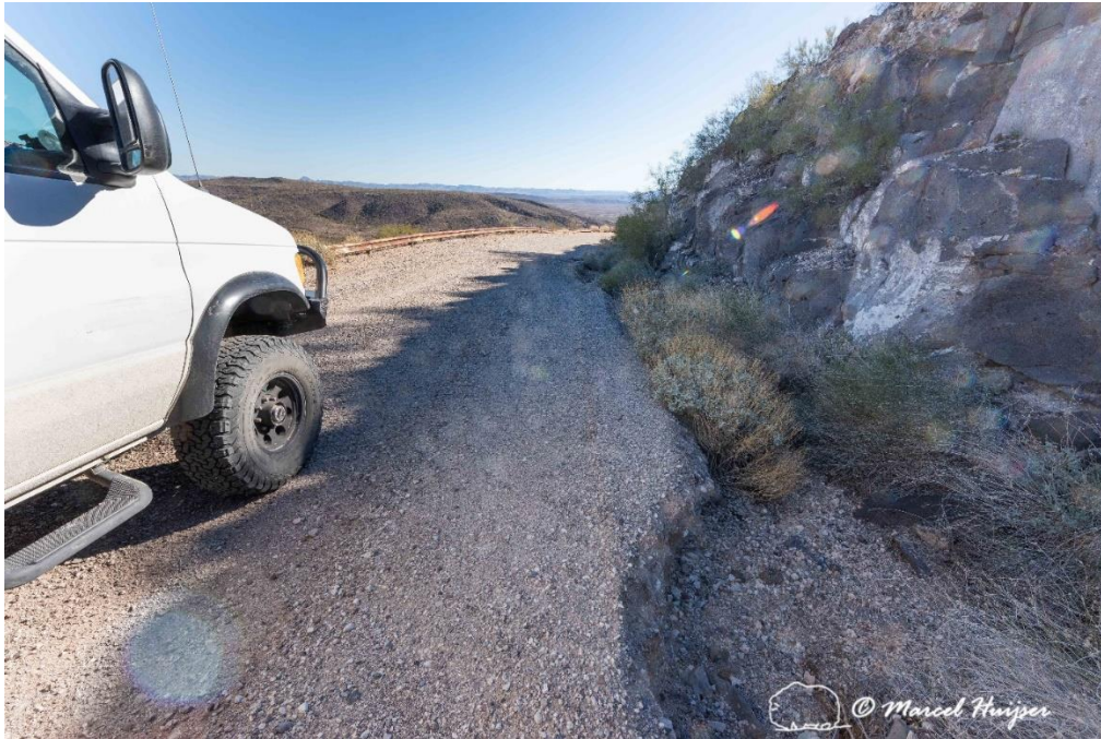
Erosion of the roadbed into the inboard ditch along the road to the Childs Mountain overlook (32°26'53.58"N 112°55'41.10"W).
