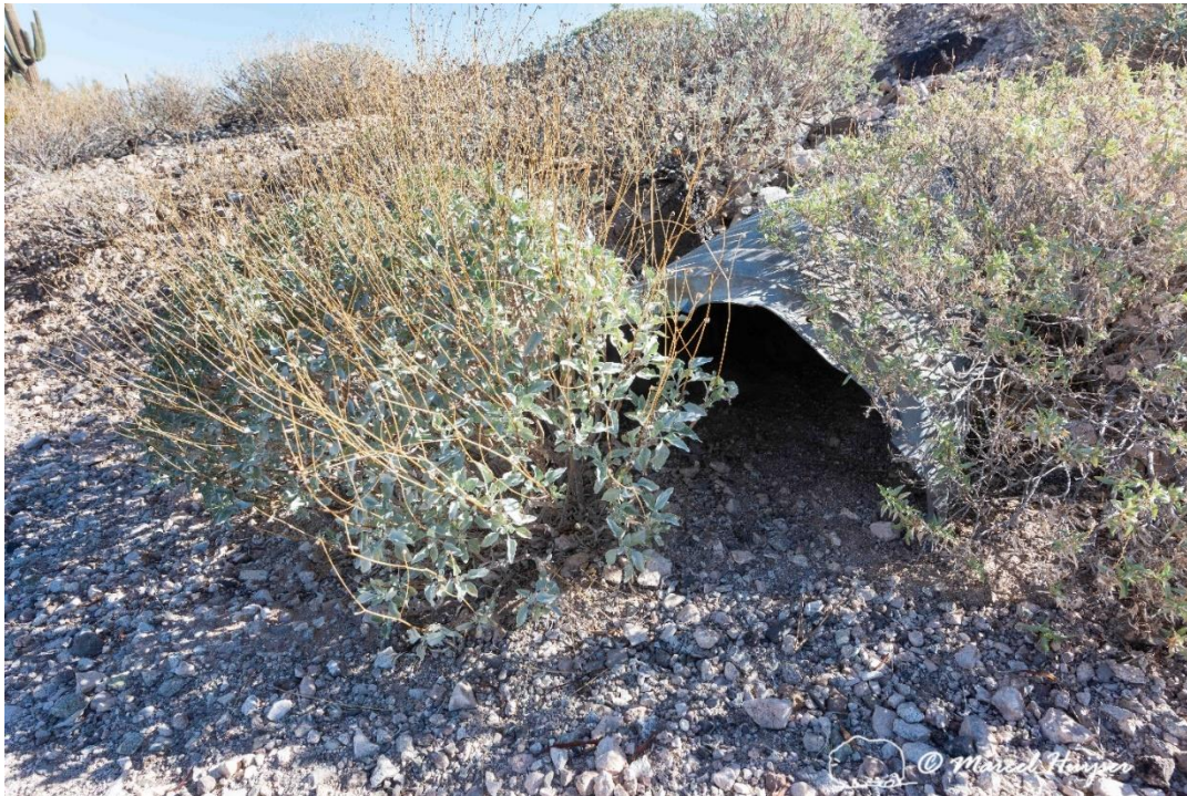
Partially clogged culvert under the road to the overlook, Childs Mountain, Cabeza Prieta National Wildlife Refuge, Arizona (32°26'34.25"N 112°55'39.26"W).
