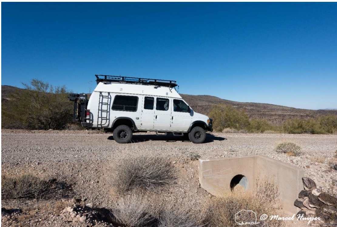
Culvert under the road to the overlook, Childs Mountain, Cabeza Prieta National Wildlife Refuge, Arizona (32°26'17.51"N 112°55'43.78"W).
