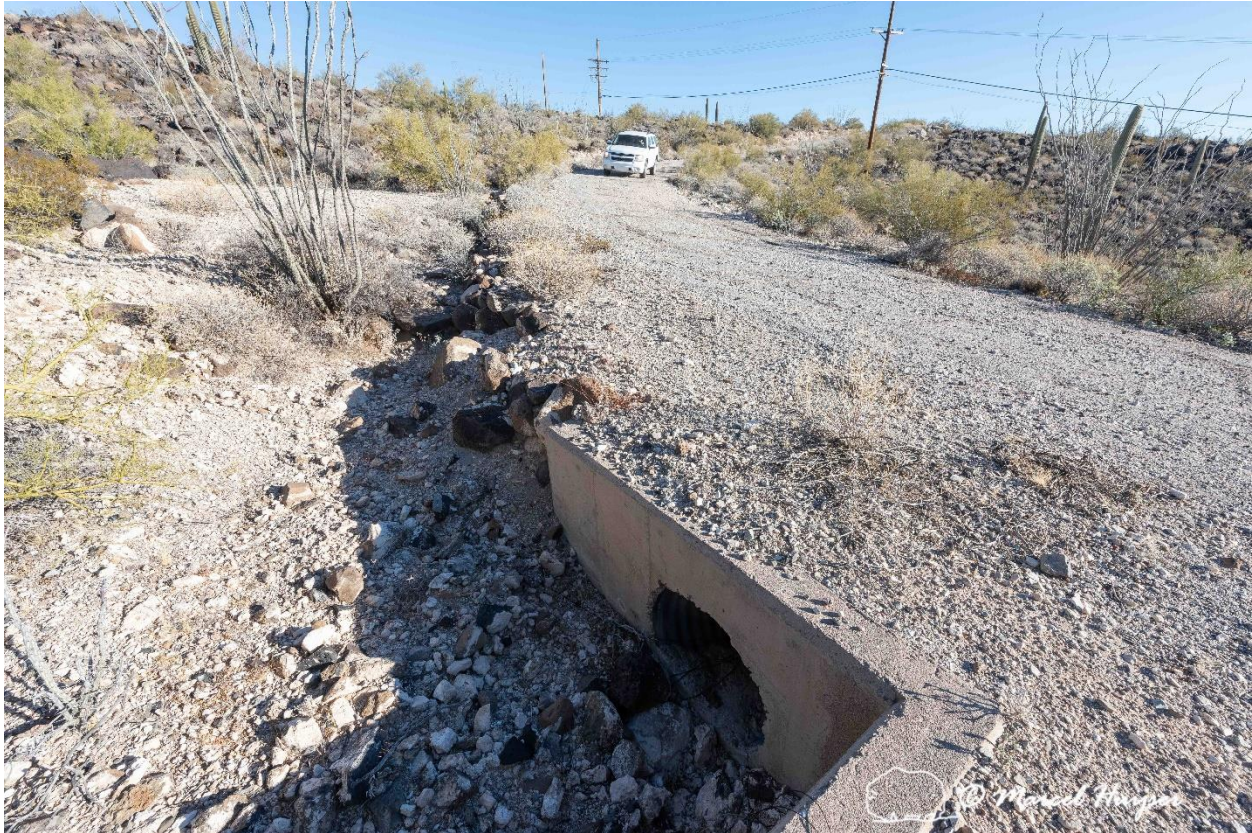
A culvert at an inboard ditch along the road to Childs Mountain overlook ( 32^{\circ}26'25.73''\text{N} 112^{\circ}56'57.82''\text{W} ).
