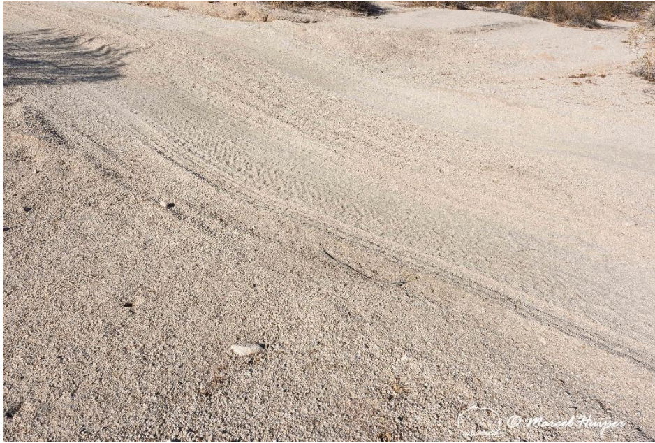
Detail of a rolling dip (possibly natural topography at the wash crossing rather than constructed) along the "old" section of El Camino del Diablo east of Tule Well, about 1.0 mile south-east of the junction with the Tule Extension road, Cabeza Prieta National Wildlife Refuge (CPNWR), Arizona ( 32^{\circ}11'26.573'' N 113^{\circ}42'54.144'' W).
