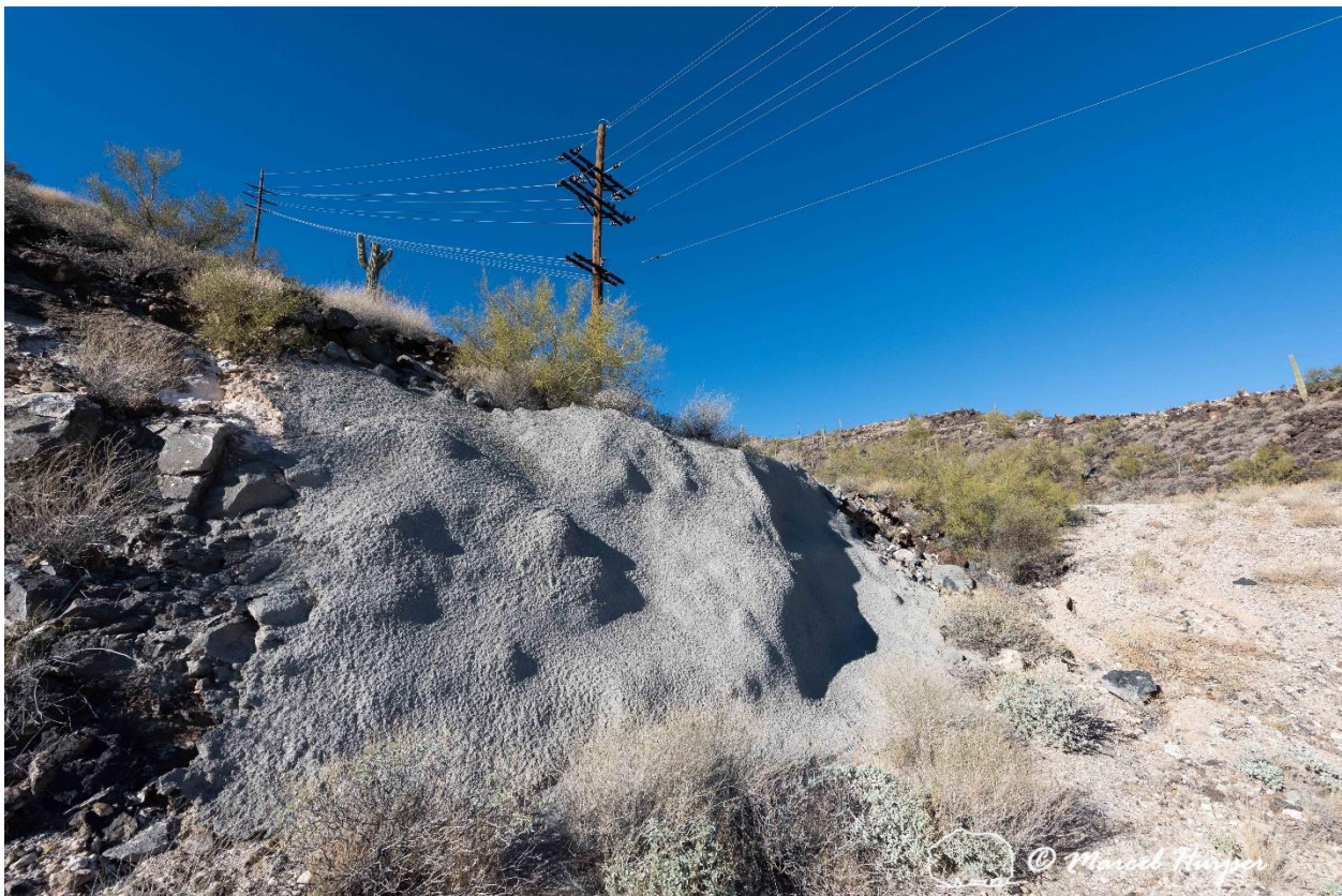
Shotcrete stabilizes a cut-slope along the road to Childs Mountain overlook (32°26'13.16"N 112°56'35.27"W).
