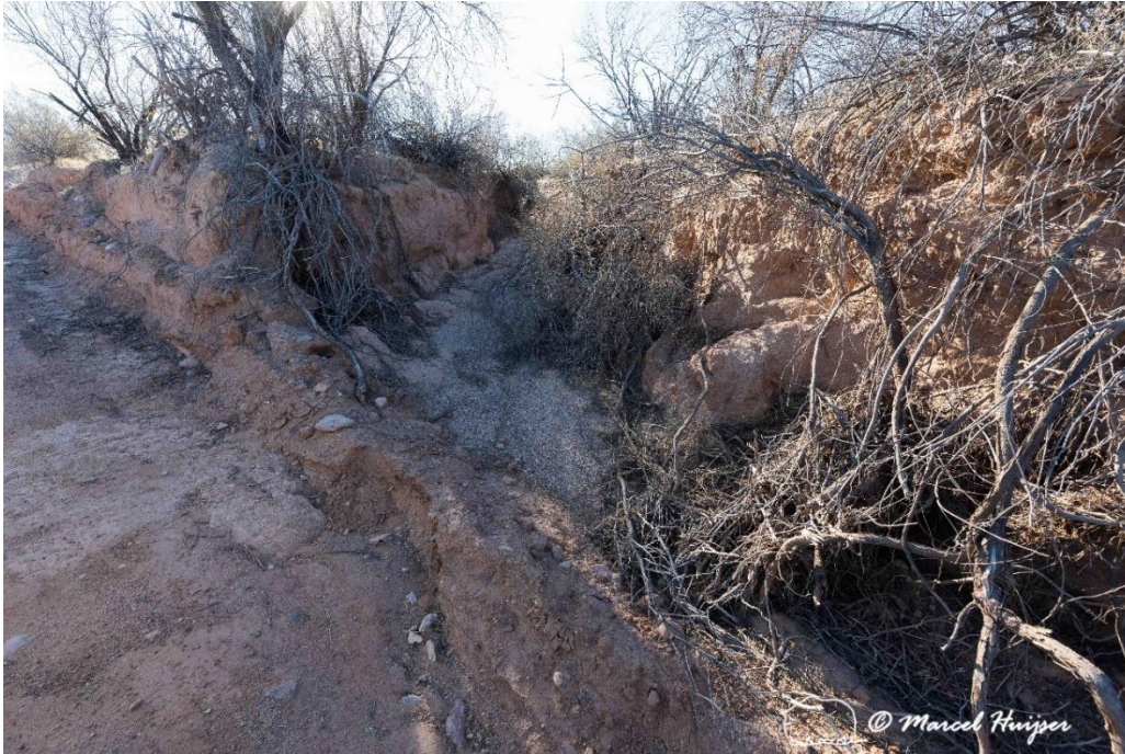
Deeply eroded side channel funneling water into incised road near Cuerda de Leña and Kuakatch wash. Organ Pipe Cactus National Monument, Arizona ( 32^{\circ}12'1.836'' N 112^{\circ}51'39.059'' W). The incised road and the side channel get wider over time, and the side channels eat further and further into the area adjacent to the road.
