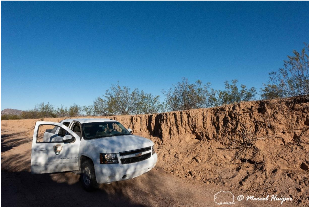
Deeply eroded and incised road (over 6 ft) near Cuerda de Leña and Kuakatch wash. Organ Pipe Cactus National Monument, Arizona (32°12'1.764" N 112°52'1.968" W).
