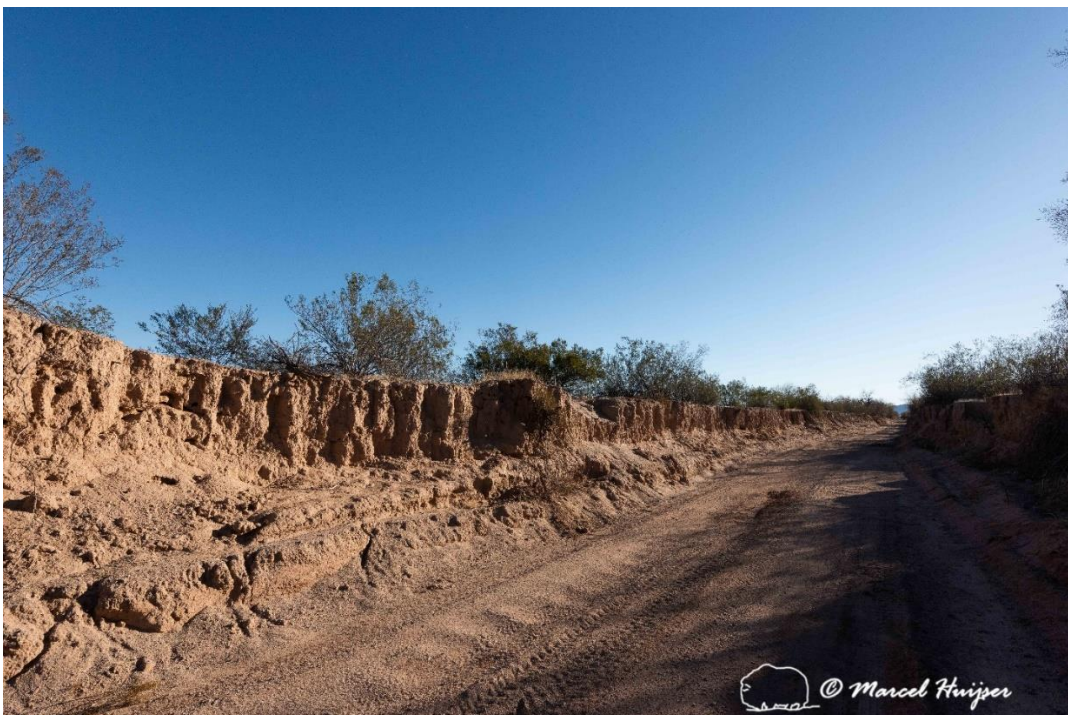
Deeply eroded and incised road (over 6 ft) near Cuerda de Leña and Kuakatch wash. Organ Pipe Cactus National Monument, Arizona (32°12'1.847" N 112°52'2.088" W).
