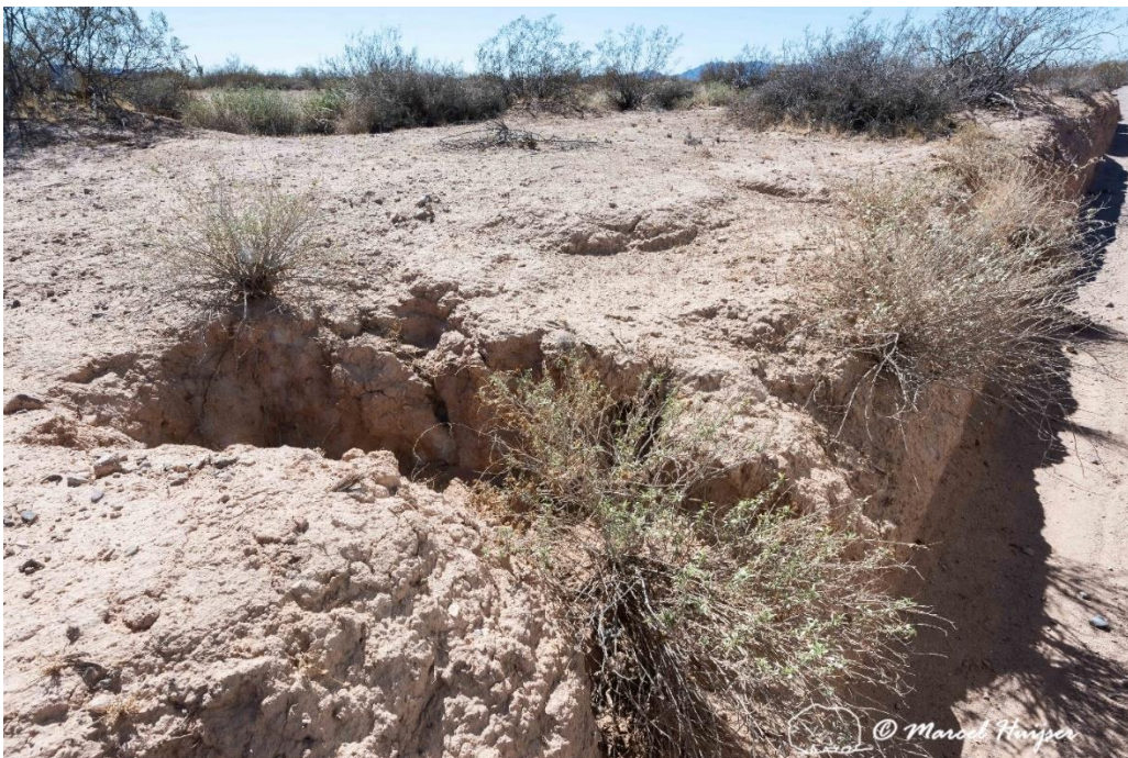
A side channel forms along heavily eroded and incised road, along Bates-Well road, Organ Pipe Cactus National Monument, Arizona ( 32^{\circ}8'58.097'' N 113^{\circ}2'6.245'' W). The side channel will progress further and further from the road, while also widening and deepening.
