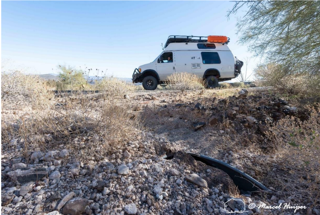
Clogged culvert under the road to the overlook, Childs Mountain, Cabeza Prieta National Wildlife Refuge, Arizona (32°26'9.14"N 112°56'32.67"W).
