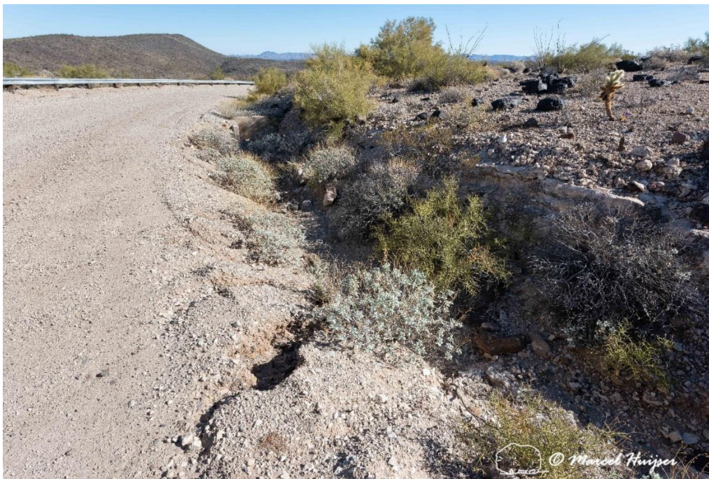
Erosion of the roadbed into the inboard ditch along the road to the Childs Mountain overlook (32°26'50.90"N 112°55'47.49"W).
