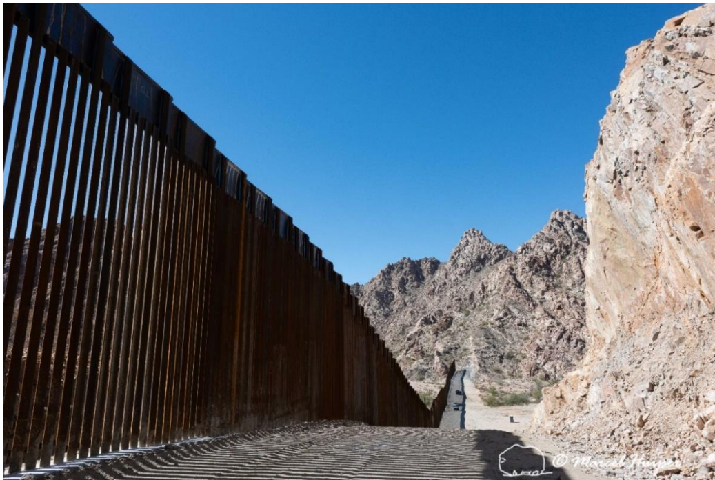
Border wall and road, south of Tule Well, at the southern end of the O-5 road, adjacent to Cabeza Prieta National Wildlife Refuge, Arizona. The Roosevelt Reservation is a 60 ft wide strip of federal land along the border that is not part of the refuge ( 32^{\circ}10'46.925'' N 113^{\circ}46'58.985'' W), but the activities and infrastructure along the border do impact the ecology of the adjacent refuge.
