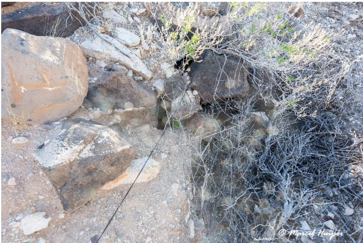
Clogged culvert under the road to the overlook, Childs Mountain, Cabeza Prieta National Wildlife Refuge, Arizona (32°26'13.70"N 112°56'48.50"W).
