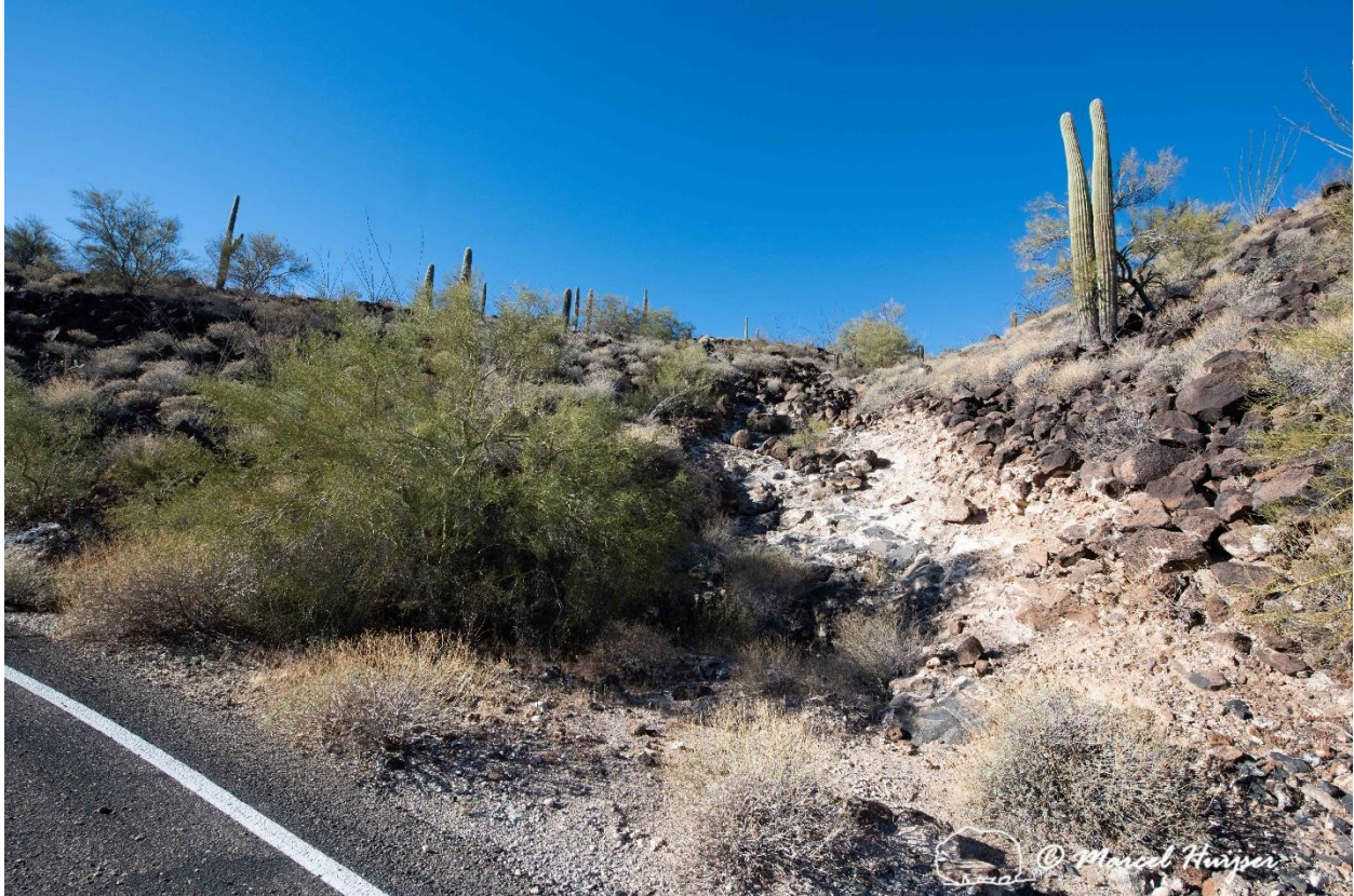
An erosion gully crosses the road to the Childs Mountain overlook (32°26'9.26"N 112°56'32.43"W).
