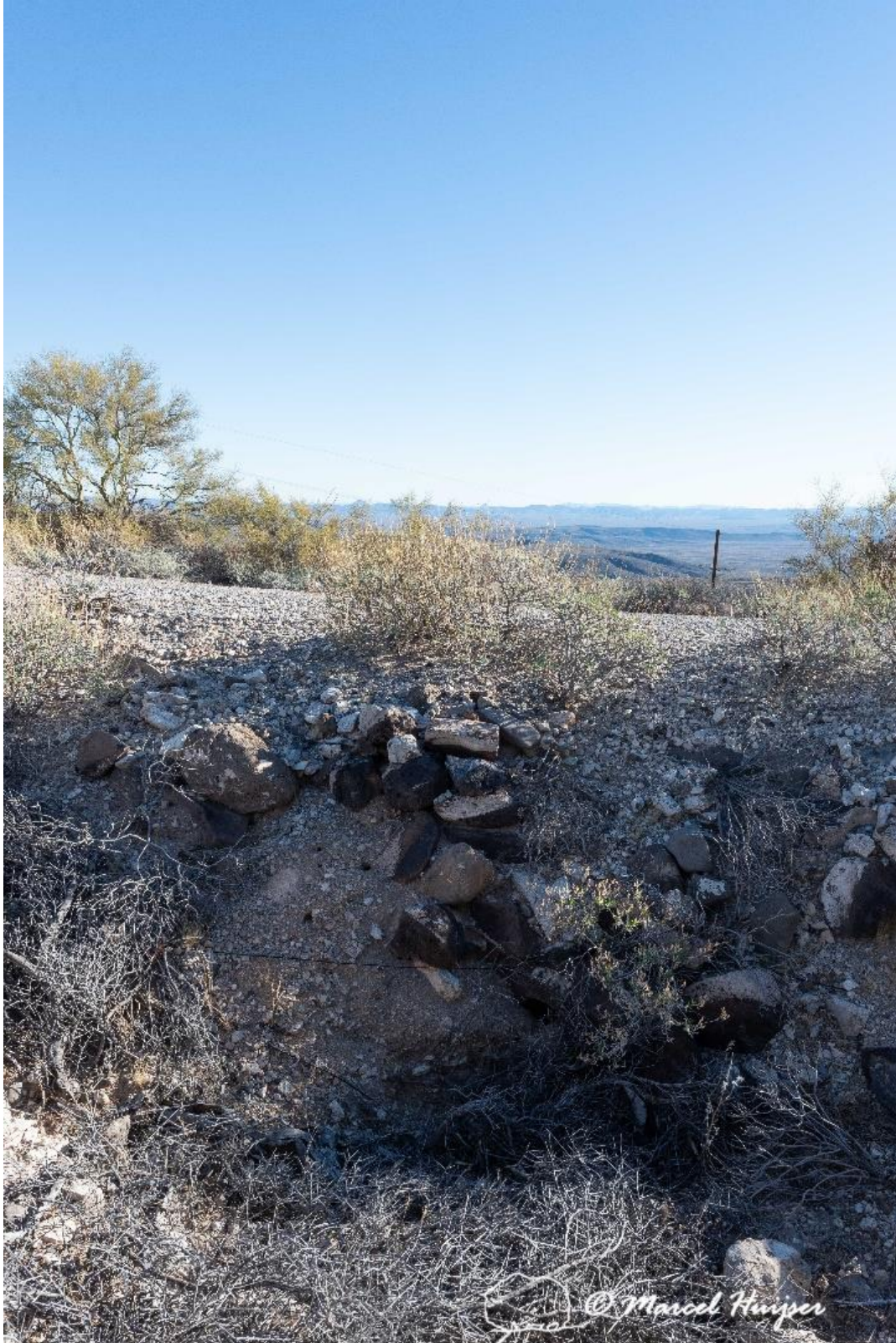
Clogged culvert under the road to the overlook, Childs Mountain, Cabeza Prieta National Wildlife Refuge, Arizona (32°26'13.85"N 112°56'48.79"W).
