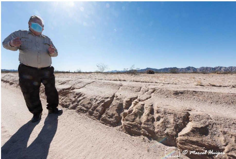
Berm with evidence of sheet flow entering the lower roadbed, primarily caused by grading, along a widened section of El Camino del Diablo, about 1.1 mile from the western boundary, Cabeza Prieta National Wildlife Refuge, Arizona ( 32^{\circ}16'32.286'' N 113^{\circ}56'36.048'' W). Ideally the sheet flow should continue on the other side of the road. Because the road is incised (because of a combination of grading and erosion), this can no longer happen. Instead the water concentrates on the road until it breaks through the berm on the other side and forms a small or large desert wash. Other areas on the "downslope side" of the road no longer receive sheet flow.
