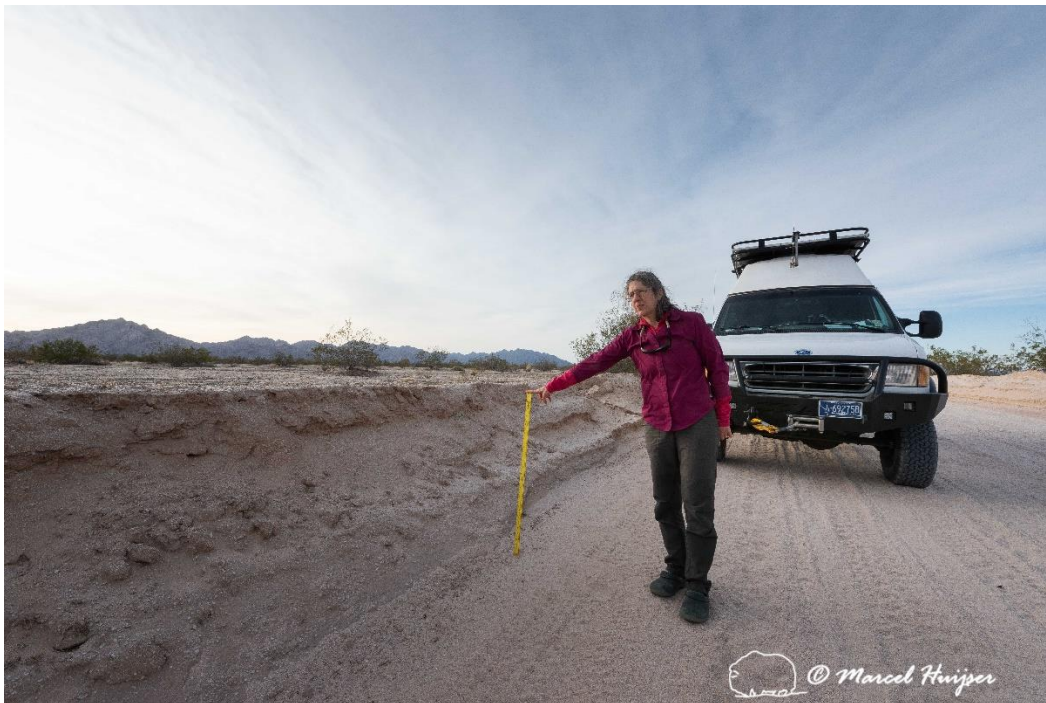
Berm (over 3 ft tall), primarily caused by erosion, but initiated by grading, along a widened section of El Camino del Diablo, about 10.3 miles north of Tinajas Altas, Barry M. Goldwater Range West (BMGR-W), Arizona ( 32^{\circ}27'14.837'' N 114^{\circ}5'57.467'' W).
