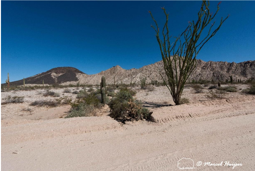
Berm (1-2 ft tall), primarily caused by grading, along a widened section of El Camino del Diablo, about 5.5 miles east of western boundary, Cabeza Prieta National Wildlife Refuge, Arizona ( 32^{\circ}15'4.506'' N 113^{\circ}52'29.273'' W).
