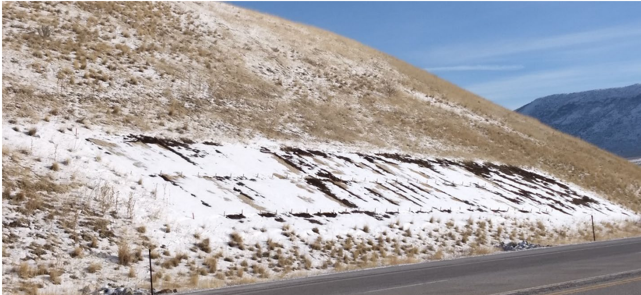
Figure 15. Block along US-30 in February 2019, showing the ECB were protected by snow from strong winds during the 2018-2019 winter season.
