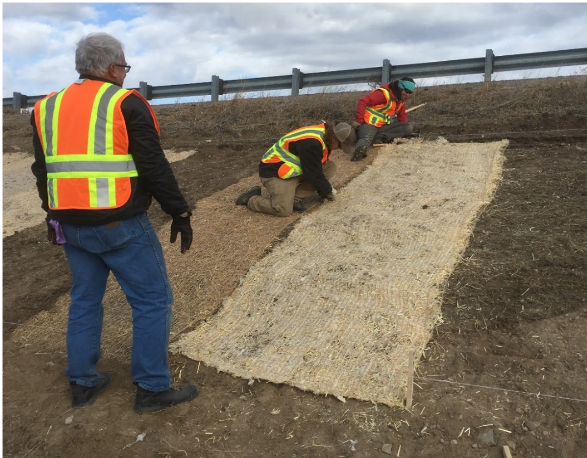
Figure 11. Researchers installing ECB blankets with sod staples. The ECB was placed over a plot that was broadcast seeded at the I-86 highway roadside test site.
