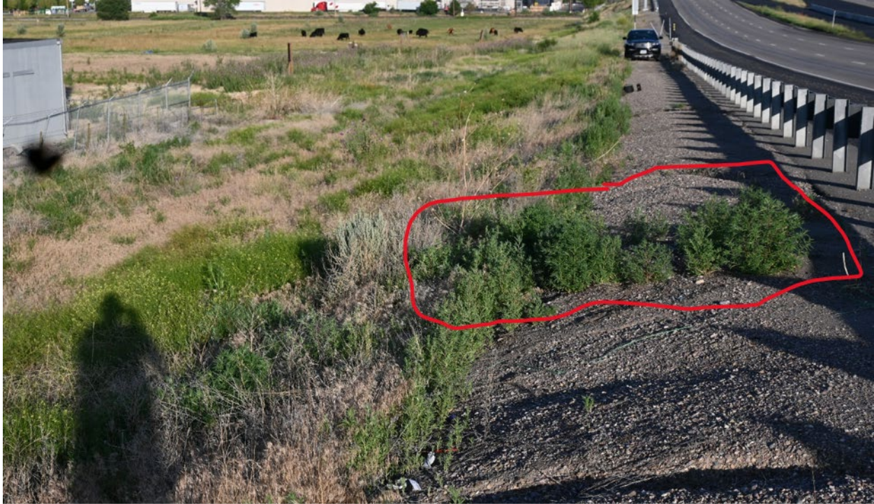
Figure 16. I-86 experimental site in July 2020 after the second year of plant growth, looking west. Red circle is location of erosion caused by unmitigated surface runoff where plot construction was avoided.
