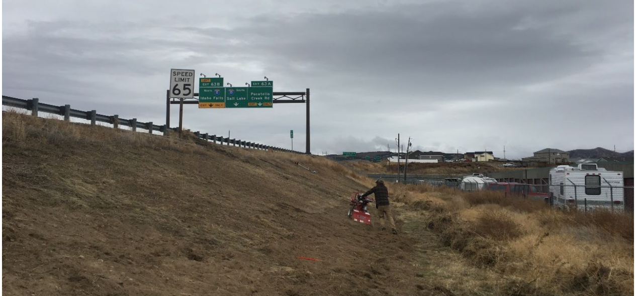
Figure 9. Researcher roto-tilling the soil along I-86 after surface vegetation has been cleared.
