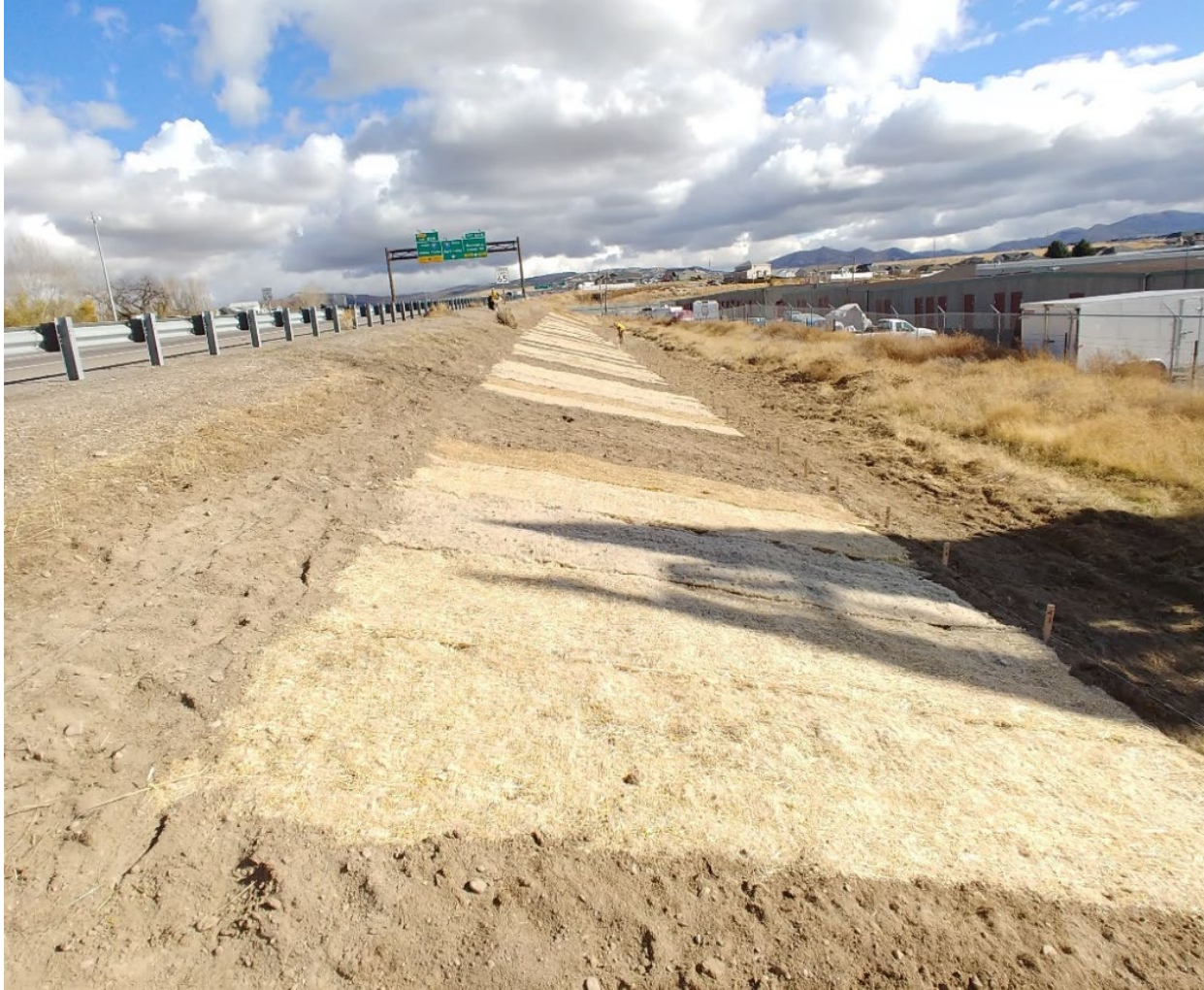
Figure 12. ECBs and bare control experimental plots after all the treatment repetitions have been installed along I-86.
