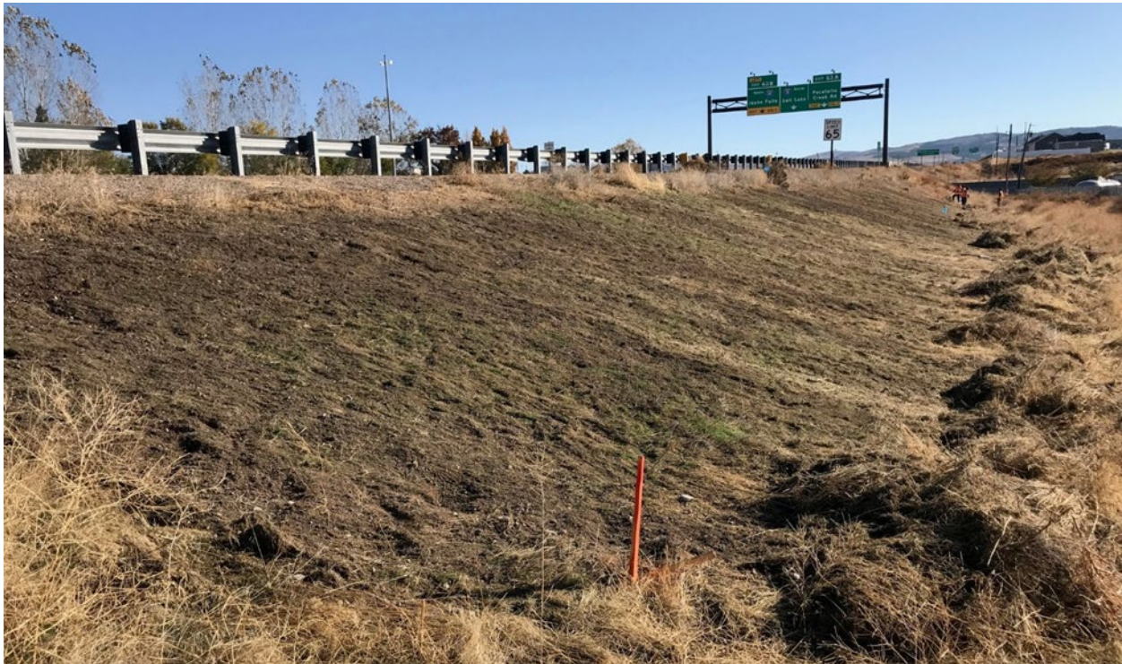
Figure 8. The I-86 plot cleared of surface vegetation, prior to installing experimental plots.
