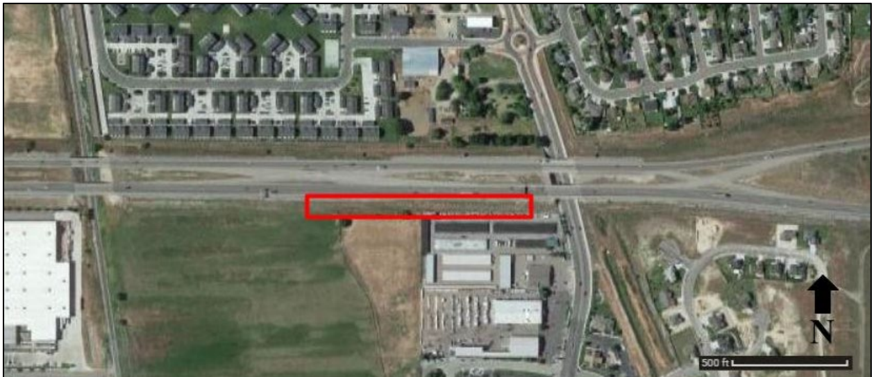
Figure 4. Aerial view of experimental block, outlined in red, along I-86 near Highline Road in Chubbuck, ID.
