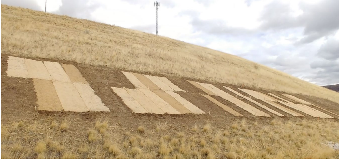
Figure 13. ECB after all the repetitions have been installed along US-30.
