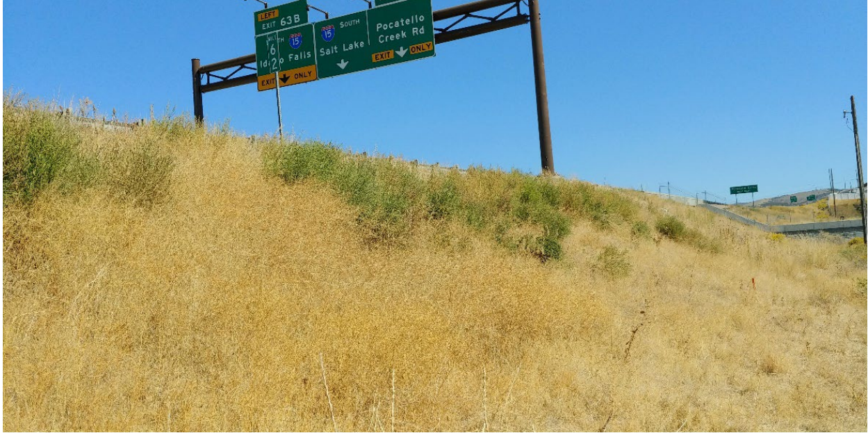
Figure 5. Photo of pre-experiment vegetation along I-86 before constructing experimental plots.
