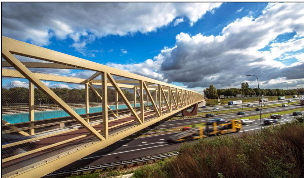
Figure 14: Hybrid bridge with FRP decking in Utrecht, the Netherlands (FiberCore Europe, 2012).
