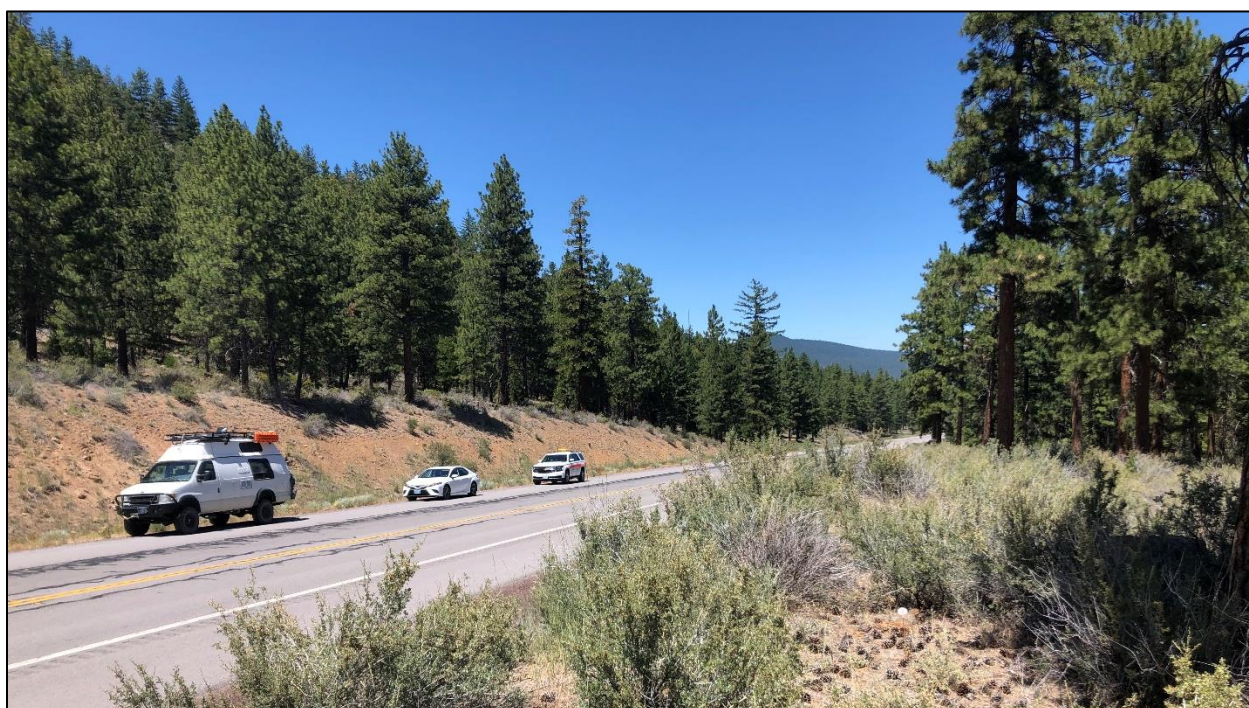
Figure 67: Below grade road alignment at Mud Lake B looking north-northwest.
