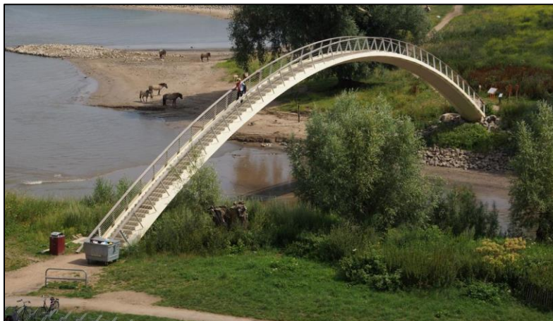
Figure 16: Arched uni-mold bridge in Nijmegen, the Netherlands (Structurae, 2014).
