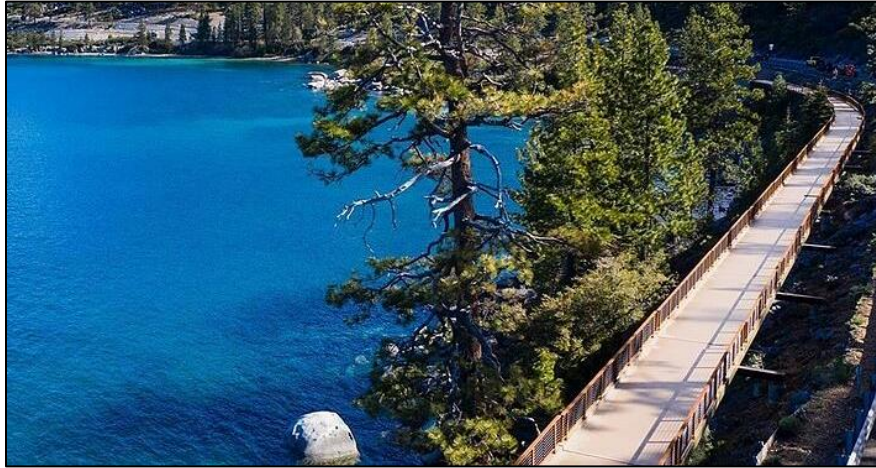
Figure 13: Hybrid walkway with FRP decking and steel supports near Lake Tahoe, California (Creative Composites Group, 2019).
