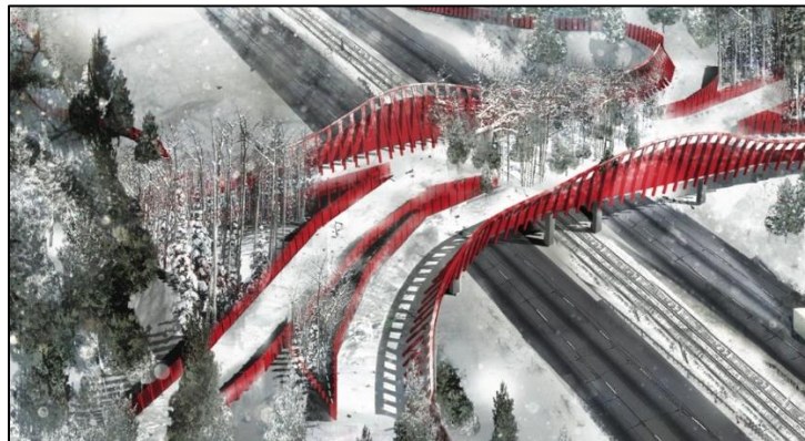
Figure 18: Guardian Bridge Rapid Construction's design of a wildlife overpass for a design competition over Interstate Highway 70 in Colorado (ARC Solutions, 2010).
