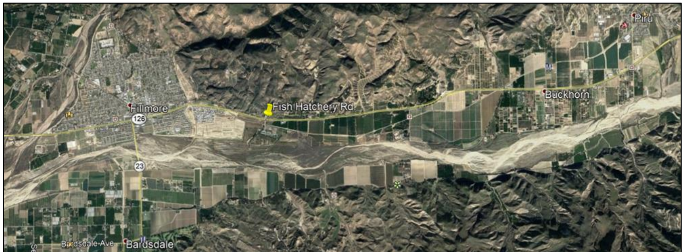
Figure 49: Proposed mitigation location along SR-126 in Ventura County, California.
