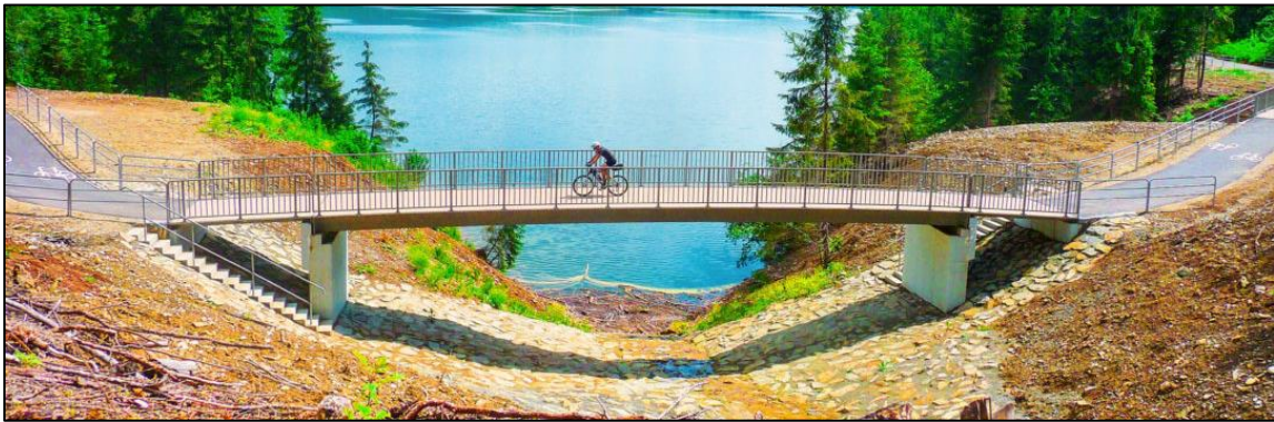
Figure 15: Example of uni-mold pedestrian bridge built around Lake Czorsztyn, Poland (FiberCore Europe, 2019a)
