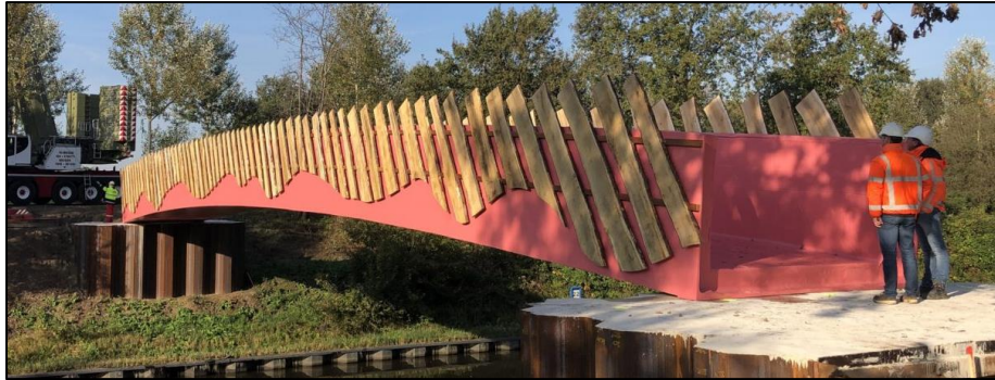
Figure 9: FRP ecoduct near Eindhoven, The Netherlands spans 36 m (118 ft) and is 3.5 m (11.5 ft) wide (FiberCore Europe, 2019b).
