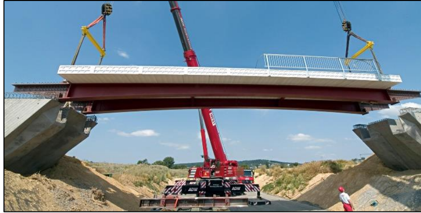
Figure 6: A hybrid traffic bridge over B3 highway in Germany (Fiberline Composites, 2006).
