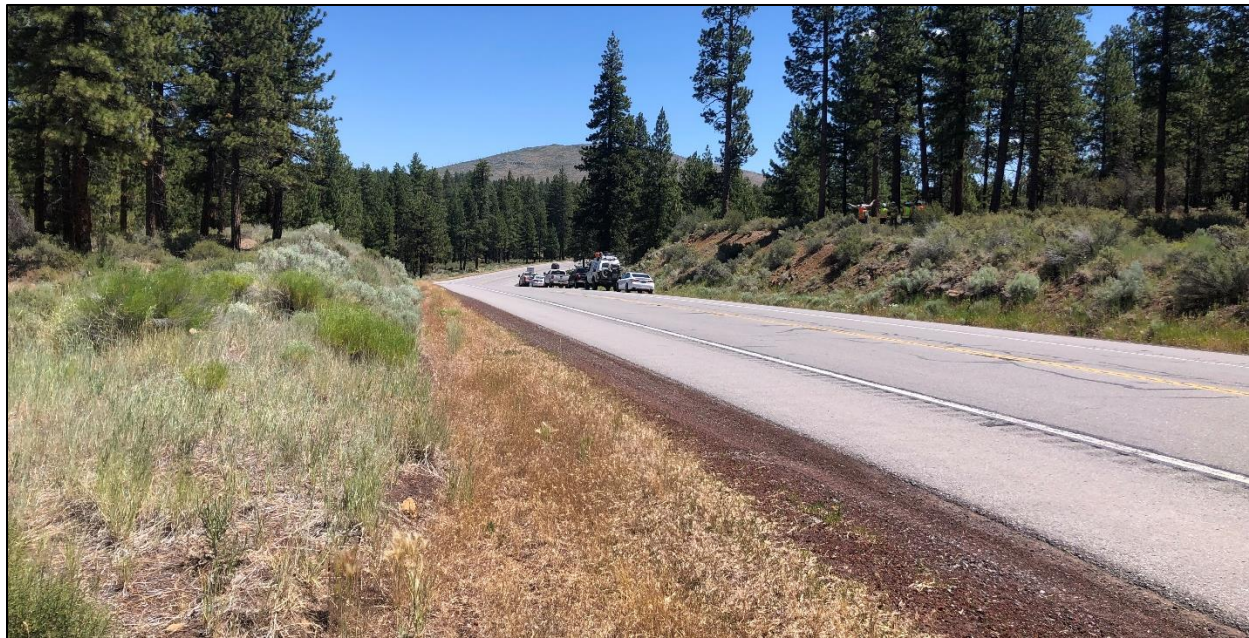
Figure 60: The downhill, below grade, elevation change at the Horsethief Creek site looking east.
