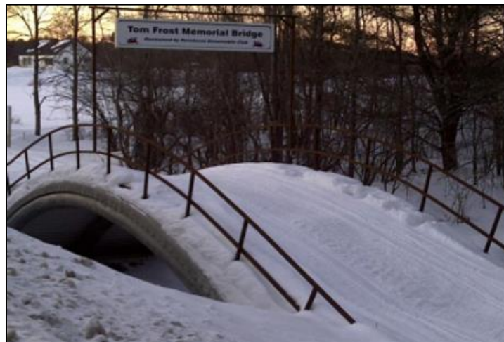
Figure 12: A hybrid CFFT pedestrian snowmobile bridge, Hermon, Maine (Advanced Infrastructure Technologies, 2010).
