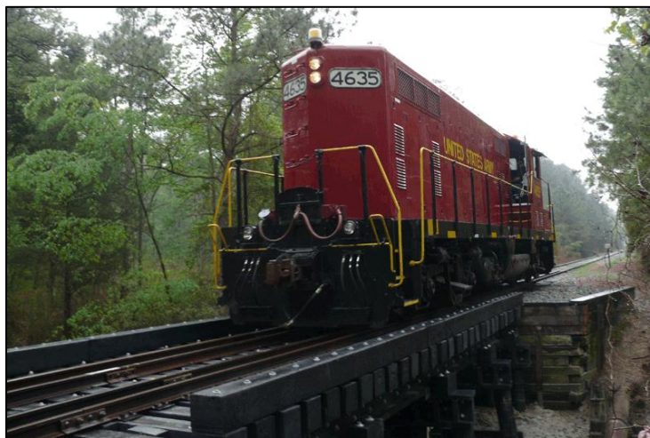
Figure 23: Pultrusion-style train bridge built from recycled plastic (Chino, 2011).
