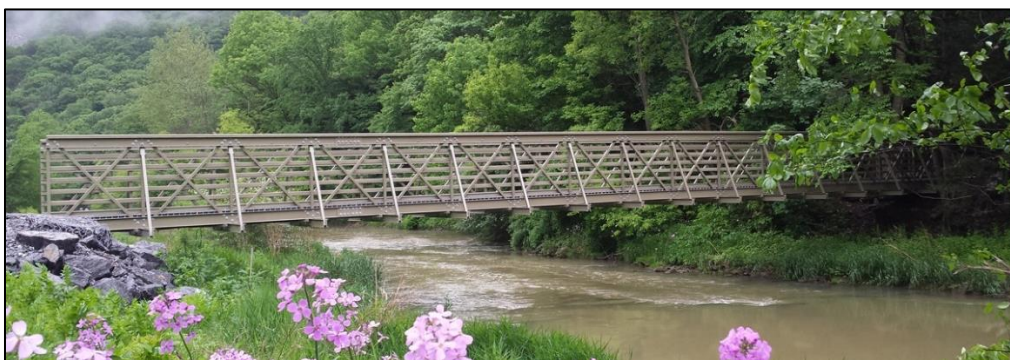
Figure 11: FRP Pultrusion pedestrian bridge built by Creative Pultrusions (Griffith, 2018).
