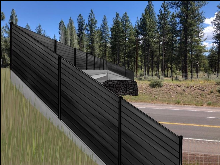
Figure 39: Recycled-plastic sound and light barrier installed on top of soil-retaining concrete curb.
