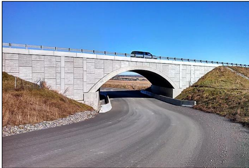
Figure 21: CFFT bridge built by AIT in Augusta, Maine.
