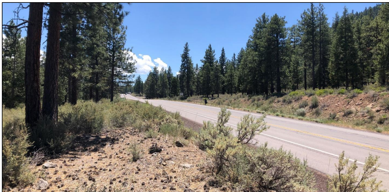
Figure 66: Below grade road alignment at Mud Lake B looking south-southwest.
