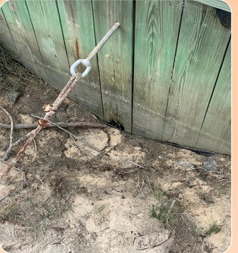
Erosion behind bulkhead due to failing sheet pile
