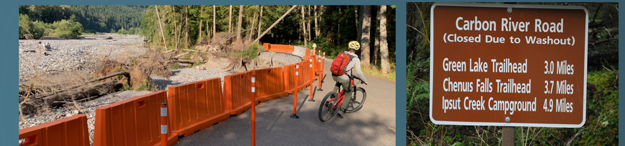
Images: Carbon River Road damages. (source: Pat McMahon)
