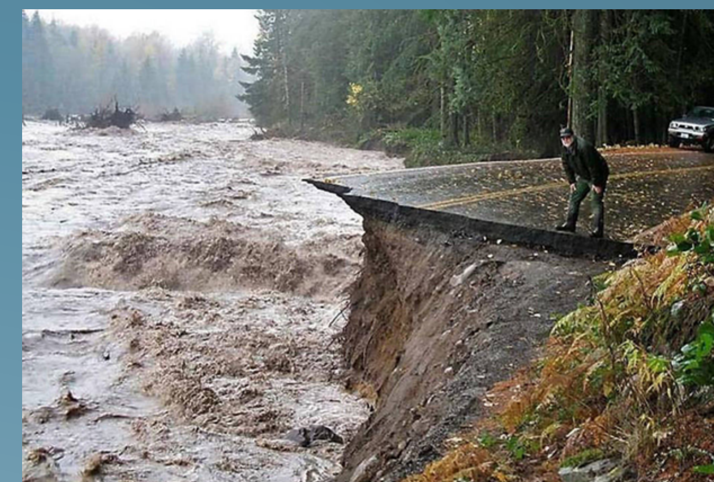
Image: 2006 washout of Nisqually Paradise road and Sunshine Point Campground. (source: The Chronicle)
