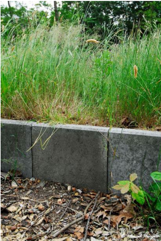
Figure 66. A “barrier wall” (concrete) integrated into the roadbed for common toads ( Bufo bufo ), Deelenseweg, between Hoenderloo and Arnhem, Gelderland, The Netherlands.
