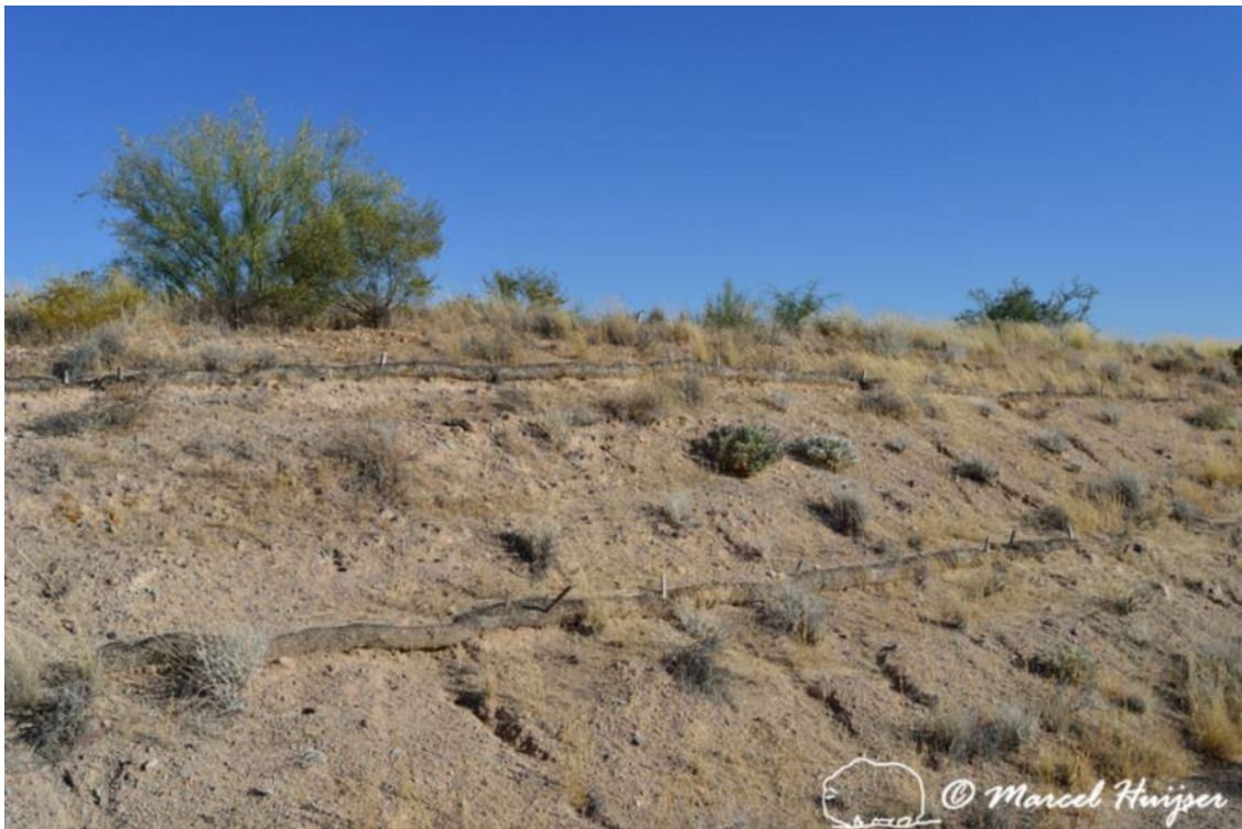
Figure 56. Straw fiber rolls to control erosion on a road cut, Hwy 87, Arizona, USA.
