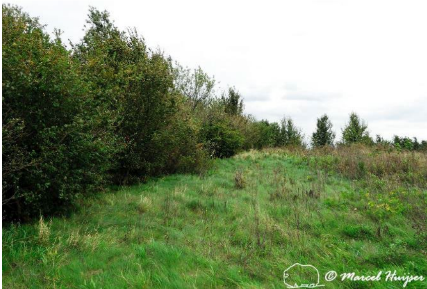
Figure 78. Cover, grassland, and edge habitat on top of multifunctional overpass (wildlife and farm road, about 100 m wide), across A4 motorway, Parndorf, Austria. The overpass is designed for farmers, agricultural machinery, hunters and wildlife including roe deer ( Capreolus capreolus ) and European hare ( Lepus europaeus ).
