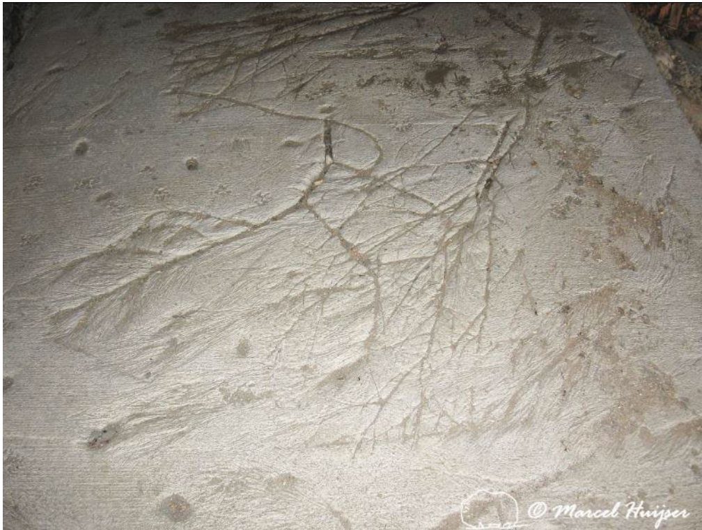
Figure 94. Imprints in concrete surface in wildlife underpass to make it less slippery for wildlife, US Hwy 93 S, Bitterroot Valley, Montana, USA.
