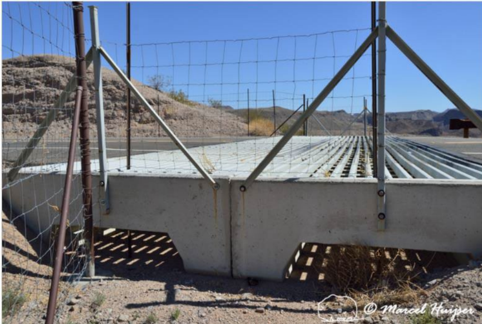
Figure 36. Combined drainage and escape for small animals under wildlife guard, Arizona, USA. The openings on the side allow for drainage under the culvert. The openings also allow invertebrates, amphibians, reptiles, small mammals and other species that may fall in between the metal bars to escape.
