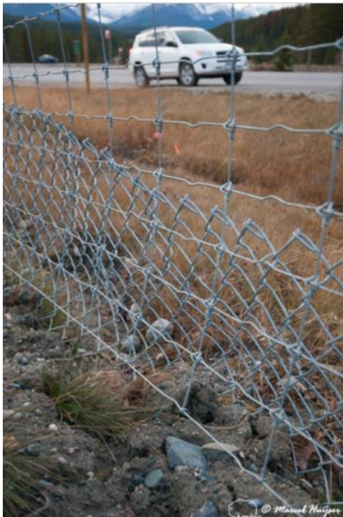
Figure 10. Wildlife fence and dig barrier (“buried fence” or “apron”), Trans-Canada Highway, Banff National Park, Alberta, Canada. The dig barrier in the soil angles (45°) towards the safe side or habitat side; it angles away from the fence and the road on the other side (Clevenger and Huijser 2011). The dig barrier keeps animals from digging under the fence. The dig barrier may consist of a 4-5 ft (1.0-1.2 m) wide galvanized chain-link fence that is attached to the bottom of the actual fence. The buried fence should extend approximately 3.5 ft (1.1 m) under the ground (Clevenger and Huijser 2011).
