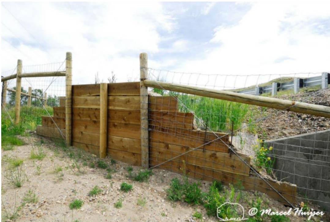
Figure 48. Wildlife fence and jump-out with a face consisting of wooden planks, near Havre, Montana, USA.
