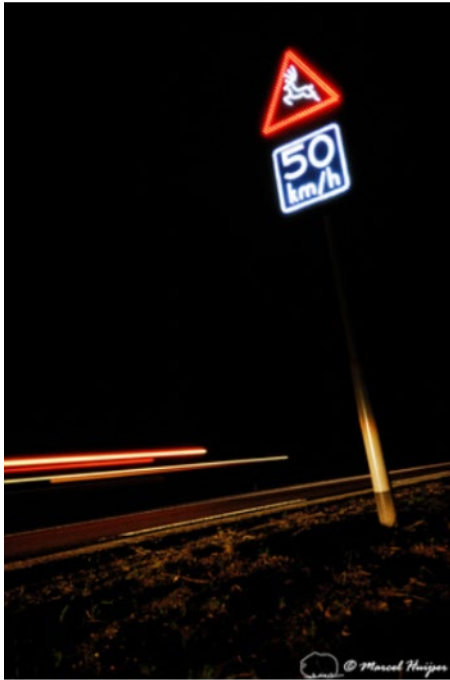
Figure 57. Animal detection system at night with reduced advisory speed limit in association with a detection, Harderwijk, The Netherlands. Note that if there is no wildlife detected, the LED sign has no message at all (it is black).
