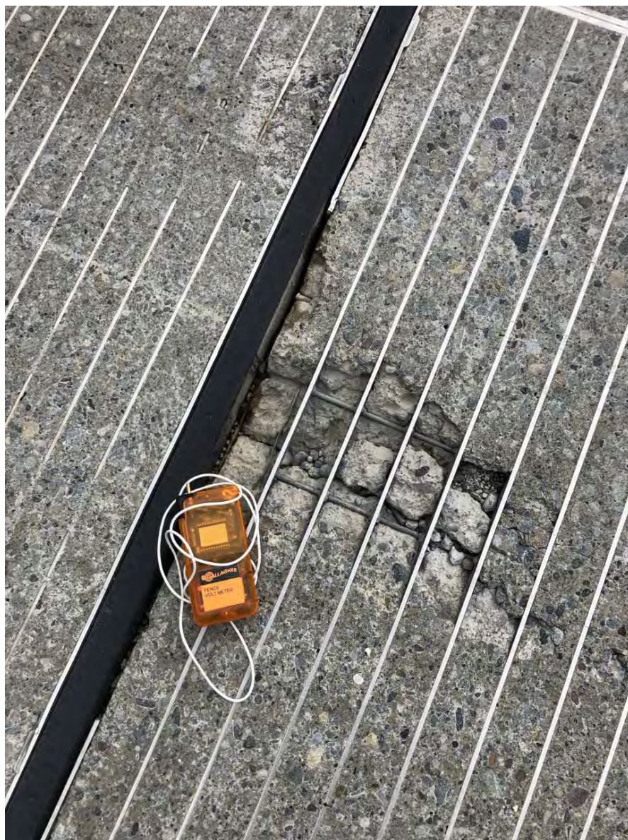
Figure 37: Crumbling concrete at the western electrified barrier, presumably associated with a change in slope after the bridge abutment settled (image Samantha Getty).
