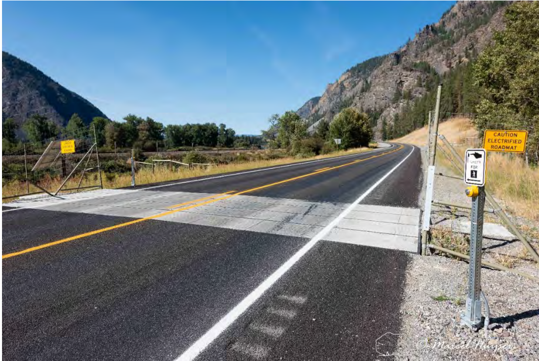
Figure 33: The electrified barrier at the east fence-end.
