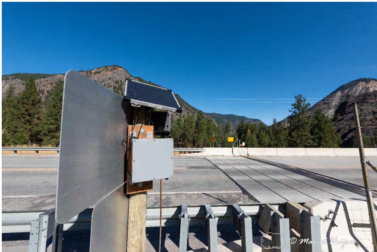
Figure 35: The camera, battery box and solar panel installed on a sign post behind the sign at the western electrified barrier.
