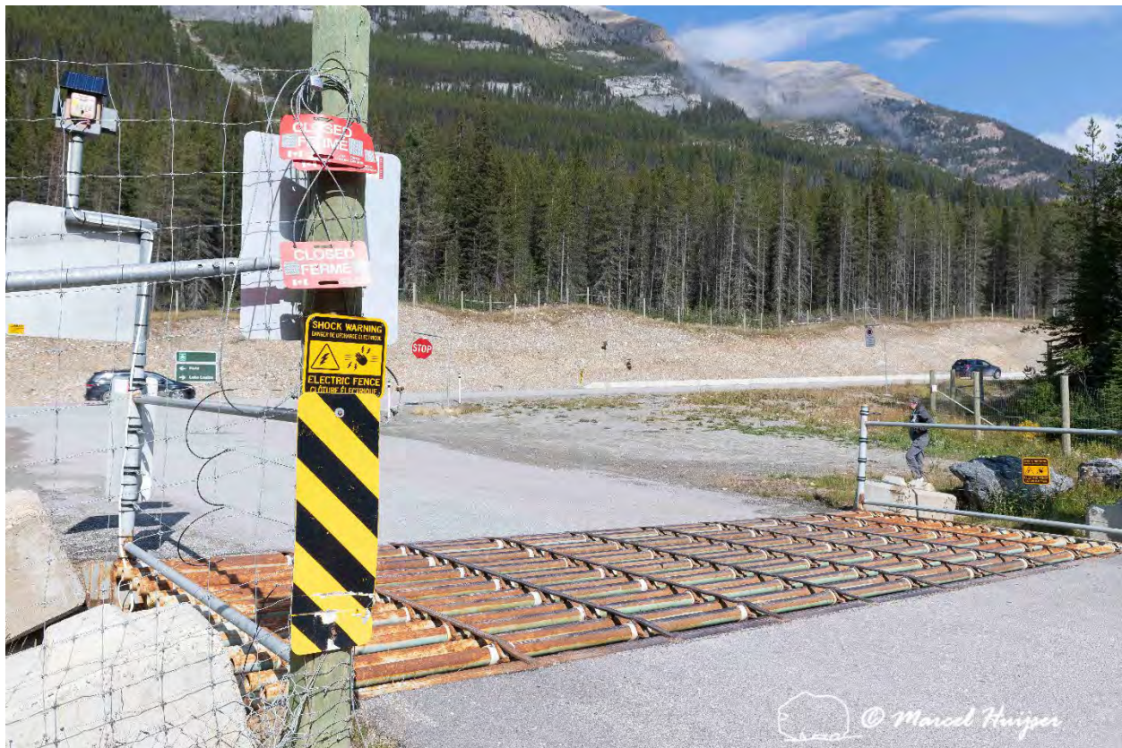
Figure 29: Electrified barrier, Lake O'Hara exit, Yoho National Park, Canada.
