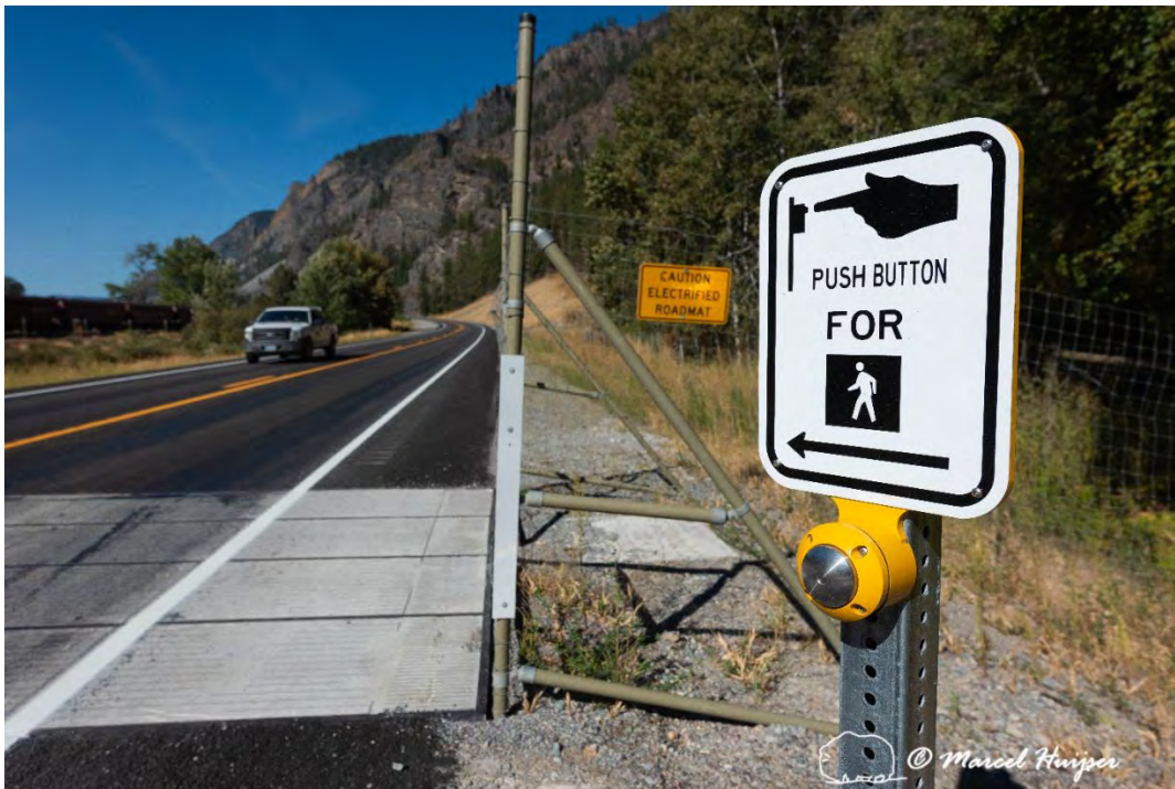
Figure 34: One of the push buttons for pedestrians at the electrified barrier at the east fence-end. There are 2 push buttons; one for each travel direction.
