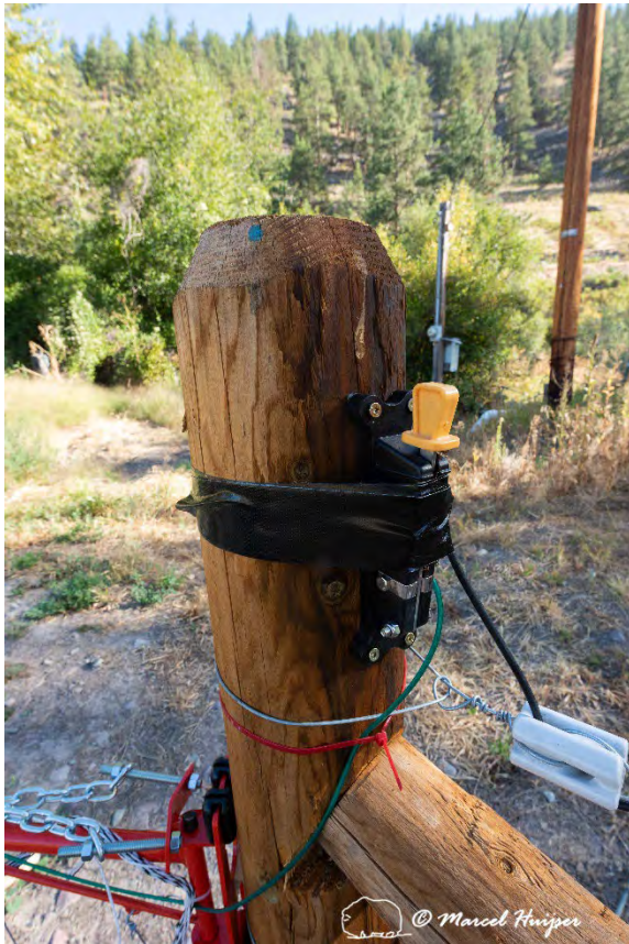
Figure 22: Switch at a bump gate taped in the permanently “on” position. Also note the adjustment bolts and nuts for the chain (lower left in image) that allows for the alignment of the horizontal pole.
