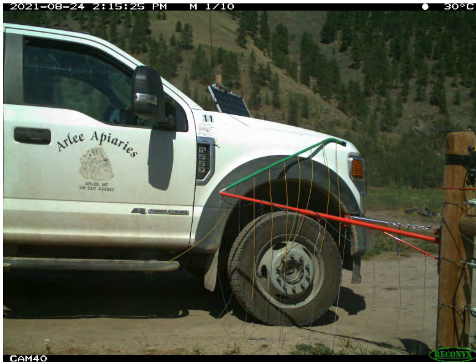
Figure 23: Broken horizontal pole of a bump gate because of a vehicle passing through.
