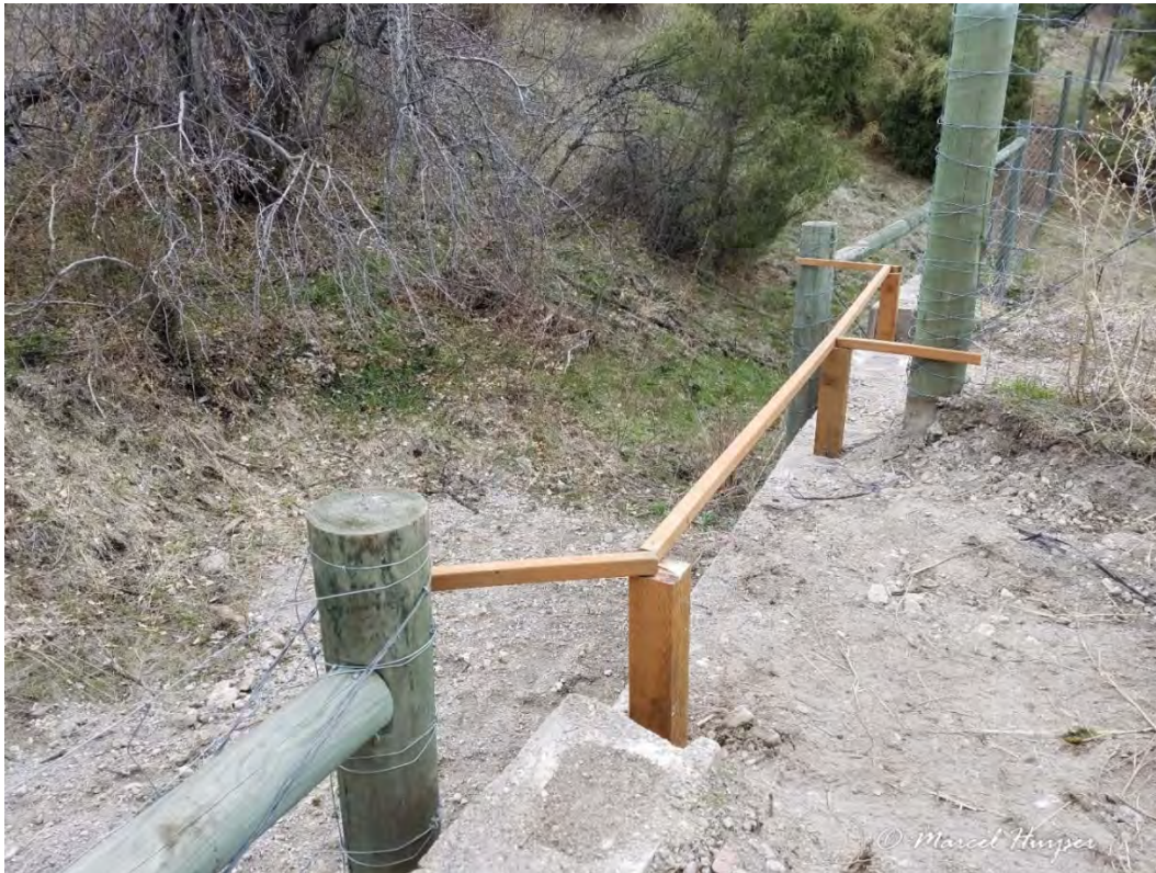
Figure 5: The prototype for the “bar” made from “2x2” inch and “4x4” inch treated lumber.
