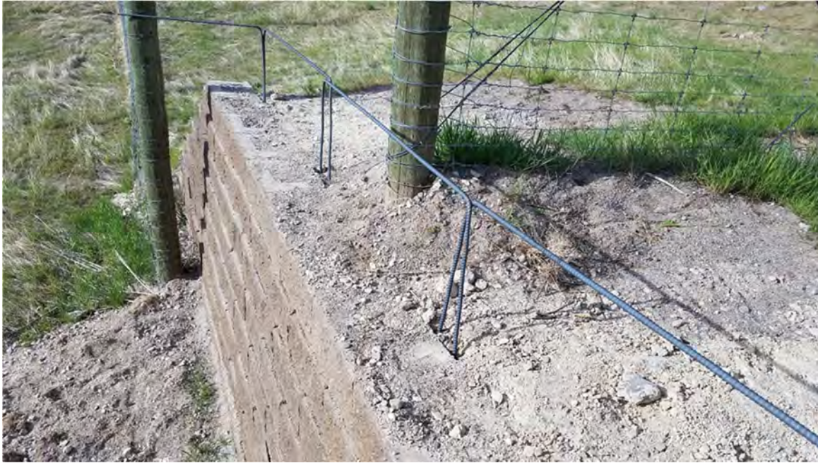
Figure 11: The rebar had a minimum setback of 12 inches (30 cm) as the legs had to be positioned behind the concrete blocks of the face of the jump-out.
