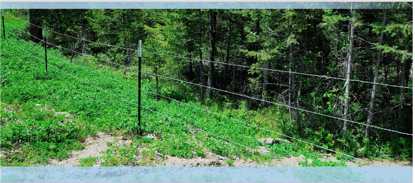
Figure 28: Wildlife friendly livestock fence with smooth top and bottom wires, Montana, USA (Marcel Huijser).
