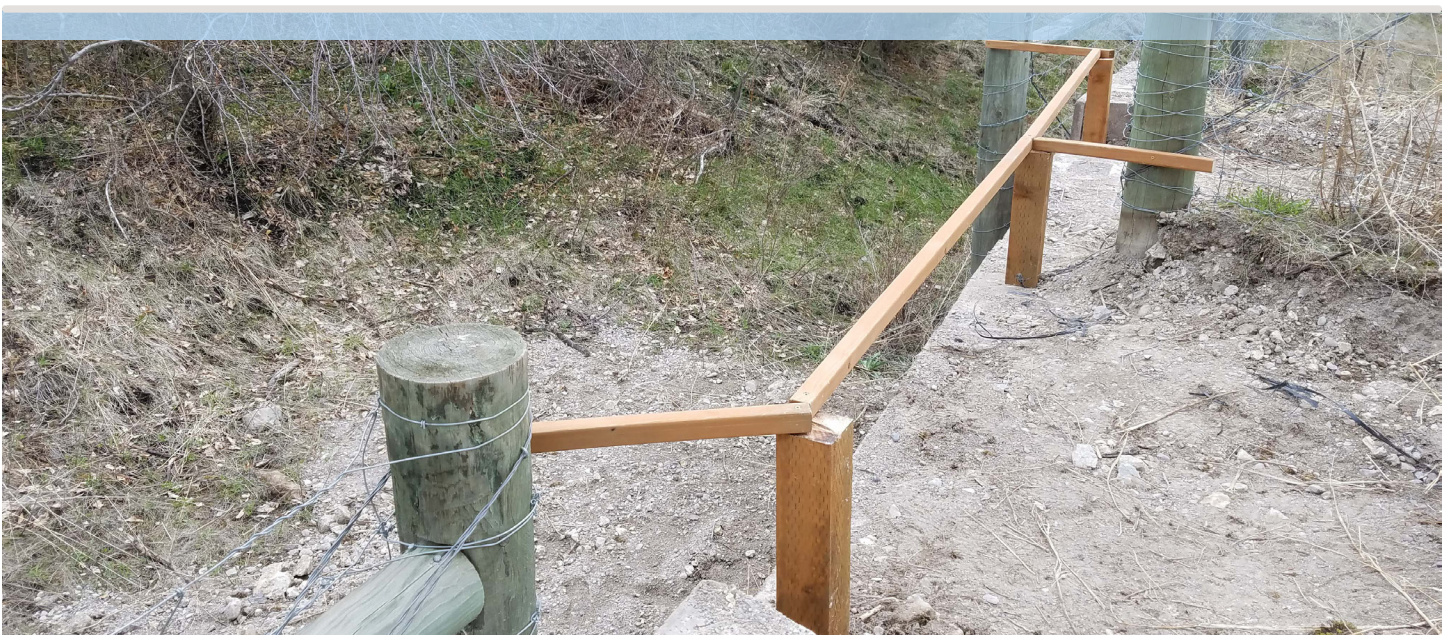
Figure 24: A jump-out that is modified with a 2 in (5 cm) by 2 in (5 cm) bar for the design experiment (Marcel Huijser).
