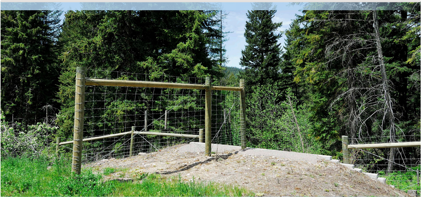
Figure 23: A view of a jump-out on the highway side of the fencing with a perpendicular fence that is designed to direct animals following the exclusionary fence to use the jump out (Marcel Huijser).
