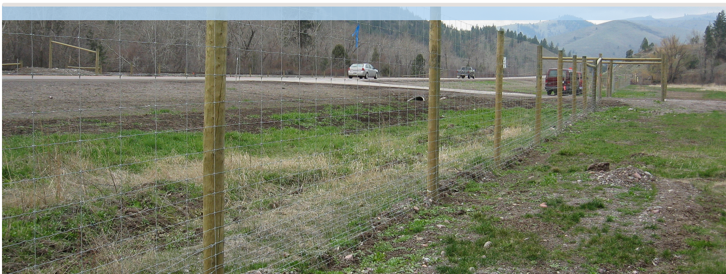
Figure 27: Typical large ungulate fence in North America, 8 ft tall, wooden posts and mesh-wire fence material, US Hwy 93 North, Montana, USA. Note that there is a dig barrier attached to the main fence material (e.g. for canids) (Marcel Huijser).
