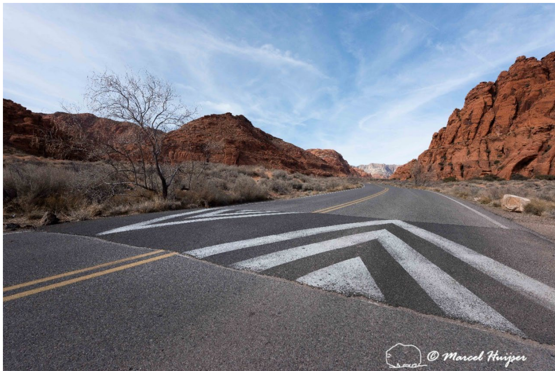
Speed bump to control speed, primarily for Mojave desert tortoise, St. George, Utah.
