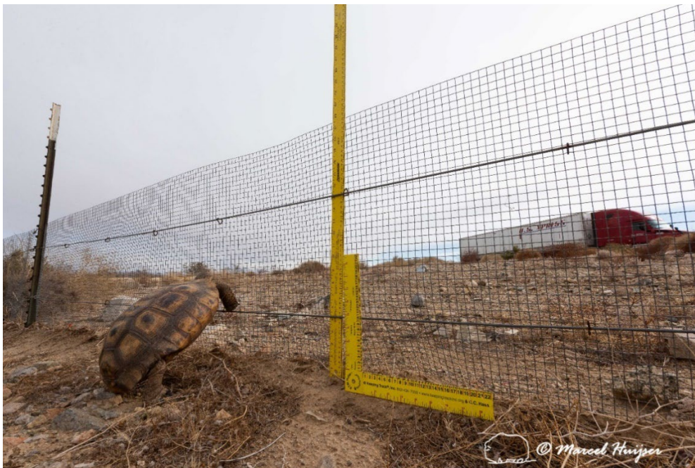
Mojave desert tortoise fence (about 21.5 inches tall, mesh size about 1x1 cm), I-15 near Barstow, California. The small mesh size may pose a greater risk to small animal species (lizards, snakes) getting stuck and dying. Small mesh sizes are also more likely to catch sediment. Note that there is no smooth wire at the very top of the fence, making the fence less rigid.
