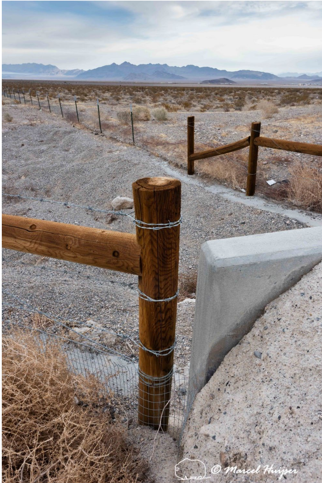
Mojave desert tortoise fencing connected to a culvert, US Hwy 95 (MP 121.6 NB) near Indian Springs, Nevada. Note concrete access paths for Mojave desert tortoises constructed along the fence.
