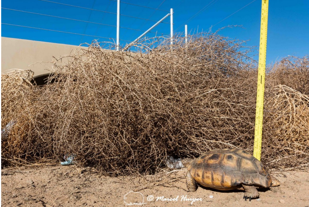
Tumbleweeds block Mojave desert tortoises approaching or leaving culverts, Hwy 58 near Kramer Junction, California.
