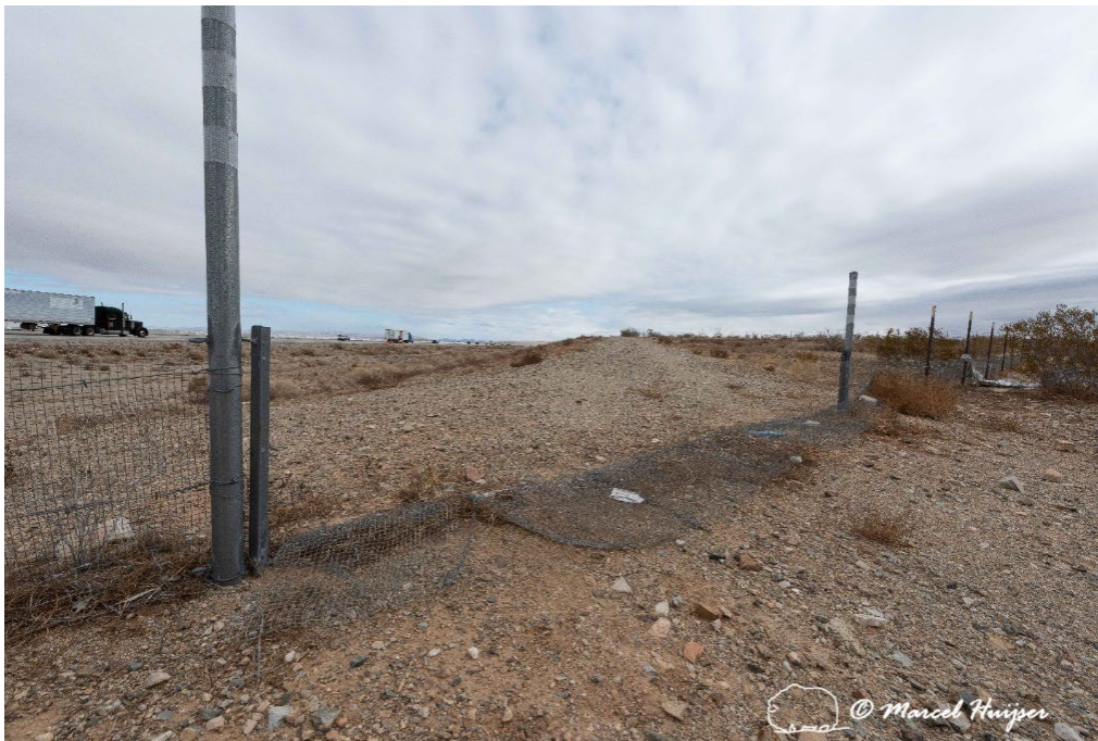
Flattened and destroyed gate at a vehicle access point associated with a Mojave desert tortoise fence, I-15 near Barstow, California. Here the fence has, or had, a gate for a dirt road, but the fence was flattened by vehicles. This suggests that gates that require people to get out of the vehicles to open them are not always effective and may result in a gap in the fence, allowing Mojave desert tortoises to access the highway.
