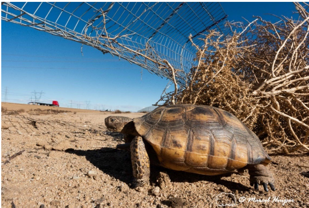
Gap under a gate associated with Mojave desert tortoise exclusion fencing, Hwy 58 near Kramer Junction, California. The gate does not have a buried component, and it had enough flex to result in permanent openings, partially as a result of tumbleweeds being blown against the fence.
