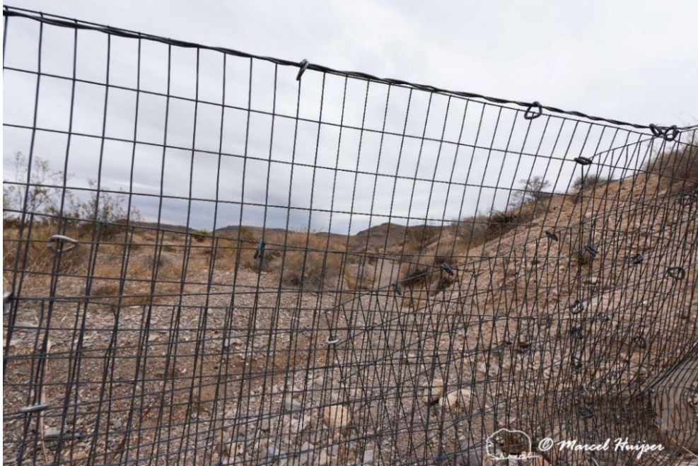
Detail of Mojave desert tortoise fencing, US Hwy 93 (MP 58 NB) near Overton, Nevada. Because of the change in slope (higher bank towards the right), the fence material was cut and installed in multiple overlapping segments.
