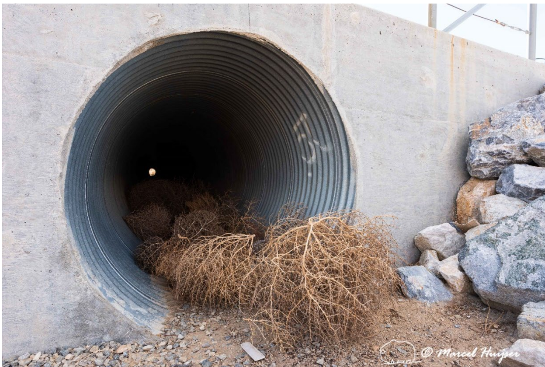
Culvert primarily constructed for hydrology, but the culvert may also allow for passage by Mojave desert tortoises I-15 near Barstow, California. However, this culvert is blocked by tumbleweed.
