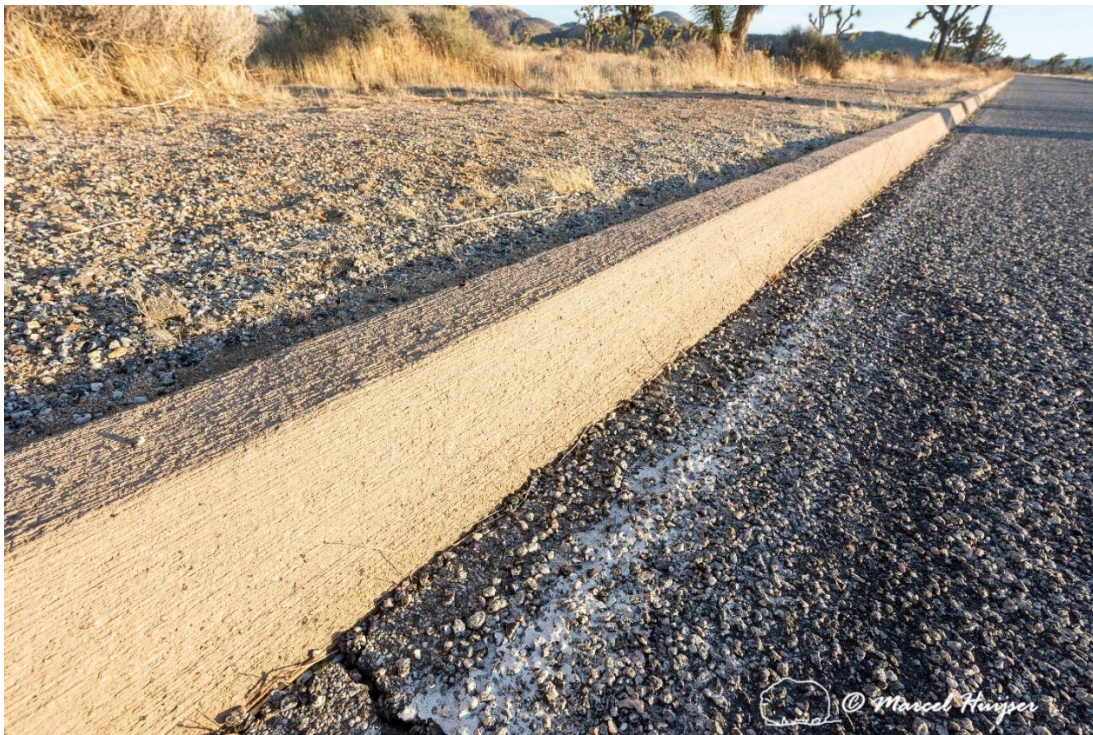
Curb to keep vehicles from leaving the pavement and parking along the roadside, Joshua Tree National Park, California. Denying vehicles access to the road shoulder can be combined with habitat restoration. The rough surface of the curb is to potentially allow Mojave desert tortoises to escape from the road.
