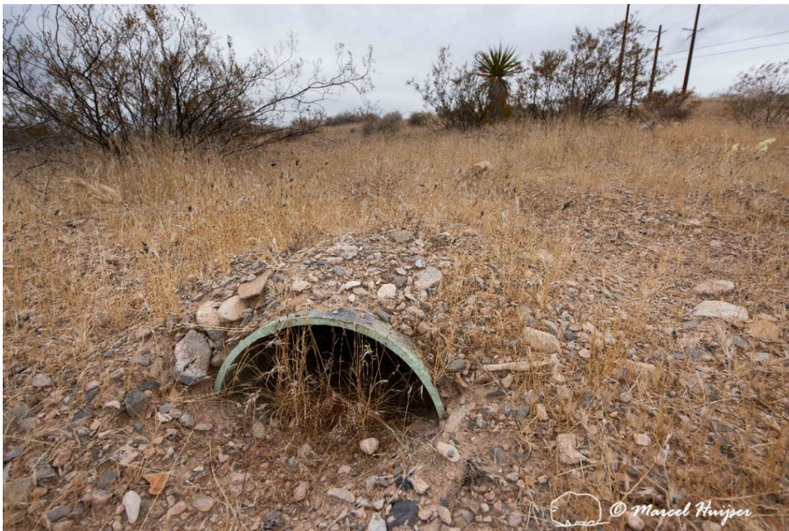
Artificial shade structure for Mojave desert tortoises, along US Hwy 93 (MP 58 NB) near Overton, Nevada.
