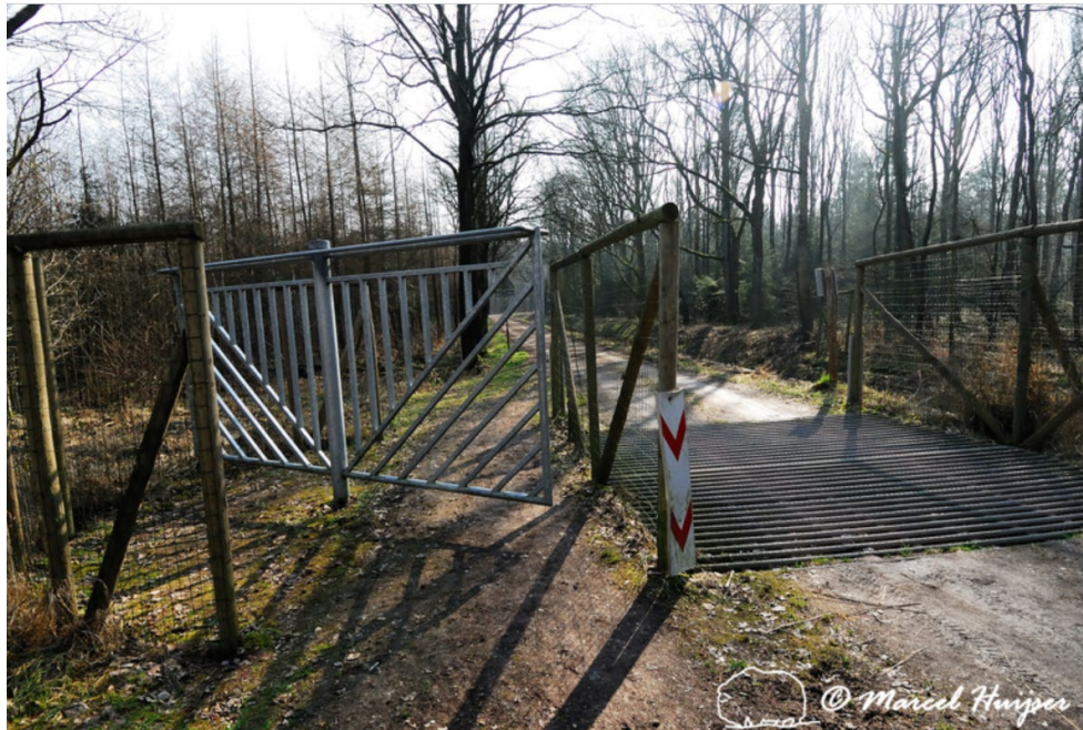
Horse swing gate, Heugterdijk, Weerterbos, near Maarheze, The Netherlands. The center of the metal swing gate is set at an angle so that gravity automatically brings the metal gate in line with the fence. Here the gate is in the process of closing.
