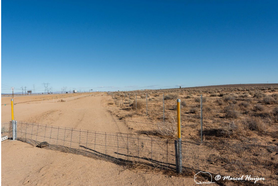
A gate associated with Mojave desert tortoise exclusion fencing, Hwy 58 near Kramer Junction, California. Note that the design of this gate resulted in gaps which affected its function as a barrier to Mojave desert tortoises (see images below).
