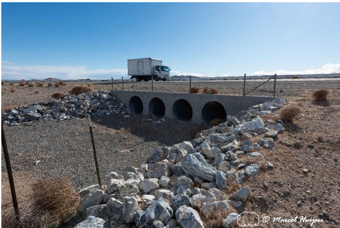
Mojave desert tortoise fencing leading up to culverts primarily designed for hydrology, I-15 near Barstow, California. Note that the fence does not physically connect to the structure and that riprap (rocks) fills the gap. However, it would have been better to leave no gap in the fence and have the fence continue on top of the bank above the boulders.
