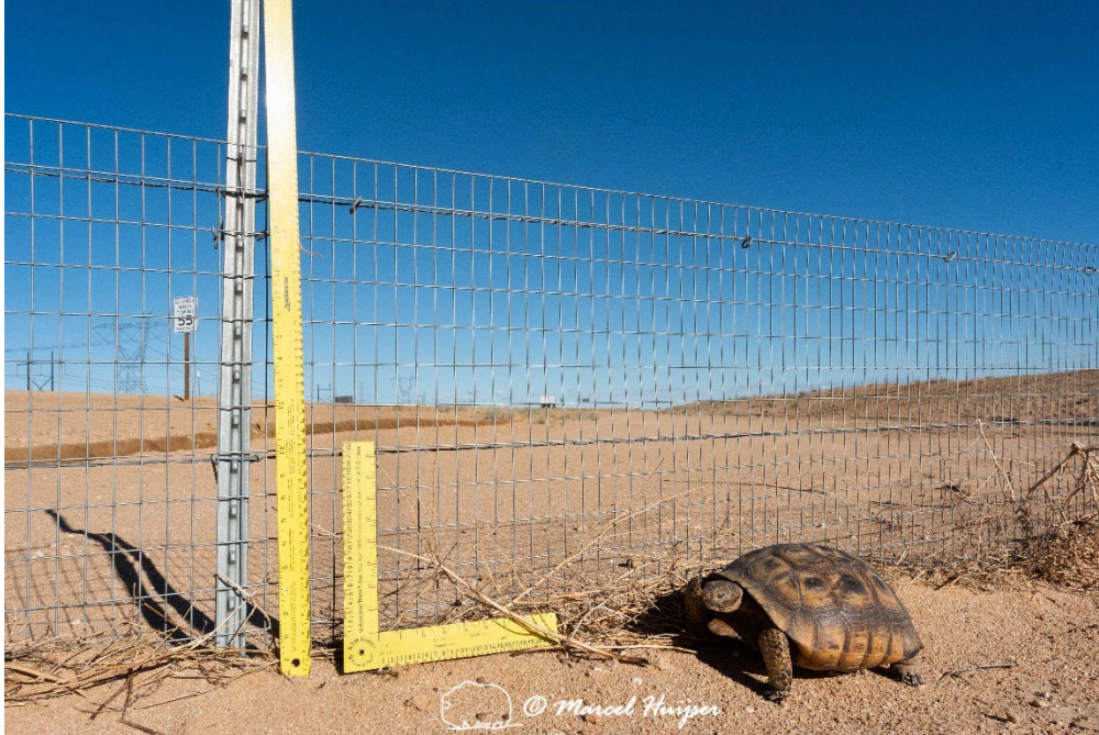
Mojave desert tortoise fence (height above ground 24 inches, presumably buried 12 inches below ground level, mesh size 1 inch wide, 2 inches tall), Hwy 58 near Kramer Junction, California. The fence material is attached to smooth wires at 10 and 22 inches above the ground.
