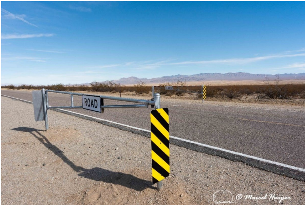
Gates for seasonal road closure to reduce road mortality of Mojave desert tortoise, Mojave National Preserve, California.
