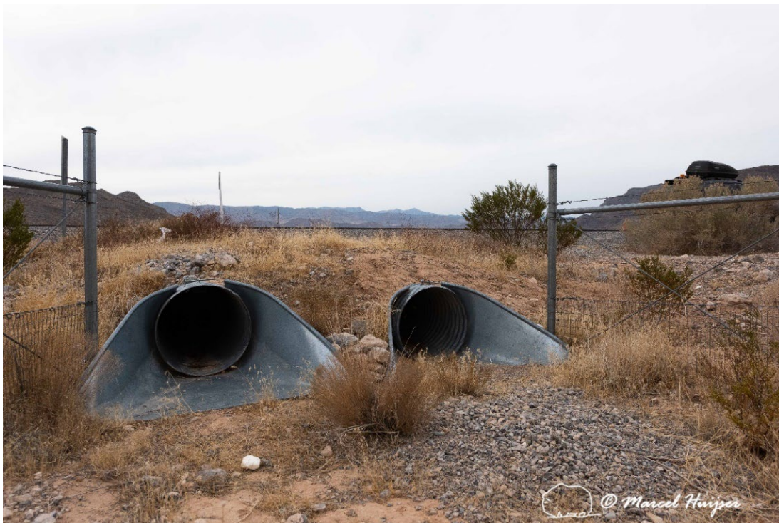
Mojave desert tortoise fencing connected to twin culverts, US Hwy 93 (MP 69.5 NB) near Overton, Nevada. The fencing would be a more effective barrier if it was continued above the culvert without any gap in the fence.
