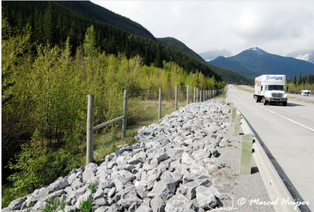
Boulder field at a fence-end, shielded through a guard rail, Alberta, Canada.
