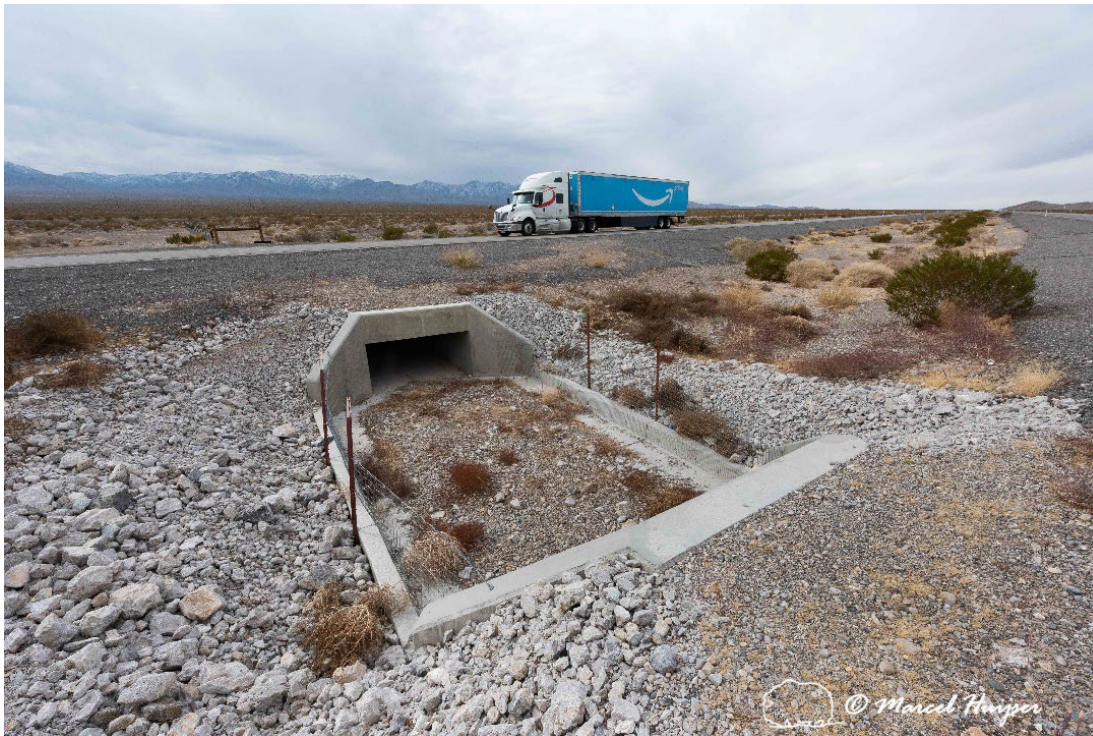
Open medians with separate crossing structures for the two travel directions should have Mojave desert tortoise fencing installed to prevent tortoises from accessing the fenced road corridor in the median.
