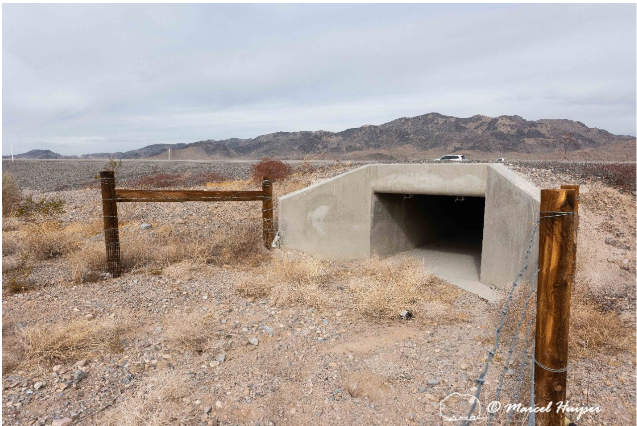
A multifunctional concrete culvert with natural substrate leading up to it, primarily designed for hydrology, but adapted for use by Mojave desert tortoises, US Hwy 95 (MP 125 SB) near Indian Springs, Nevada.
