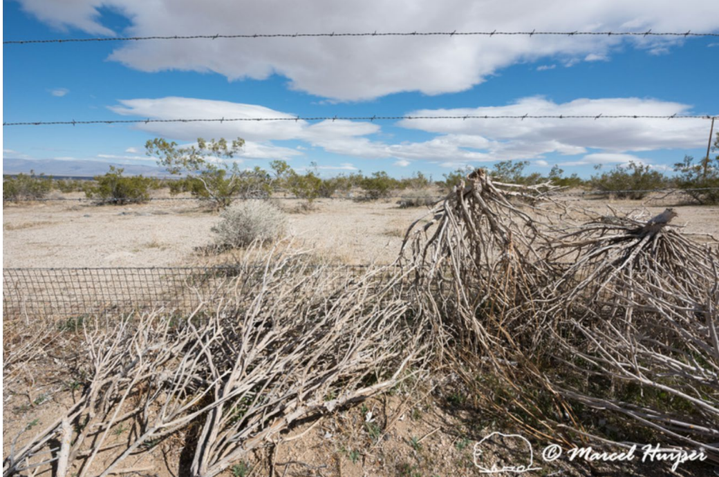
Dead vegetation has blown against the Mojave desert tortoise fence, reducing the barrier effect of the fence to keep tortoise from accessing the highway, Aerospace Hwy, Hwy 14 near Inyokern, California. Note that the height of the fence, as installed, is insufficient to begin with.
