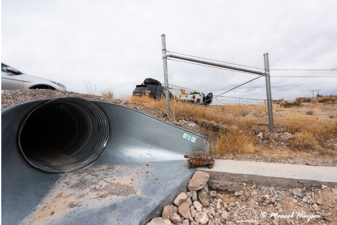
Mojave desert tortoise fencing connected to a culvert, US Hwy 93 (MP 58 NB) near Overton, Nevada. The fencing would be a more effective barrier if it was continued above the culvert without any gap in the fence.
