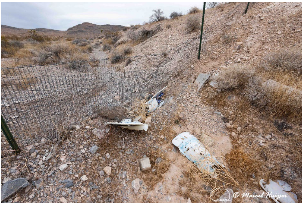
Mojave desert tortoise exclusion fencing across a desert wash with sedimentation at the fence, US Hwy 93 (MP 58 NB) near Overton, Nevada. The sedimentation reduces the effective height of the fence, and it may eventually threaten the integrity of the fence. Also note that the fence material has been cut in multiple overlapping segments to allow for the change in angle because of the change in slope (see next image for details).
