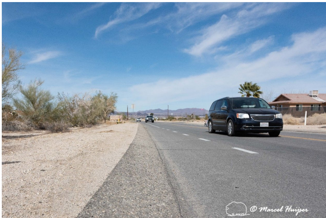
While the shoulder is still accessible to vehicles, this gentle sloped curb allows Mojave desert tortoises to leave the road, Twentynine Palms, California.
