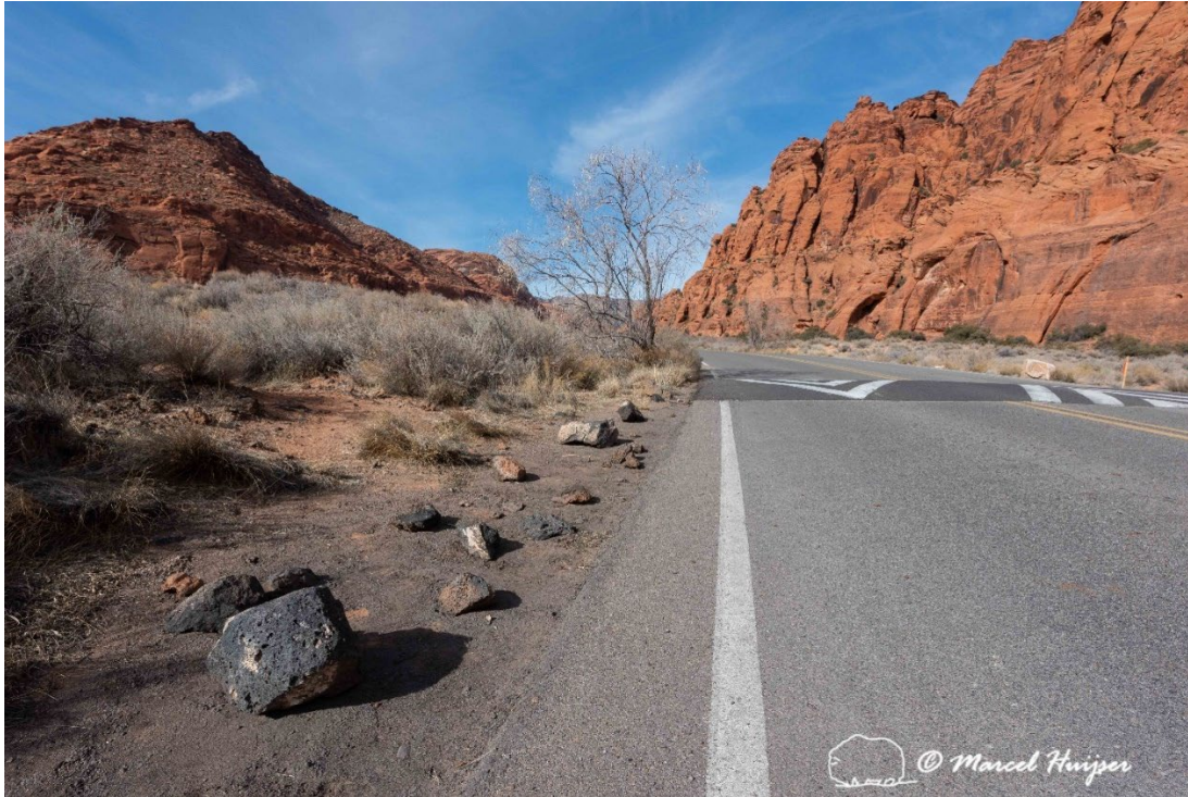
Large rocks along edge of pavement to discourage off road parking that destroys vegetation and that could kill Mojave desert tortoise, Snow Canyon State Park, St. George, Utah.
