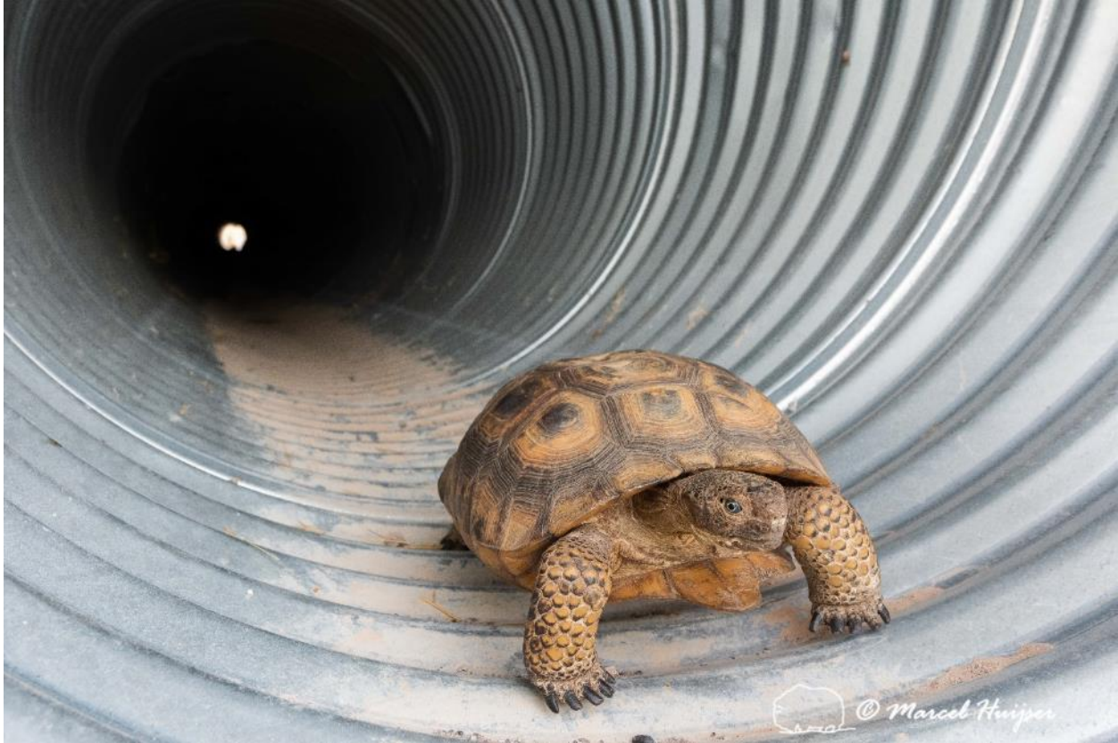
An adult tortoise model in a corrugated metal culvert (Corrugated Metal Pipe (CMP)), US Hwy 93 (MP 58 NB) near Overton, Nevada. Adult tortoises have been observed passing through these types of culvert structures, regardless of whether natural substrate was present (BLM and DCP 2022).
