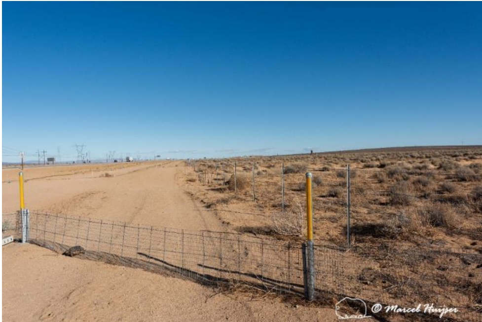
A gate associated with Mojave desert tortoise exclusion fencing, Hwy 58 near Kramer Junction, California. Note that the design of this gate resulted in gaps which affected its function as a barrier to Mojave desert tortoises (see images below).
