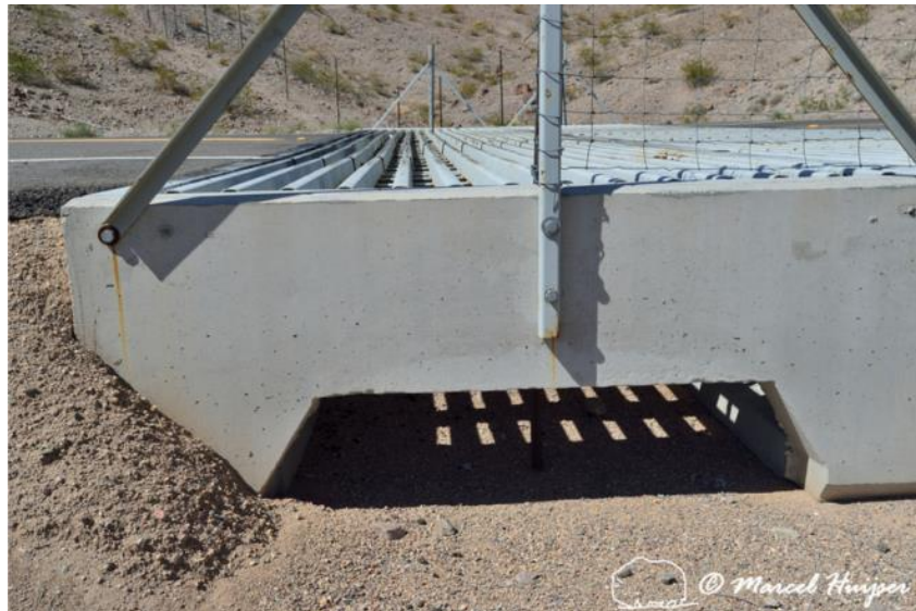
Combined drainage and escape for small animal species under a wildlife guard, Arizona, USA. While the metal bar design of this particular wildlife guard is not appropriate as a barrier for Mojave desert tortoises, the openings on the concrete walls on the side allow invertebrates, amphibians, reptiles, small mammals and other species that may fall in between the metal bars to escape to the safe side of the fence (not the roadside). For wildlife guards that have a fully enclosed pit with contiguous walls wooden planks or metal strips are sometimes attached, allowing animals to climb out of the pit. Wildlife guards are no longer recommended because Mojave desert tortoises may still cross and there may be maintenance issues if debris (e.g. tumbleweed) gets stuck in the pit (Pers. com. Kerry Holcomb, USFWS).
