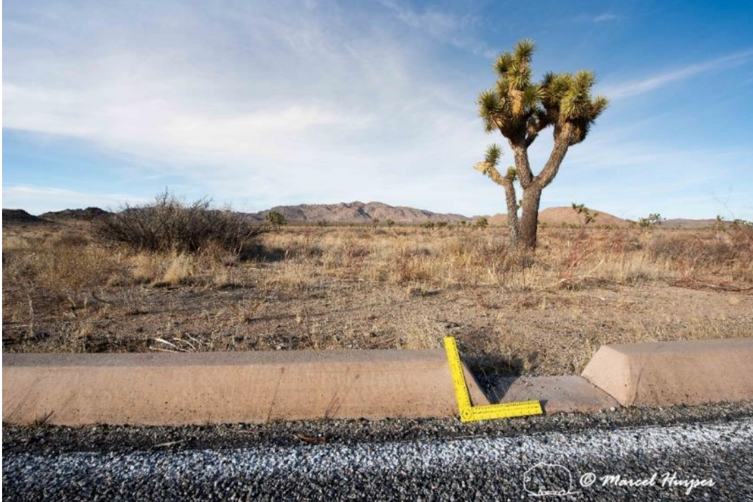
Tortoise trot, or gap in the curb, allowing Mojave desert tortoise to leave the road, Joshua Tree National Park, California.
