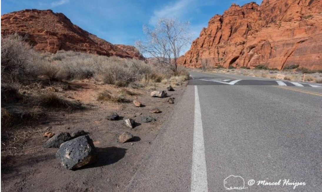
Large rocks along edge of pavement to discourage off road parking that destroys vegetation and that could kill Mojave desert tortoise, Snow Canyon State Park, St. George, Utah.
