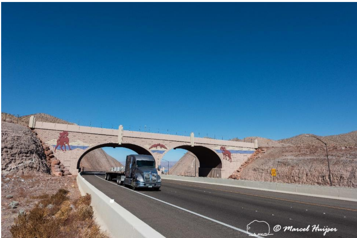
Wildlife overpass primarily designed for desert bighorn sheep, I-11, near Boulder City, Nevada.
