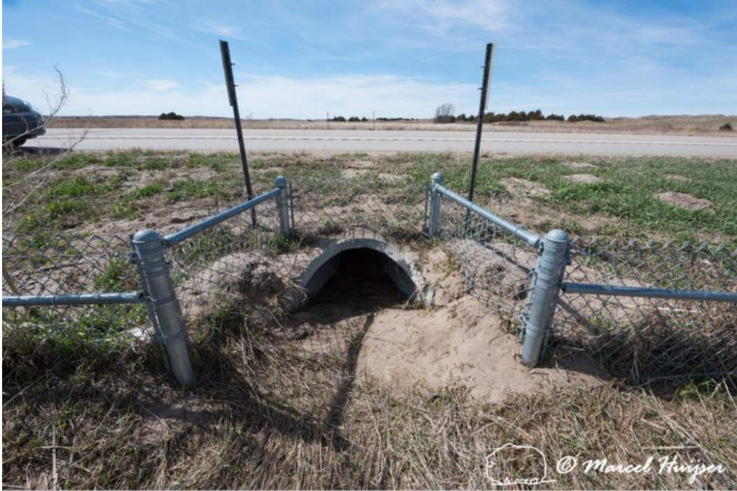
Turtle fence and a dry culvert used by turtles, Valentine National Wildlife Refuge, Ballard's South, Valentine, Nebraska, USA. This culvert is 30 inches wide, 22 inches tall. Note that this turtle fence has no gap and continues behind and on top of the culvert.
