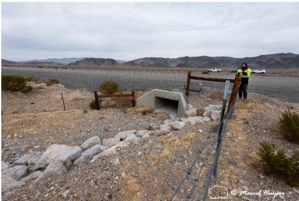
Mojave desert tortoise fencing and a concrete box culvert, US Hwy 95 (MP 127.5 SB) near Indian Springs, Nevada. Note that the fence on the near side is located on top of the bank of the desert wash, and not in the wash or on the bank.
