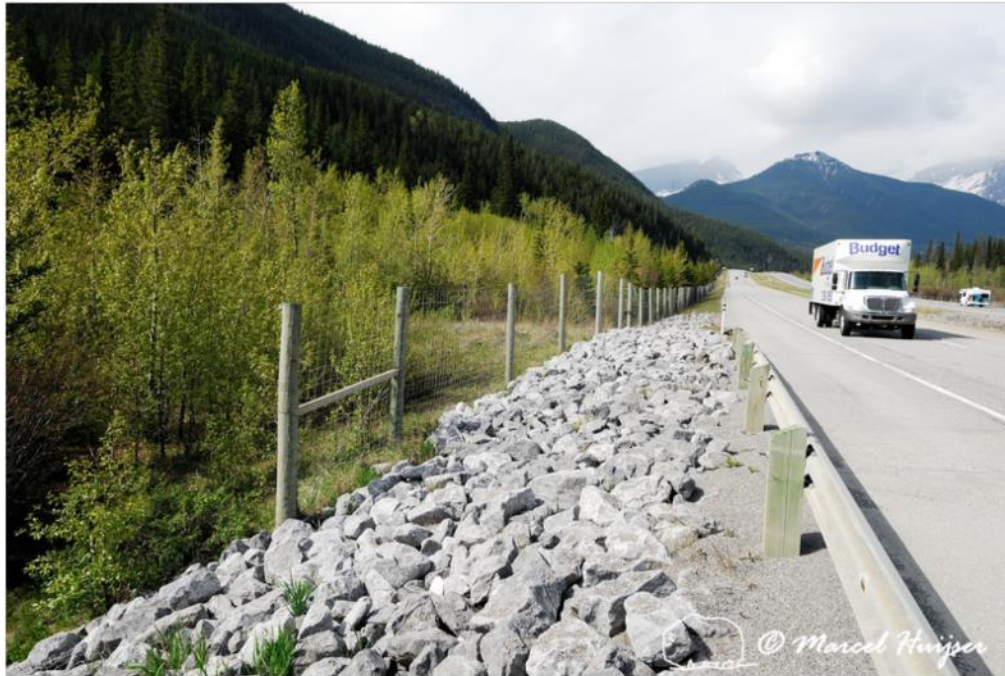
Boulder field at a fence-end, shielded through a guard rail, Alberta, Canada.
