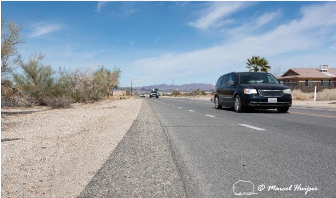
While the shoulder is still accessible to vehicles, this gentle sloped curb allows Mojave desert tortoises to leave the road, Twentynine Palms, California.
