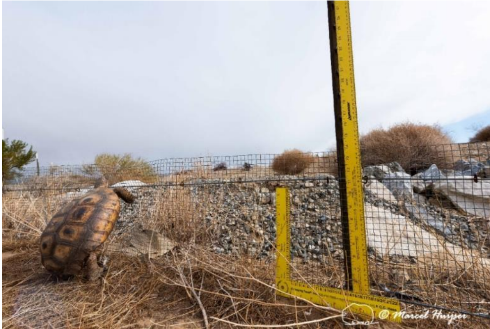
Mojave desert tortoise fence (about 14 inches tall, mesh size about 1x1 cm), I-15 near Barstow, California. The small mesh size may pose a greater risk to small animal species (lizards, snakes) getting stuck and dying. Small mesh sizes are also more likely to catch sediment. Note that this fence is too low and there is no smooth wire at the very top of the fence, making the fence less rigid.
