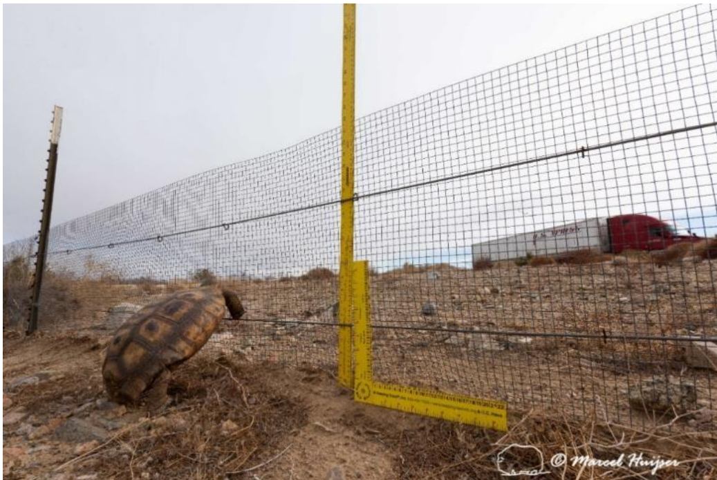
Mojave desert tortoise fence (about 21.5 inches tall, mesh size about 1x1 cm), I-15 near Barstow, California. The small mesh size may pose a greater risk to small animal species (lizards, snakes) getting stuck and dying. Small mesh sizes are
