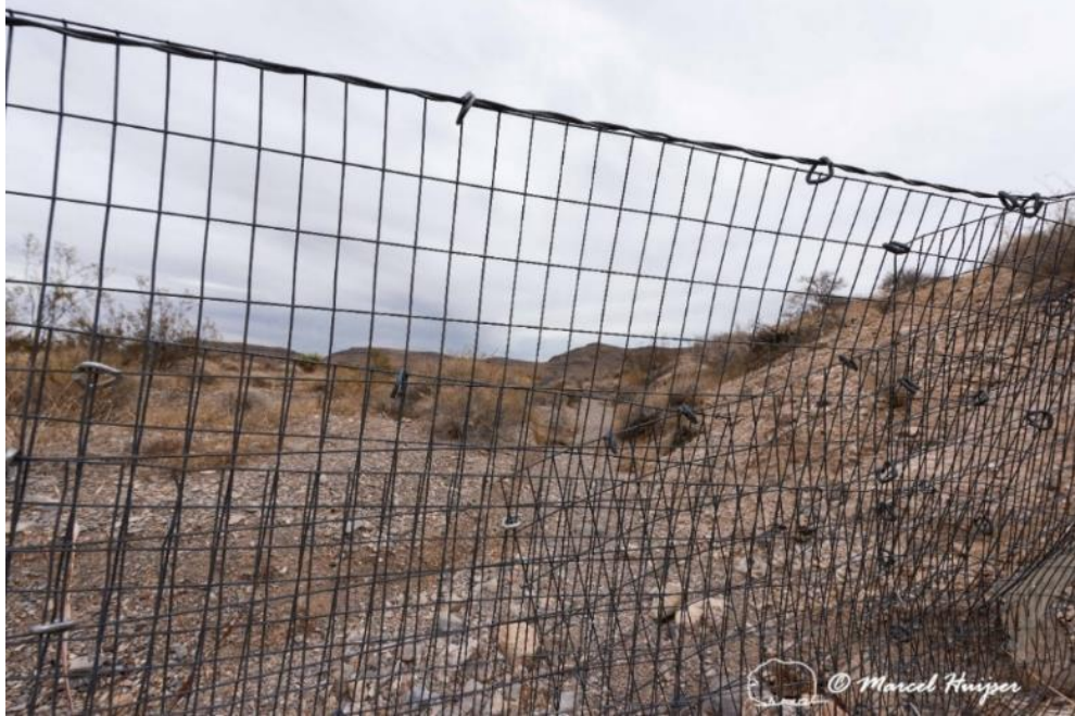
Detail of Mojave desert tortoise fencing, US Hwy 93 (MP 58 NB) near Overton, Nevada. Because of the change in slope (higher bank towards the right), the fence material was cut and installed in multiple overlapping segments.
