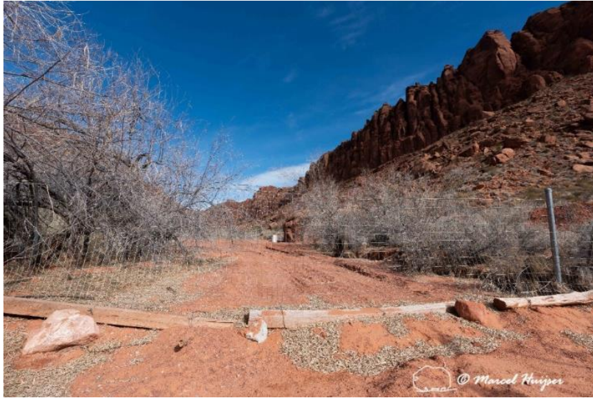
Mojave desert tortoise exclusion fencing across a desert wash, St. George, Utah. Here the fence crosses a desert wash. The cedar logs will float and lift up the fence during a flooding event. This minimizes damage to the fence because of flooding and debris.
