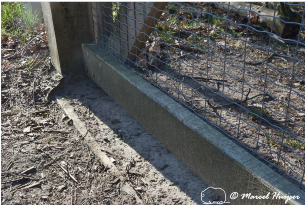
Snug fit of a gate at a wildlife fence, south of Otterlo, The Netherlands. The snug fit discourages animals from crawling under the gate.
