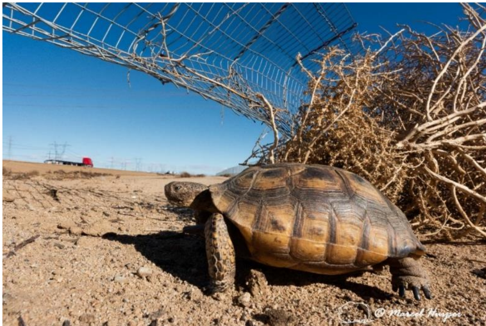
Gap under a gate associated with Mojave desert tortoise exclusion fencing, Hwy 58 near Kramer Junction, California. The gate does not have a buried component, and it had enough flex to result in permanent openings, partially as a result of tumbleweeds being blown against the fence.
