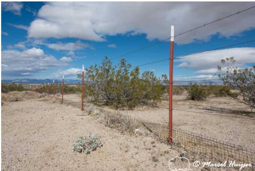
Mojave desert tortoise exclusion fence, USA Aerospace Highway (Hwy 14), near Inyokern, California. The small mesh size may pose a greater risk to small animal species (lizards, snakes) getting stuck and dying. Small mesh sizes are also more likely to catch sediment. Note that this fence is far too low (perhaps only a few inches) to be a functional barrier for Mojave desert tortoises.
