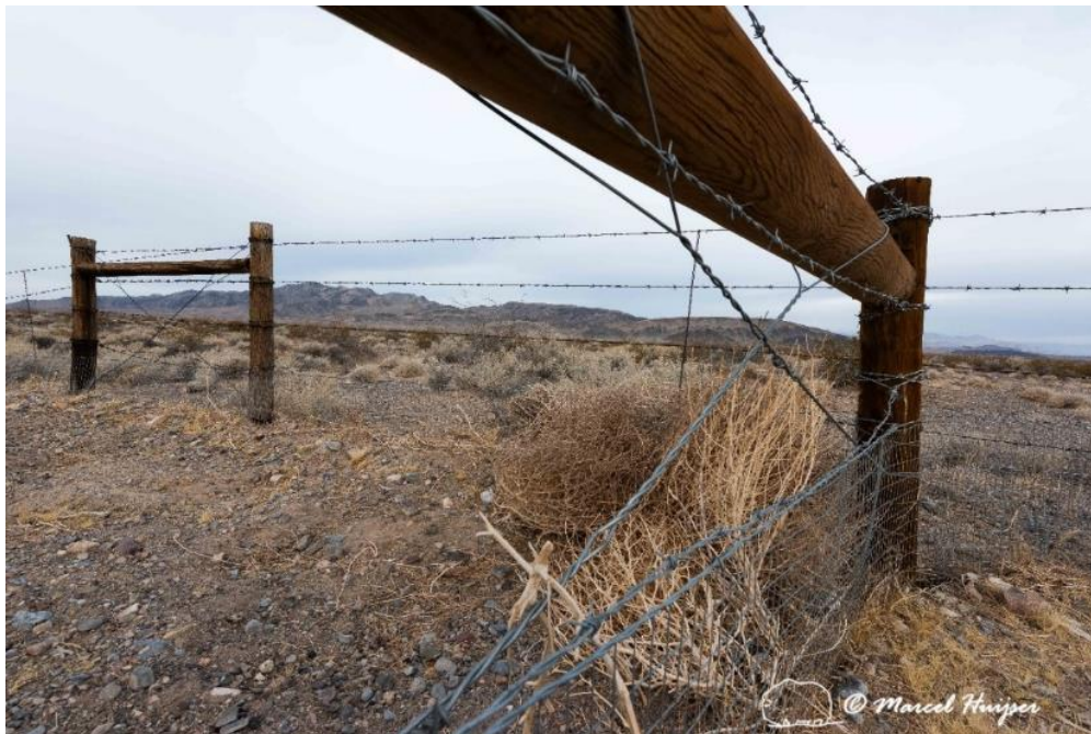
Mojave desert tortoise fence blocking access to a culvert that is considered a danger (e.g. entrapment between riprap or drowning in a deep plunge pool), US Hwy 95 (MP 125 NB) near Indian Springs, Nevada. The decision to block tortoises from accessing the culvert implies that the danger associated with accessing and using a culvert is considered greater than the benefits of potential crossings.
