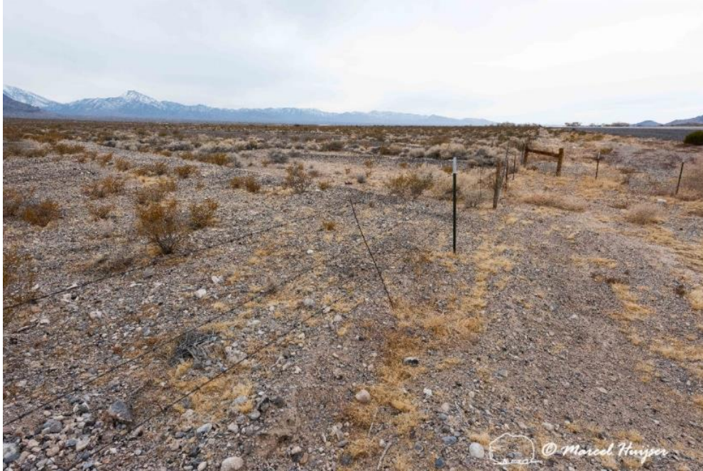
Mojave desert tortoise fencing, US Hwy 95 (MP 121.6 SB) near Indian Springs, Nevada. This is a right-of-way and cattle fence installed across the wash, intended to keep cattle from entering the culvert (which is to the right). The Mojave desert tortoise fencing (upper right) angles away from the property boundary towards the culvert.
