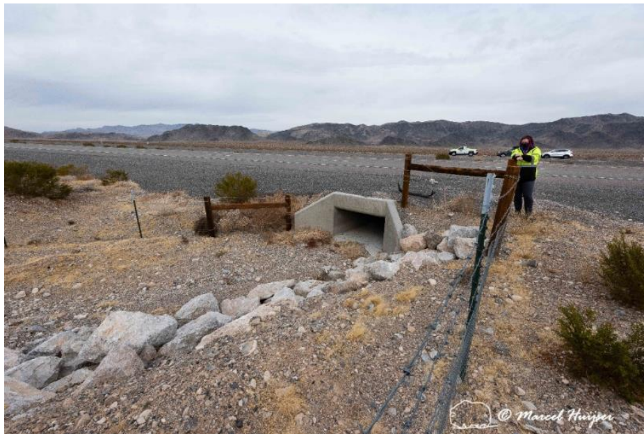
Mojave desert tortoise fence and a culvert US Hwy 95 (MP 127.5 SB) near Indian Springs, Nevada. Riprap stabilizes the slope between the fence and the culvert. Mojave desert tortoises that follow the fence cannot easily access the culvert; they would have to navigate the riprap on the slope first. Design and construction of culverts, fences, and measures aimed at erosion control should ensure that tortoises can easily access the culvert, including when they follow the fence.
