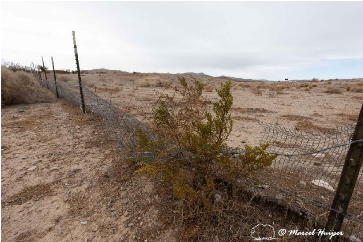
Mojave desert tortoise fencing, I-15 near Barstow, California. The fence is in disrepair and a shrub has grown through the fence, reducing its effective height.
