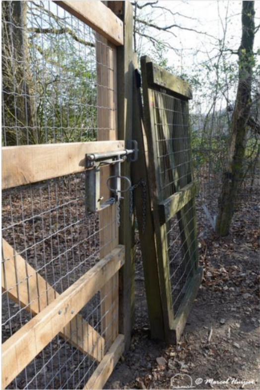
Swing gate, set at an angle so it closes through gravity, The Netherlands.
