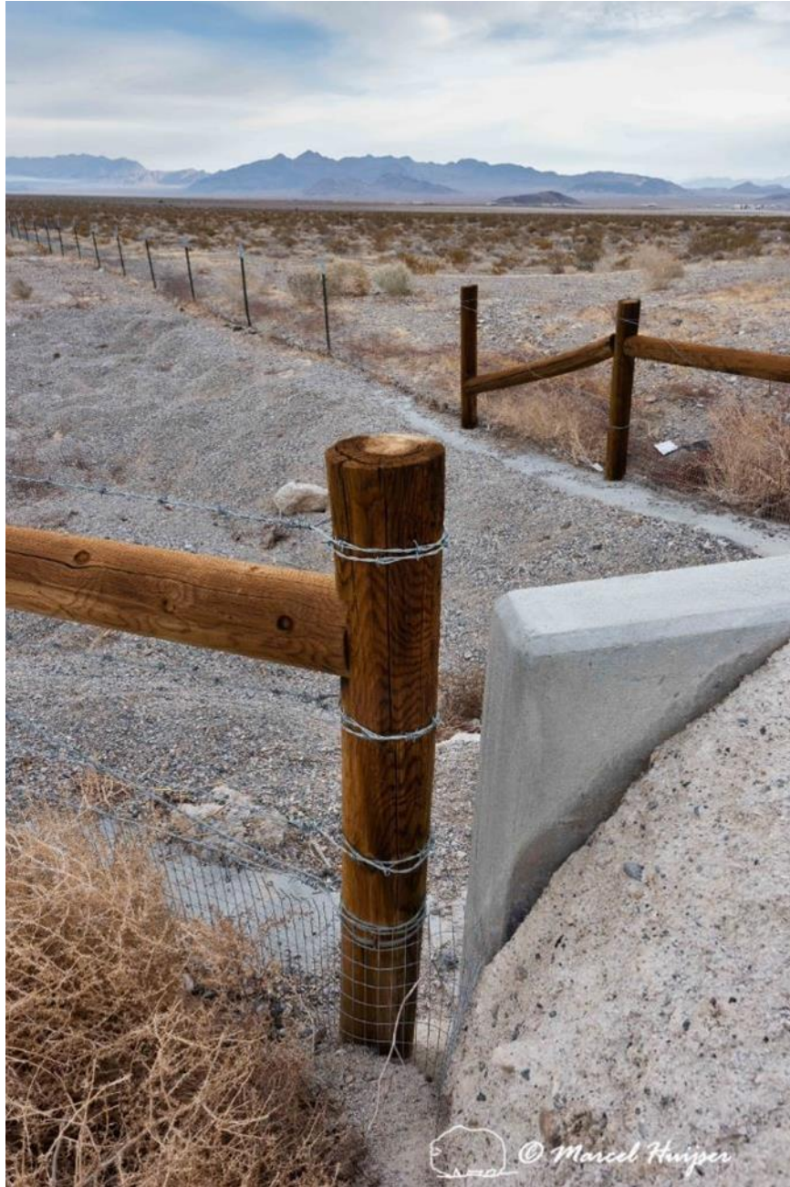
Mojave desert tortoise fencing connected to a culvert, US Hwy 95 (MP 121.6 NB) near Indian Springs, Nevada. Note concrete access paths for Mojave desert tortoises constructed along the fence.
