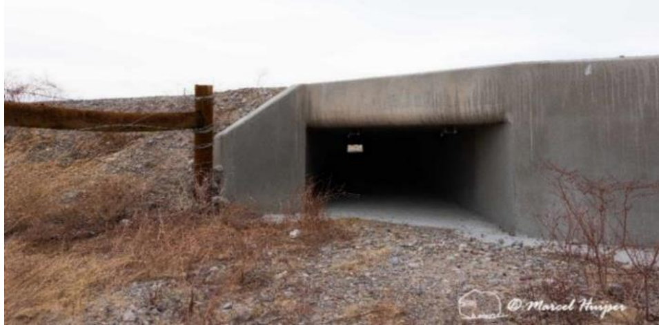
Mojave desert tortoise fence and a culvert with concrete pathways leading up to the entry, US Hwy 95 (MP 121.6 SB) near Indian Springs, Nevada. This inflow shows no noticeable erosion; Mojave desert tortoises of any size can easily access this culvert across the entire width of the culvert.
