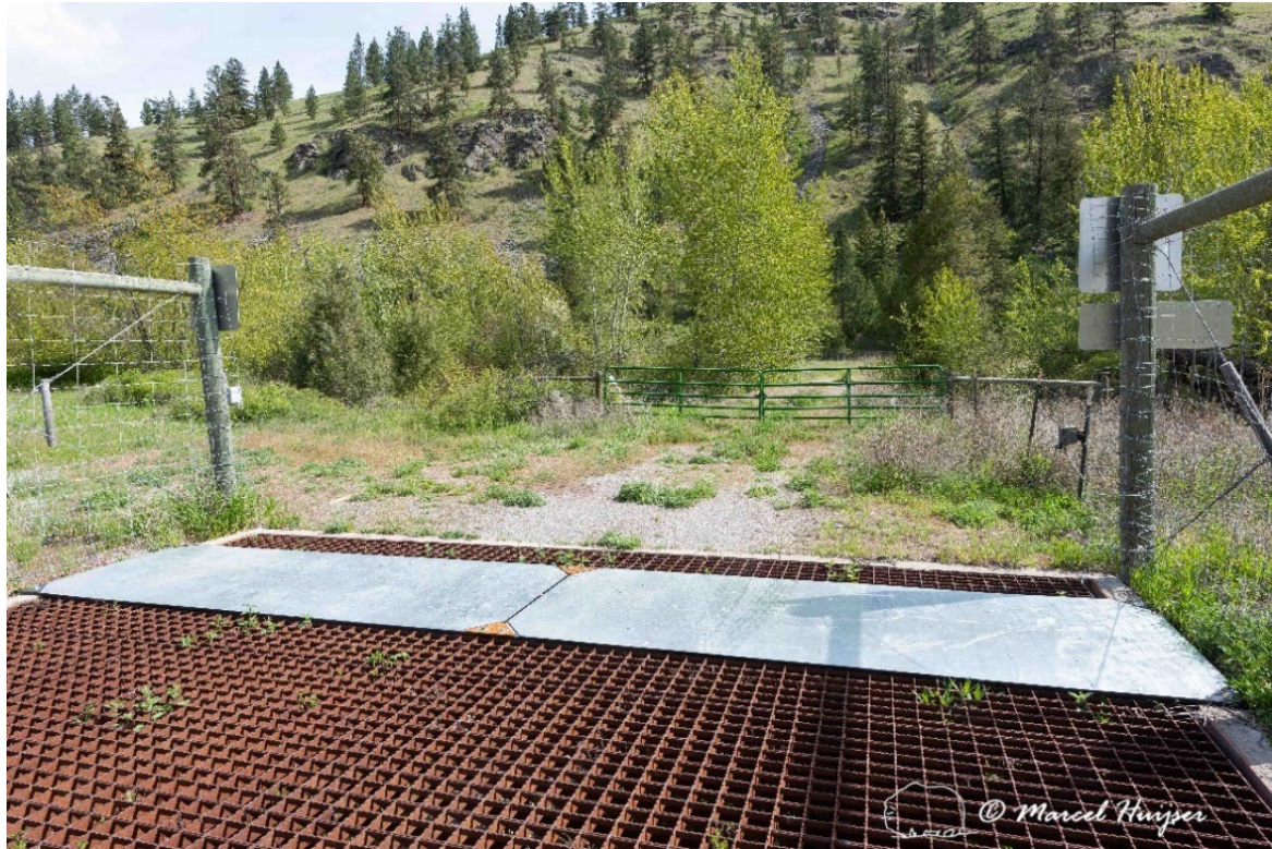
Figure 4: The electrified mat installed by BS Fabrications at the south wildlife guard, US Hwy 93, south of Ravalli, Montana.
