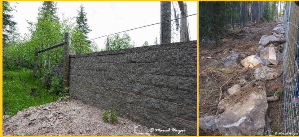
Figure 2. Examples of a wildlife jump-out along US Hwy 93, Flathead Indian Reservation, Montana, USA and wildlife fence and dig barrier (or apron), TransCanada Highway, Banff National Park, Alberta, Canada
