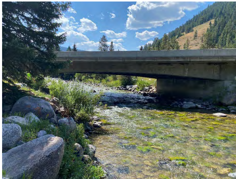
Figure 22 Bridge over Taylor Fork (RM 33.9)
