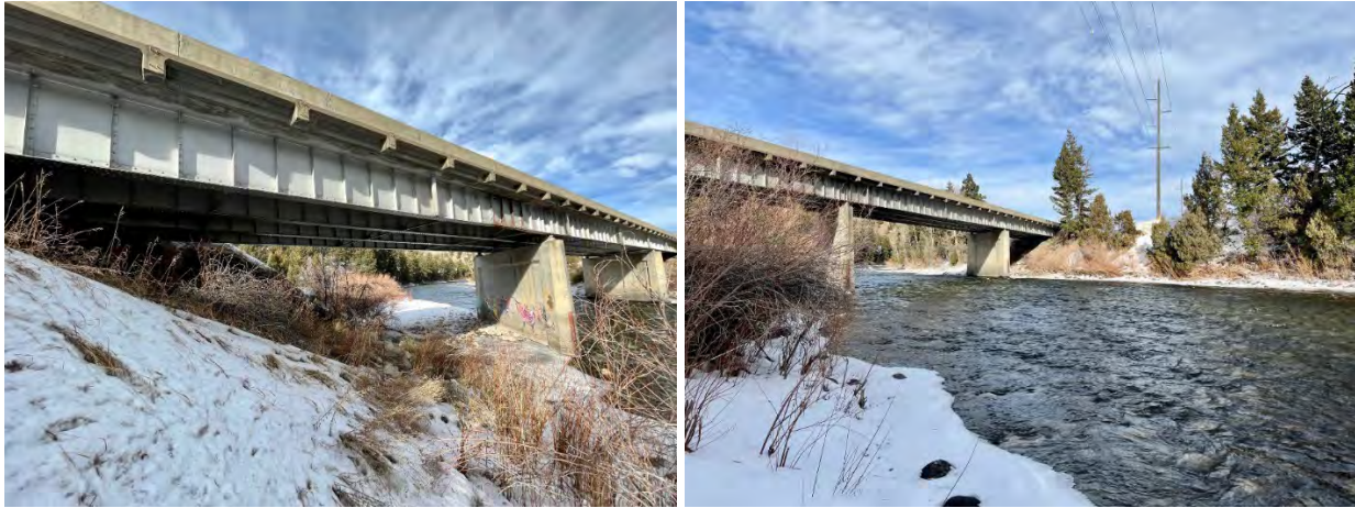
Figure 27 Gallatin River Bridge (RM 70.5)
