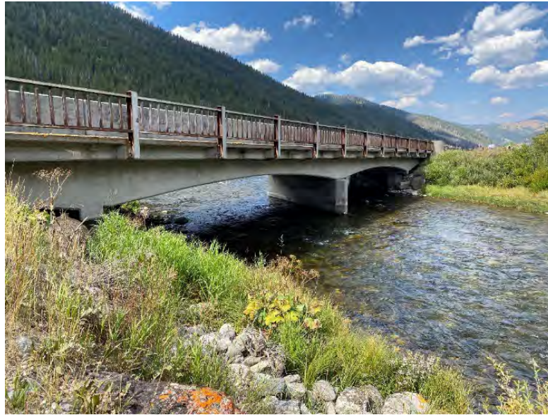
Figure 20 Bridge over the Gallatin River (between RM 23-24)
