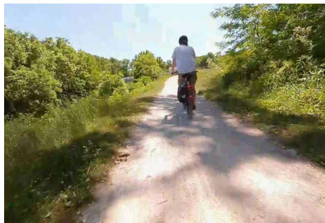
Figure 11: A crushed limestone trail surface.
