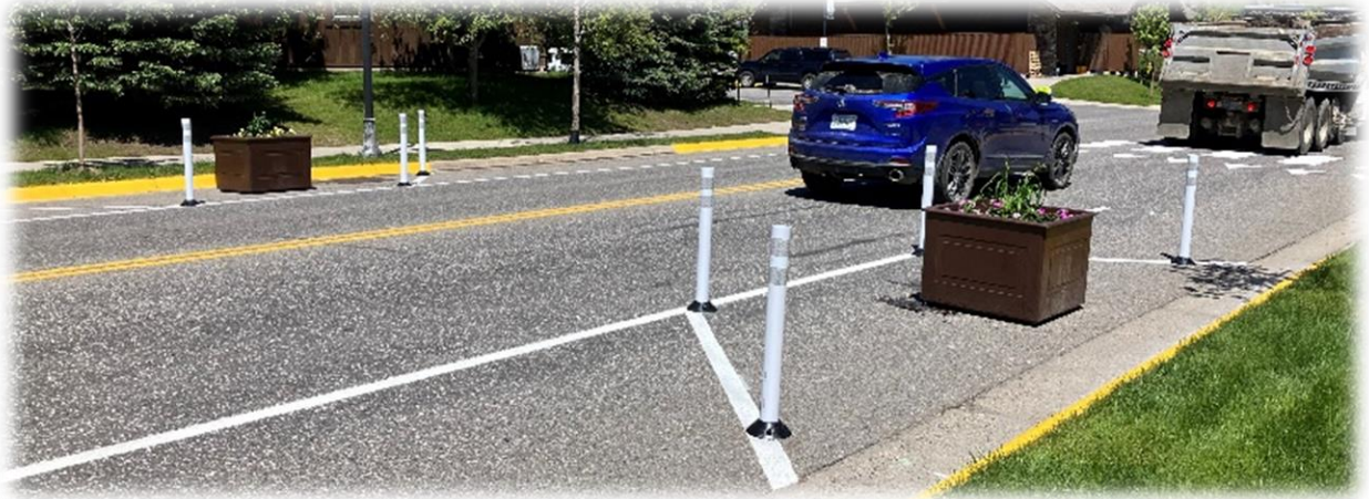
Figure 15. Gateway curb extensions on Ousel Falls Rd.
