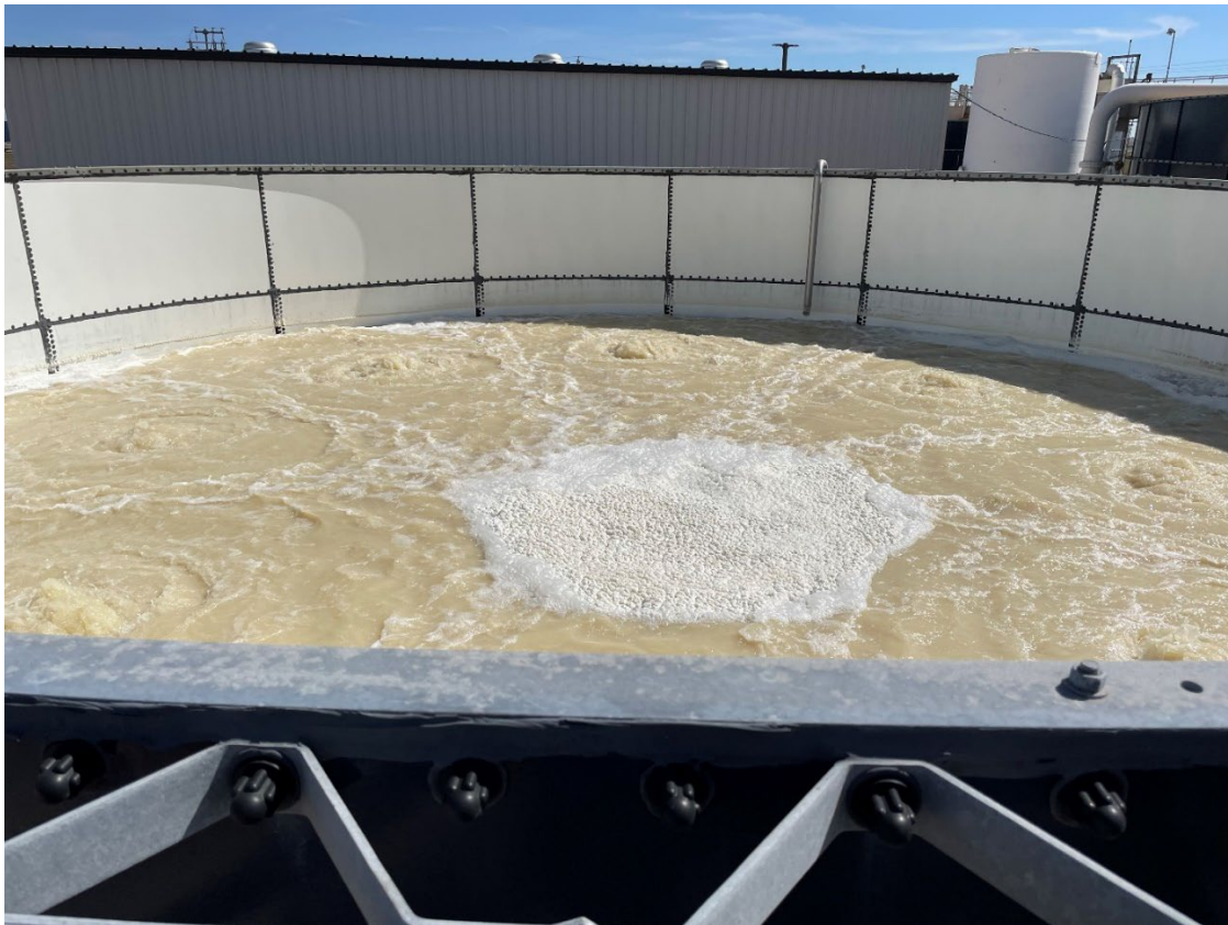
Figure 9. LCB storage tank at Leprino Foods in Fort Morgan, CO.
