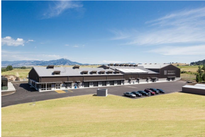
Figure 1. Hyalite/Sourdough Water Treatment Plant
