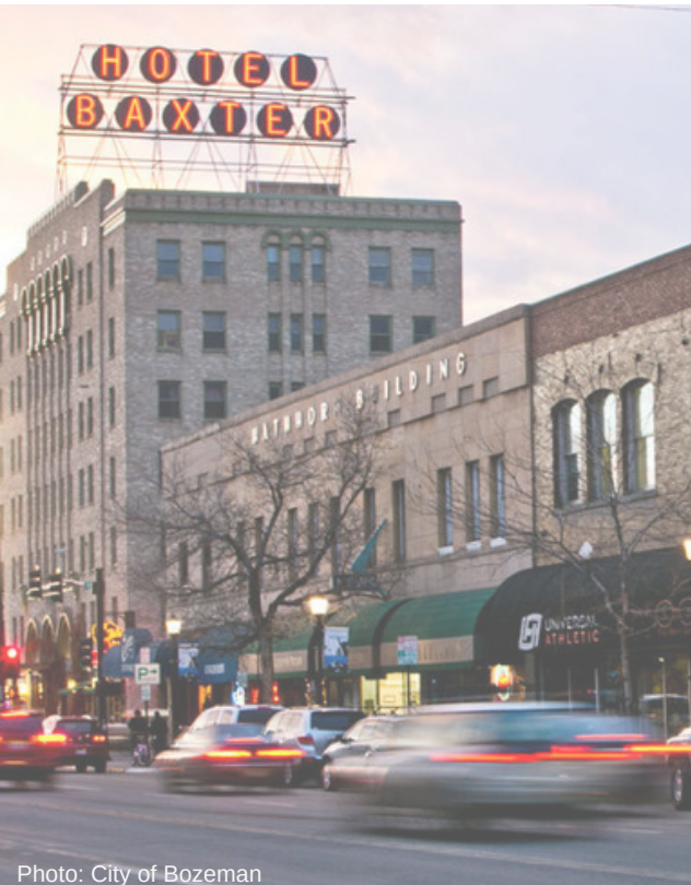
Photo: City of Bozeman
