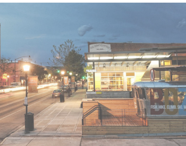
Photo: City of Bozeman
