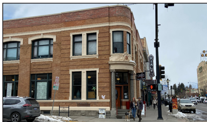
Building entrance facing the street corner.
