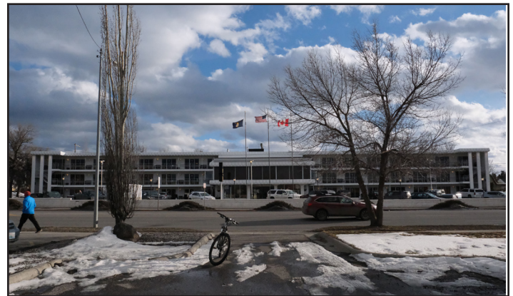
This photo shows a departure of the parking code. The code states no more than 50% of street frontage may be taken up by surface parking, while at the Lewis and Clark Motel has 100% of street frontage taken up by surface level parking.
