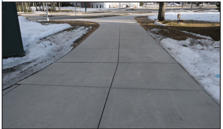
This photo taken at the corner of College st. and 11th ave. shows a sidewalk along an arterial route that is greater than 6' (about 9' wide).
