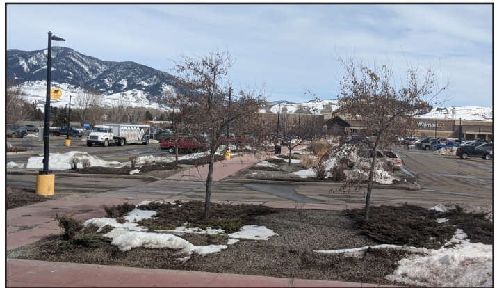
In this parking lot, they built a walkway from the entrance to back of the parking lot in order to create a safe place to walk. Photo Source: Alec Humphries
