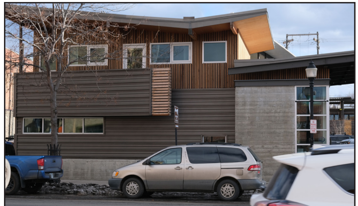
This photo taken outside The Lark shows a departure from the transparency code that states at least 25% of the ground level facade must be transparent. A possible compromise being the interesting architecture.
