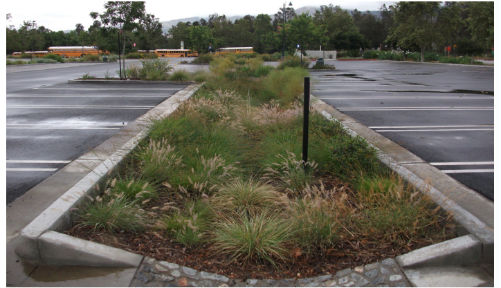
Sec. 38.550.050, H, 2: curb departure example - superior design standards allowing for stormwater management.
