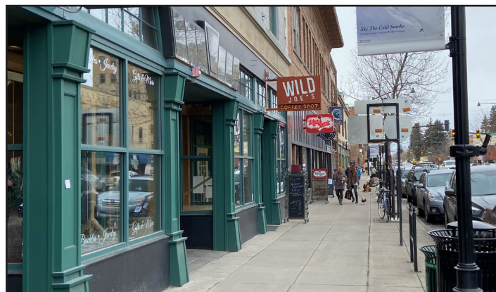
Buildings must be on the back edge of the sidewalk.
