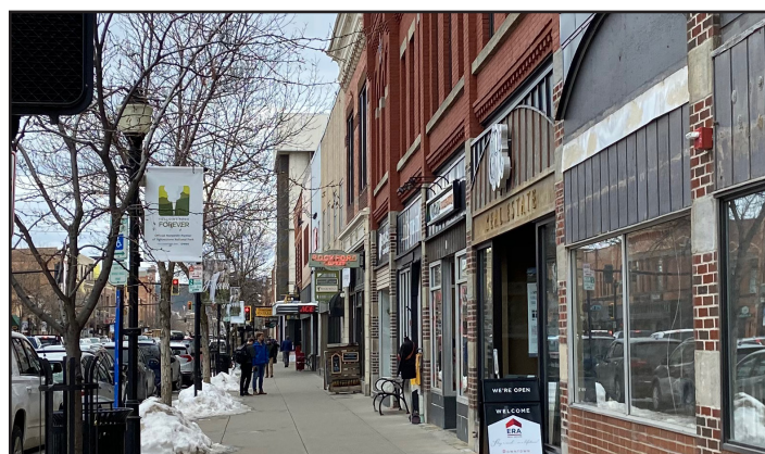
Alternative weather protection with the doors being setback into the building and covered by the roof.
