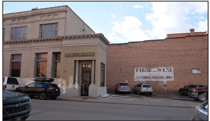
This photo taken on the corner of Main st. and Tracy ave. shows the juxtaposition of proper transparency codes (likely a newer building) and a building that is not up to code (likely built before codes were set in place).
