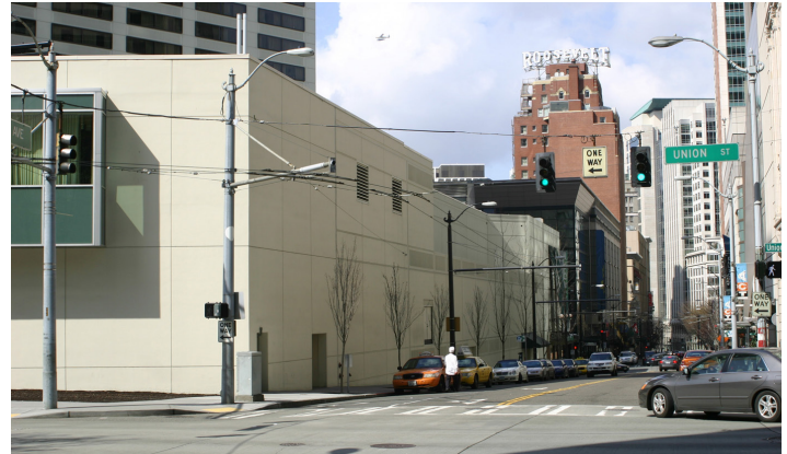
The blank walls the code is trying to mitigate.
