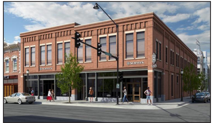
Commercial first floor with glass design and pedestrian space.
