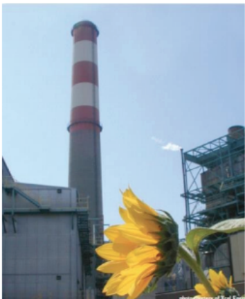
Xcel Energy's Cherokee Station in Denver, Colorado where reclaimed water feeds the plant's cooling towers (photo source: Xcel Energy)
