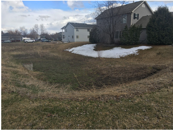
Figure 11: Probable Rating: Fair (2) Pond bottom is clear but pond sides have overgrown vegetation
