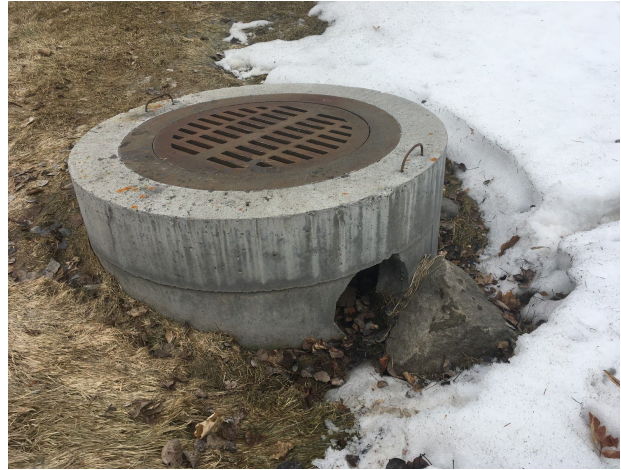
Figure 14: An outlet structure in good condition. No noticeable cracking.
