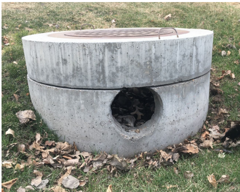
Figure 4: Probable Rating: Good (1) Slight debris in outlet structure, easily accessible, opening is not covered
