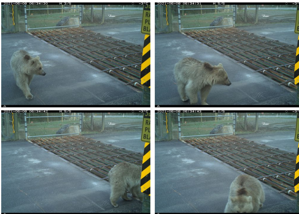
Figure 10: Grizzly bear receives an electric shock when attempting to enter the fenced road corridor at Lake O'Hara Road
