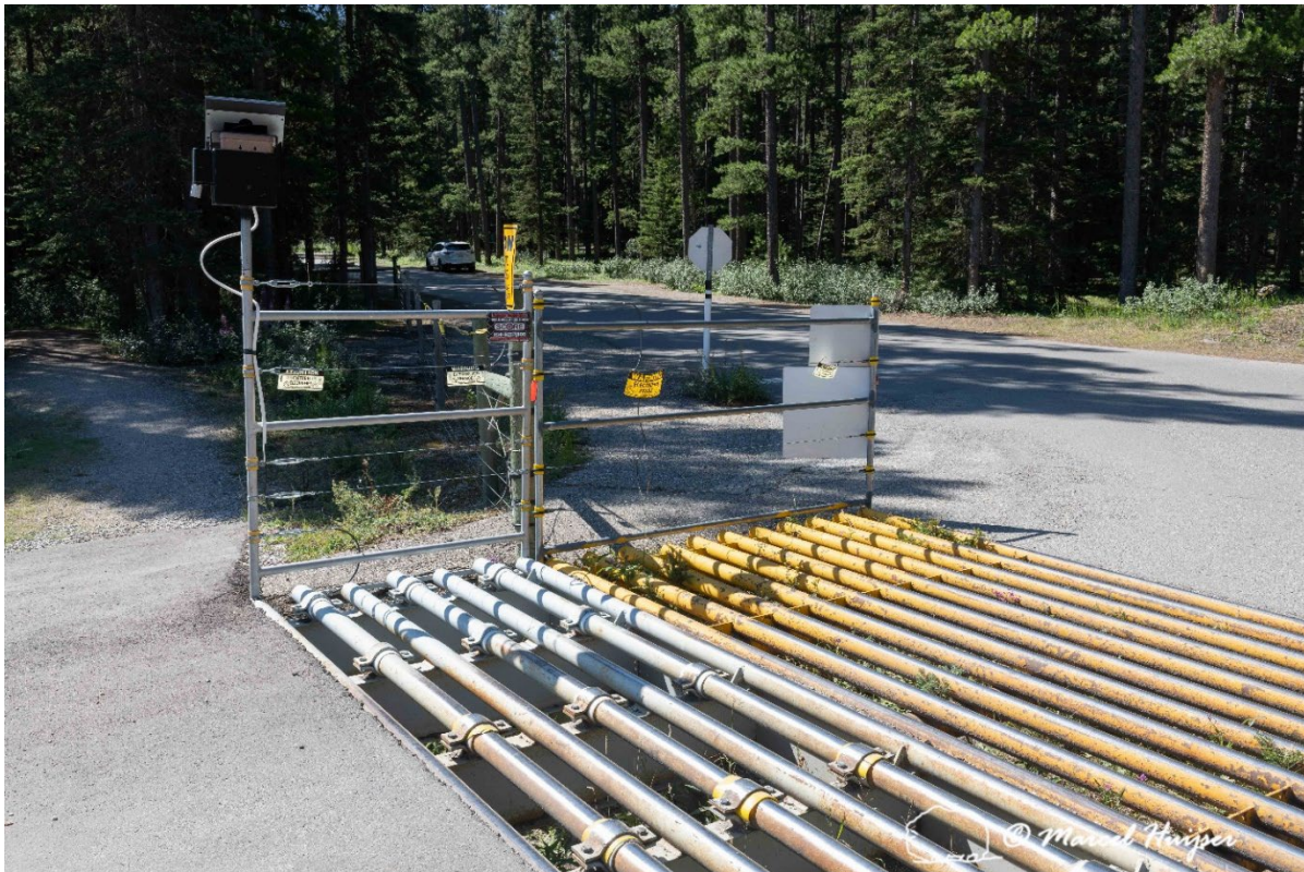
Figure 3: Electrified barrier, Lake Louise Campground, Lake Louise, Canada
