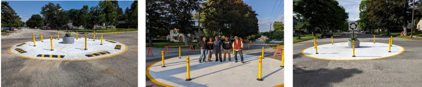
Figure 3: The pop-up traffic circles were completed (left, center, right) through the hard work of the installation crew (center).
