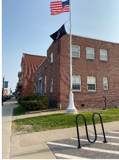
Figure 18: Pushed Over (and Disconnected on One Side) Bike Rack at the Post Office
