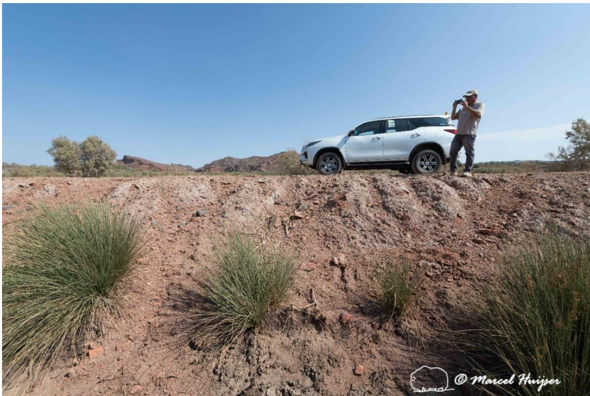
Figure 28: The dirt road is situated on an embankment for a portion of the wetland, near Fort Nazar, Kaybar, Medina Province, Saudi Arabia.
