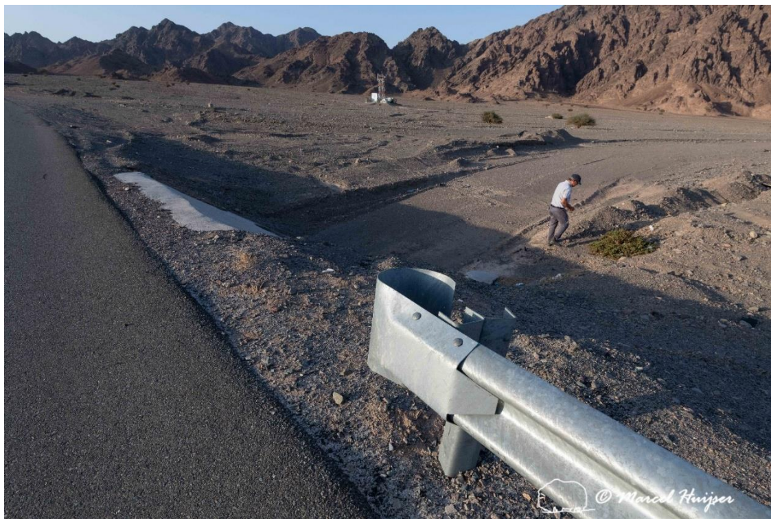
Figure 24: Human made channel in a desert wash at the outflow of a plugged culvert, Hwy 328 between Masader and Jadedah, AIUla, Medina Province, Saudi Arabia.
