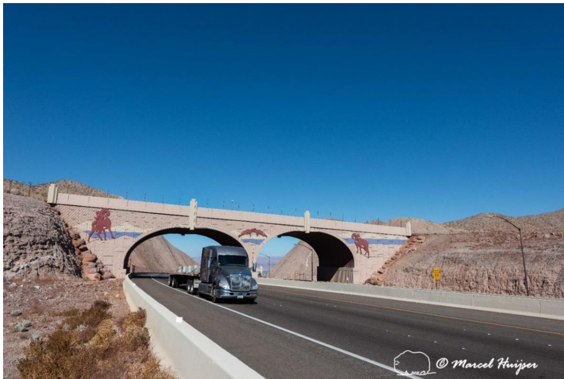
Figure 10: Wildlife overpass primarily designed for desert bighorn sheep, I-11, near Boulder City, Nevada, USA. Note that the bighorn sheep depicted on the overpass communicate the purpose of the overpass and that the design and color of the structure fit into the landscape better than a standard bridge design.
