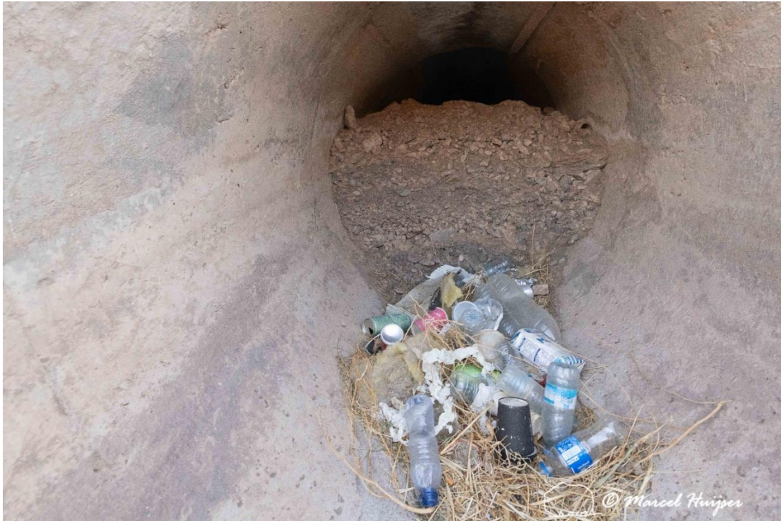
Figure 26: Plugged culvert south (downstream) of potential mitigation site for Nubian ibex ( Capra nubiana ), Hwy 328 between Masader and Jadedah, AIUla, Medina Province, Saudi Arabia.
