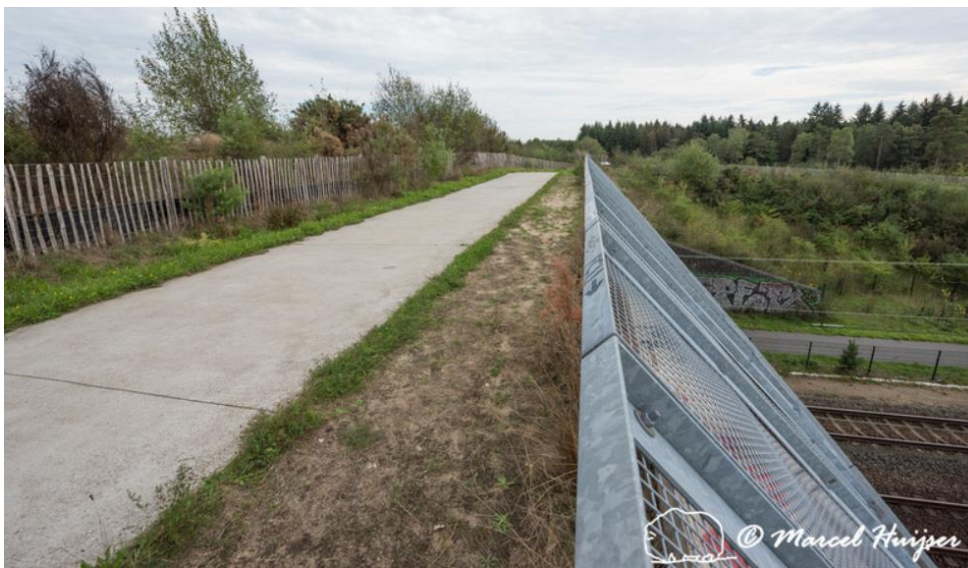
Figure 55. Hiking and biking trail combined with wildlife overpass across railroad tracks, Soest, The Netherlands. The vegetated “wildlife area” on the overpass is further to the left, separated from the trail by a berm and shrubs and trees.
