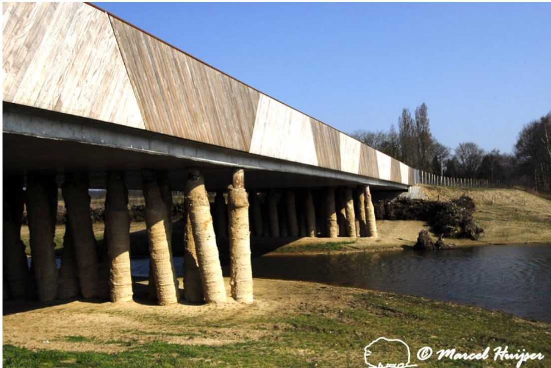
Figure 46. Wildlife underpass with dimensions that would be suitable for most large mammal species. Note the visual barrier. The barrier reduces visual and noise disturbance from traffic for the animals that approach the underpass.
