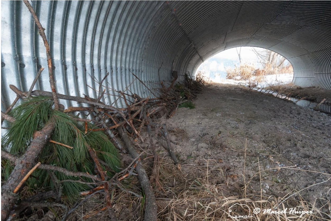
Figure 54. Underpass for large wild mammals made more suitable for small mammals, amphibians, and mammals by placing cover (branches) along the sides, Montana, USA.
