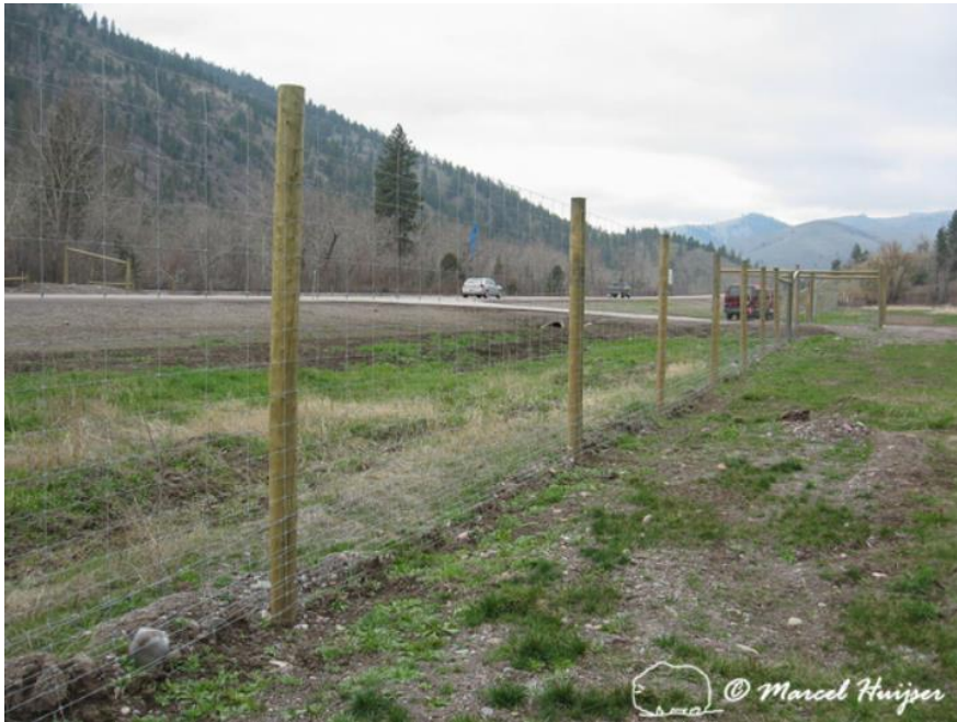
Figure 42. Typical large ungulate fence in North America, 8 ft tall, wooden posts and mesh-wire fence material, US Hwy 93 North, Montana, USA. Note that there is a dig barrier attached to the main fence material (e.g. for canids).
