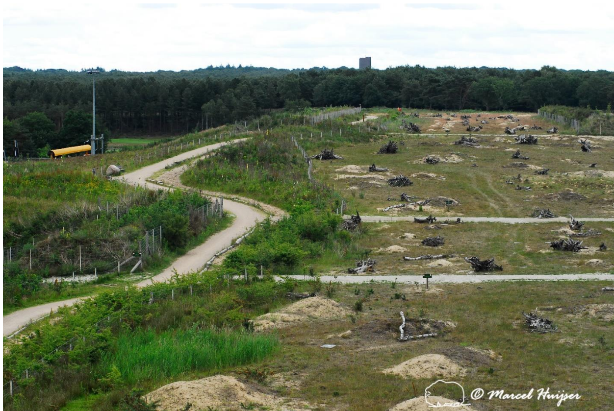
Figure 39. Ecoduct Natuurbrug Zanderij Crailoo, The Netherlands. On the far left is the trail for non-motorized recreation. A fence and vegetated berm separate the trail from the designated zone for wildlife to the right. The corridor is about 50 m wide and 800 m long and connects forests and heathlands on both sides. The corridor consists of embankments and two bridges. One bridge spans a two-lane highway, the other a railroad and railroad yard. The embankment also goes through sports fields.
