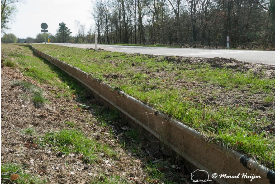
Figure 50. Barrier or wall for amphibians integrated into roadbed Deelenseweg between Hoenderloo and Arnhem Gelderland, The Netherlands.
