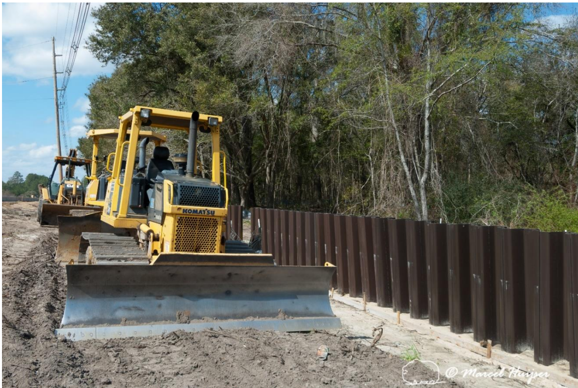
Figure 51. Barrier wall for turtles, alligators, snakes, and amphibians. Lake Jackson Ecopassage Tallahassee Florida USA.
