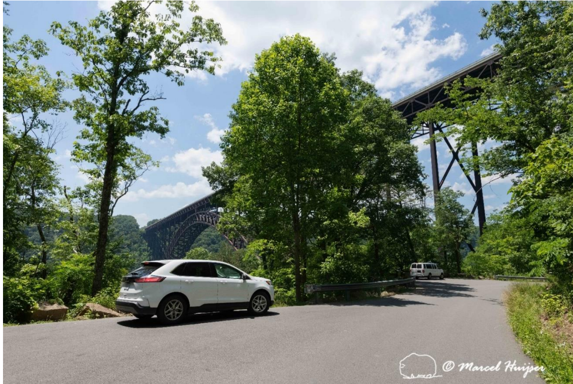
Figure 13: Fayette Station Road winds down the gorge under the New River bridge and has pull-outs, New River Gorge National Park and Preserve, Fayetteville, West Virginia.
