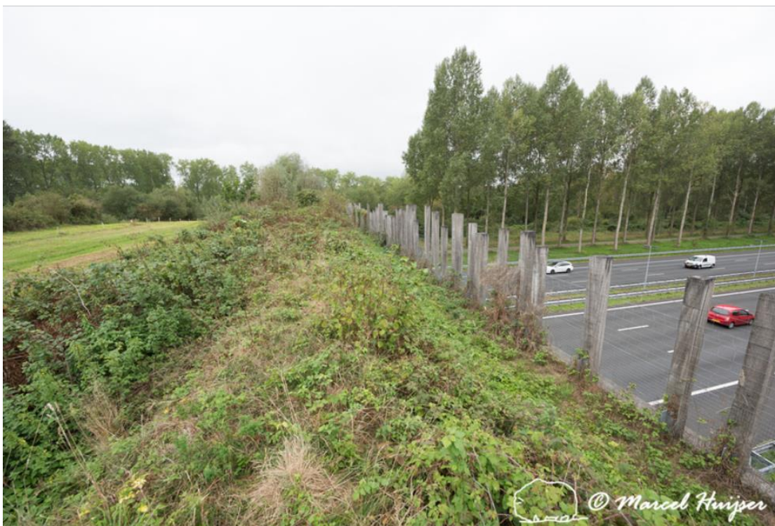
Figure 47. Wildlife overpass with dimensions that would be suitable for most large mammal species. Note the berm on wildlife overpass. The berm with root wads and shrubs provides cover on either side and reduces visual and noise disturbance barrier combined with large mammal fence on an overpass.
