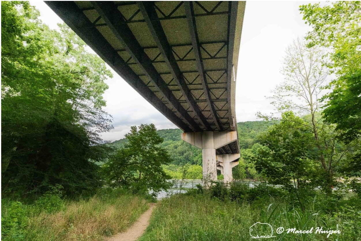
Figure 34: Highway 340 (William L. Wilson Freeway), bridge across Shenandoah River, from the viewpoint of the north bank at Harpers Ferry, West Virginia. The stairs up to the bridge are on the opposite bank.
