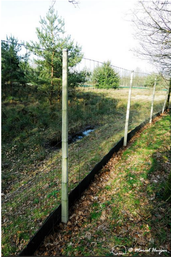
Figure 44. Wildlife fence for amphibians (e.g. common toad ( Bufo bufo )), medium sized mammals (e.g. Eurasian badger ( meles meles )) and large ungulates (e.g. roe deer ( Capreolus capreolus ), red deer ( Cervus elaphus )) at ecoduct Woeste Hoeve A50 near Apeldoorn, The Netherlands.
