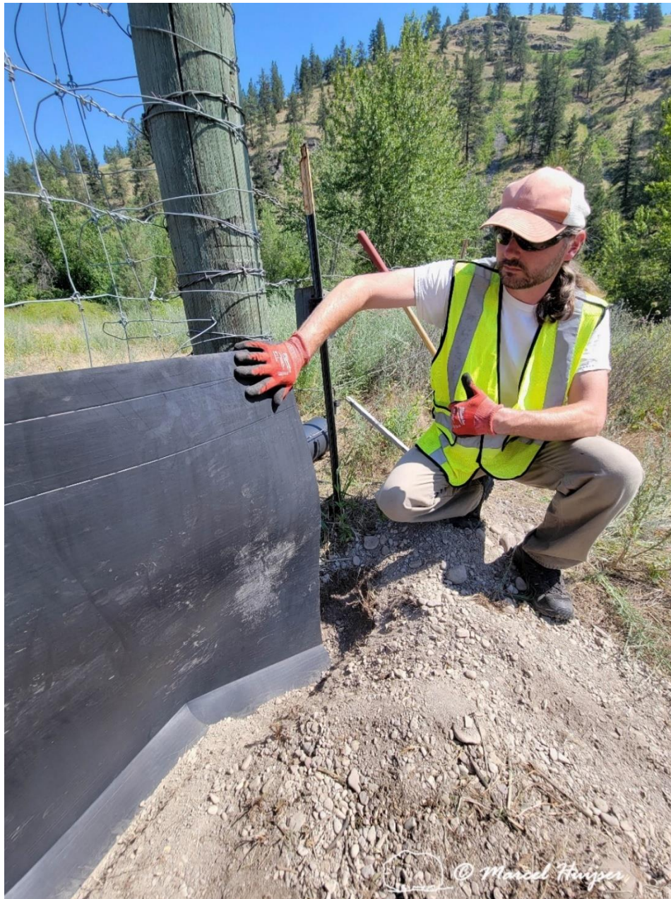
Figure 49. Plastic sheeting during installation for amphibians, reptiles, and small mammals, Montana, USA.
