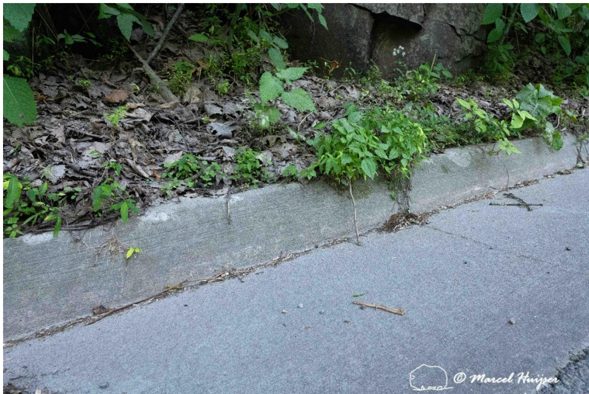
Figure 25: Curb presents a barrier to herpetofauna, Cunard road, New River Gorge National Park and Preserve, Oak Hill, West Virginia.
