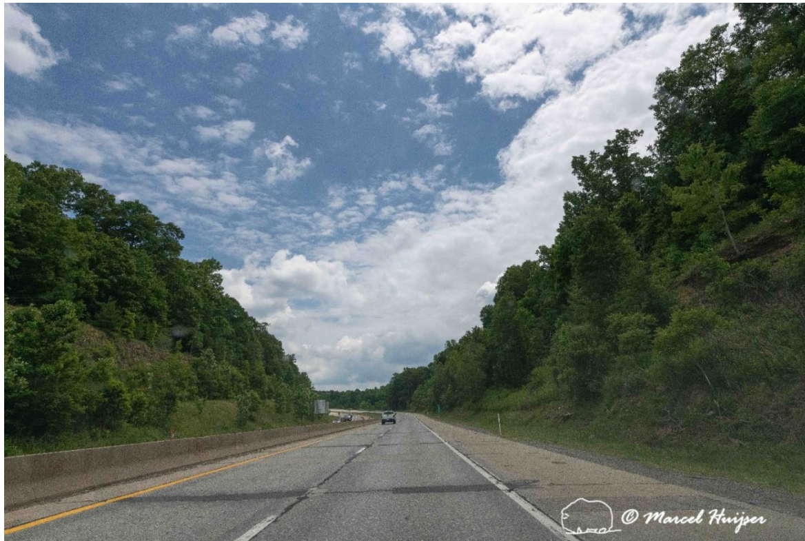
Figure 9: Road cuts through ridges provide an opportunity for wildlife overpasses. I-64 just east of Glade Creek bridge, New River Gorge National Park and Preserve, Shady Spring, West Virginia.
