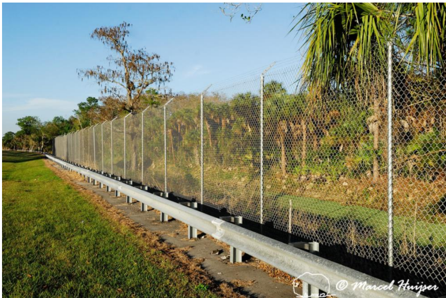
Figure 43. Fence for Florida panther ( Puma concolor coryi ), 10 ft tall, metal posts, chain-link fence material, and overhang, SR 29, Florida, USA).
