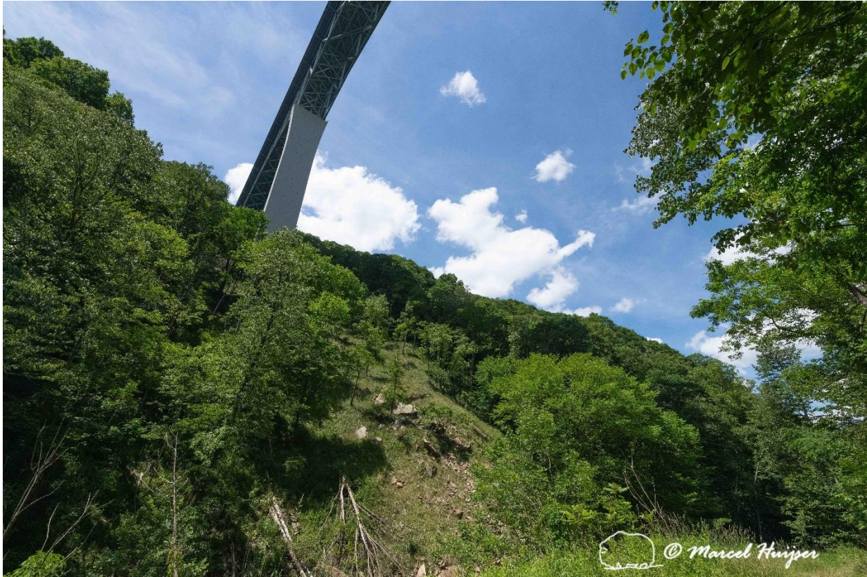
Figure 38: I-64 bridge across Glade Creek, just north of Upper Glade Creek Trail Head, Shady Spring, West Virginia.
