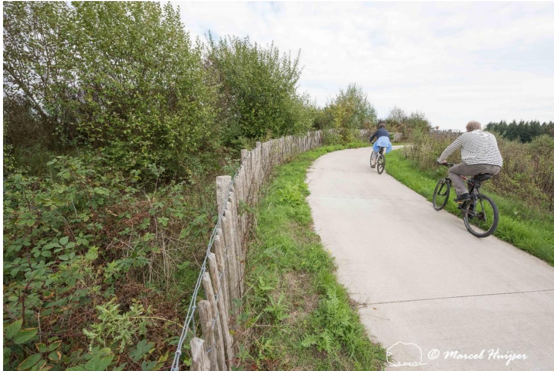
Figure 40. Hiking and biking trail combined with wildlife overpass across railroad tracks Soest The Netherlands. The designated wildlife area is to the left, on the other side of the fence and vegetated berm.
