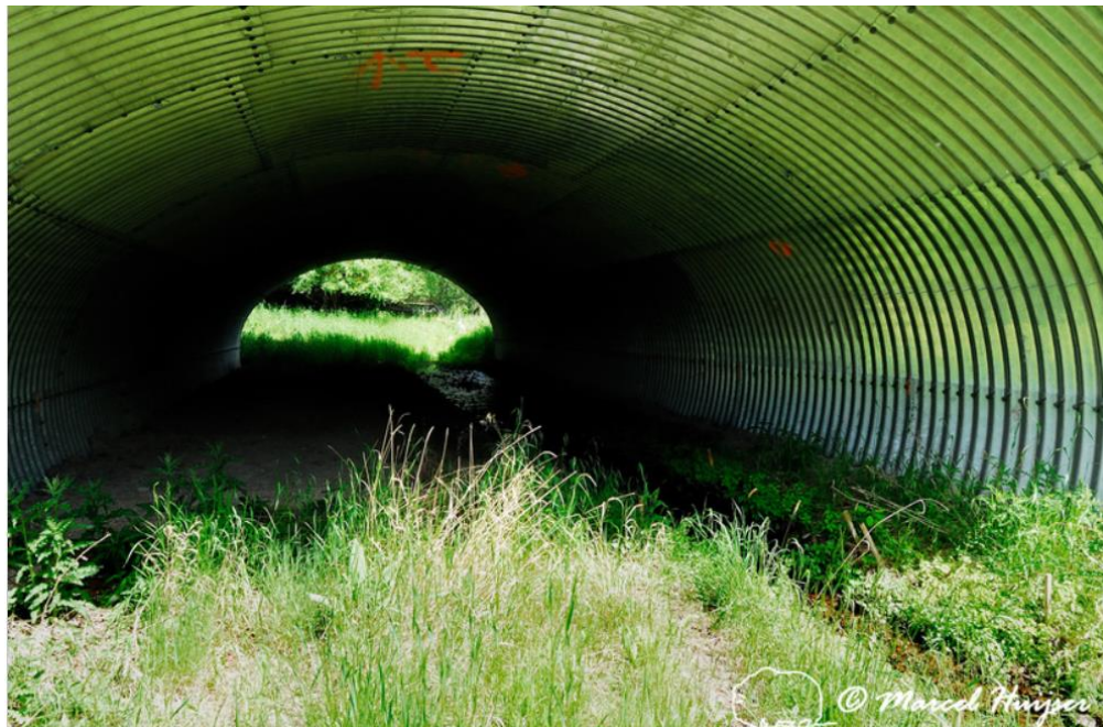
Figure 45. Wildlife underpass (width 7-8 m, height 4-5 m) suitable for white-tailed deer and mule deer and black bear. Not suitable for e.g., elk, pronghorn, grizzly bear.
